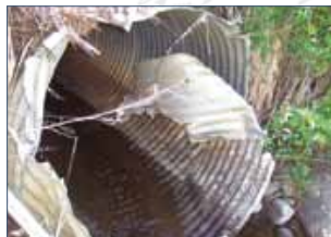
damaged culvert
