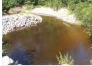
scouring and erosion
