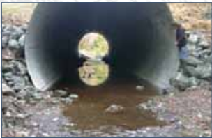
culvert properly embedded into streambed
