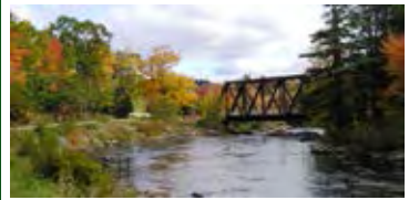
Steel trestle bridge at Cable Pool
