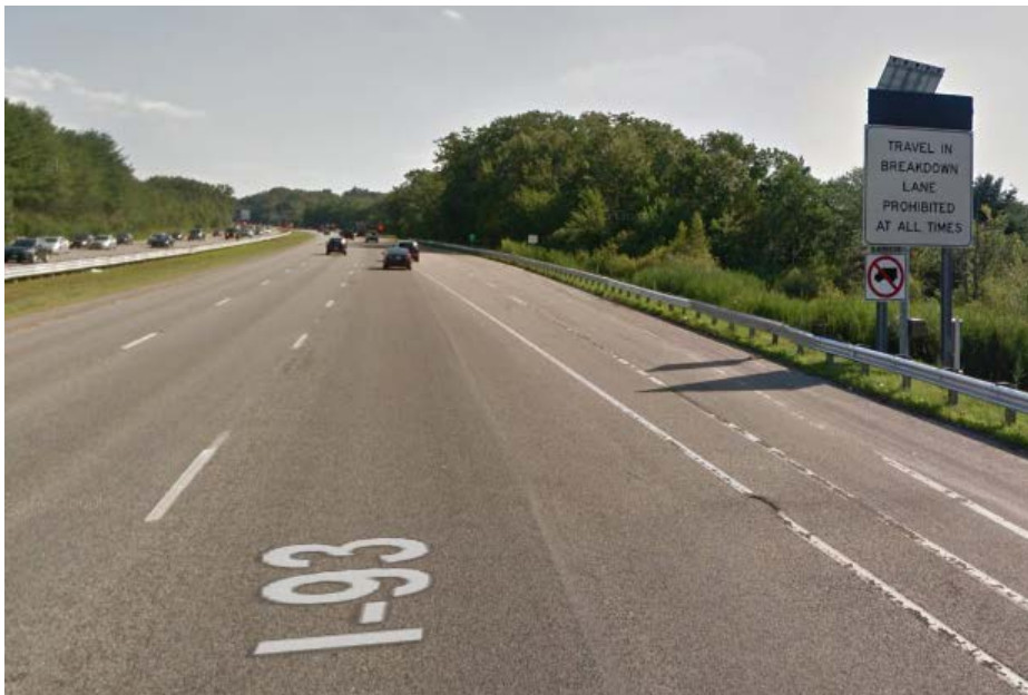
Figure IV-2. Emergency Refuge Area in Methuen, Massachusetts
