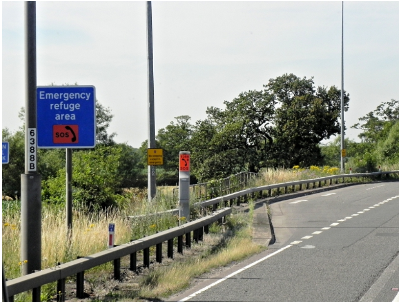
Figure IV-1. Emergency Refuge Area in Great Britain with Emergency Roadside Telephone
