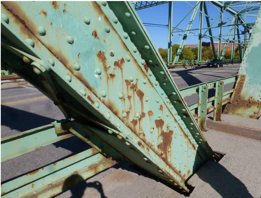
Photo 16: Typical paint condition near travelway
