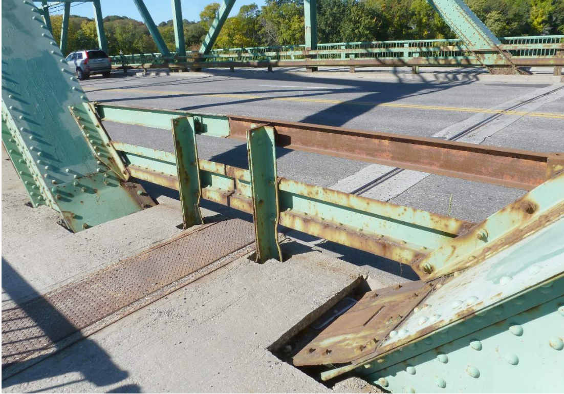
Photo 13: Traffic rail (view over a pier)
