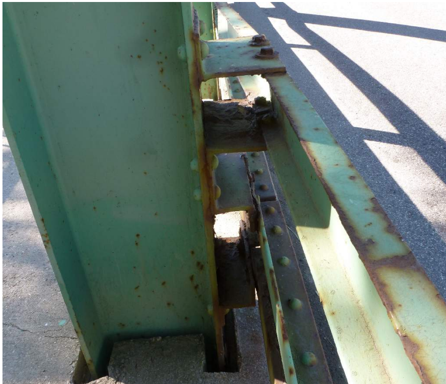
Photo 14: Traffic rail (view at truss vertical)
