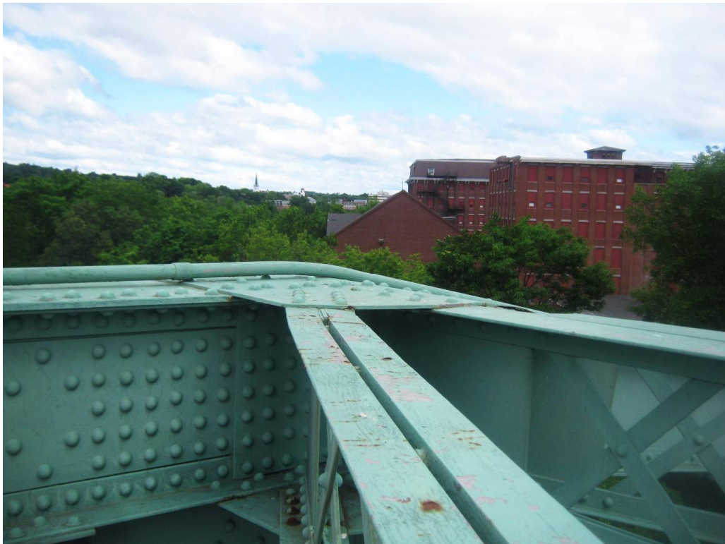
Photo 18: Typical paint condition of truss superstructure
