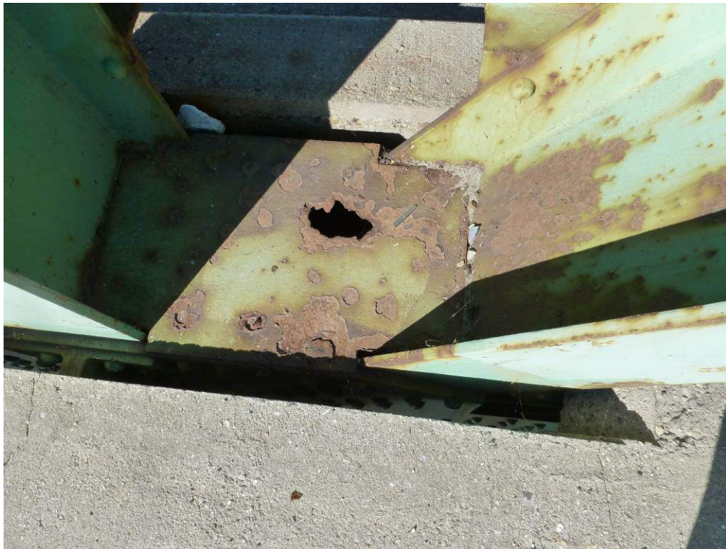
Photo 20: Bottom chord closure plate
