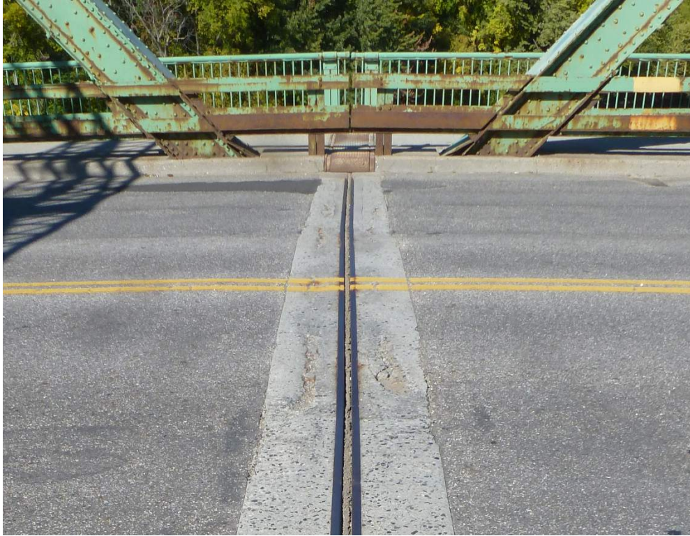
Photo 15: Joint and concrete header (view over a pier)
