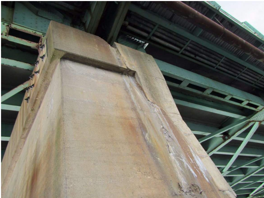
Photo 32: Pier 2 downstream end of pier
