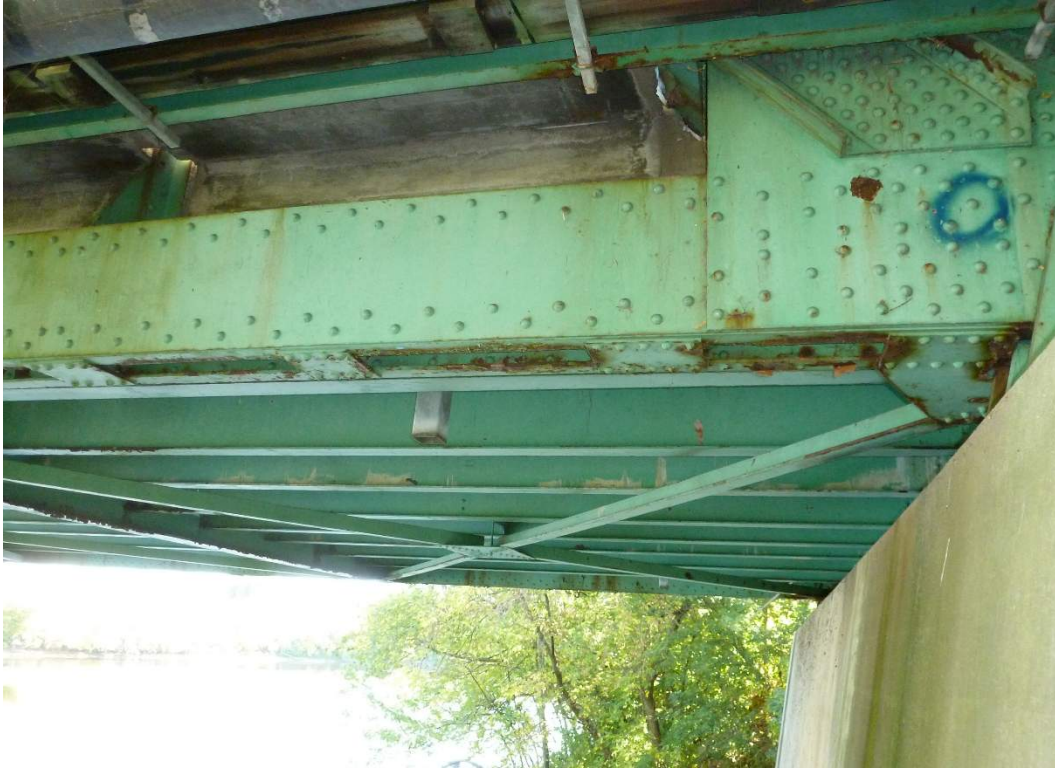
Photo 17: Typical paint condition of floor system
