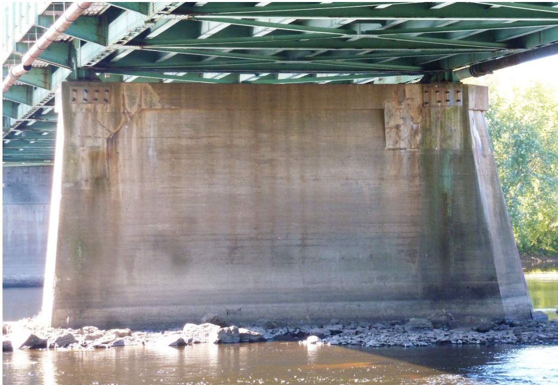
Photo 30: Pier 2 elevation showing 1995 emergency repairs
