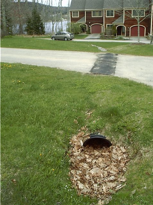
The material was spread throughout this lawn area. During wet weather, water from the lawn is intended to drain through this culvert and into Penobscot Bay.
