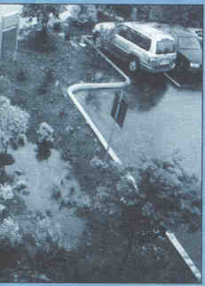
Permeable pavement in parking areas not only allows water to infiltrate the ground but reduces runoff.
