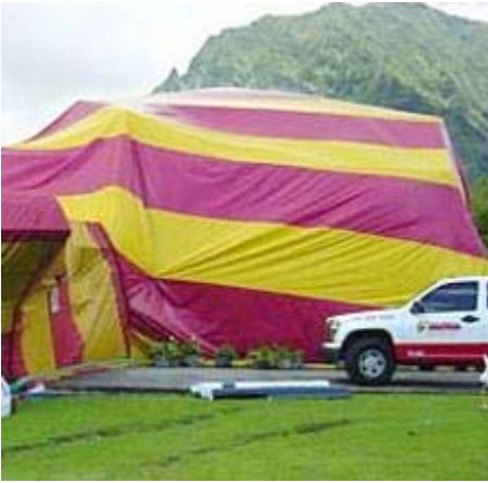
Houses tented for termite treatment with sulfuryl fluoride are a common sight in Honolulu. (Photo courtesy Aloha Termite @ Pest Control )
