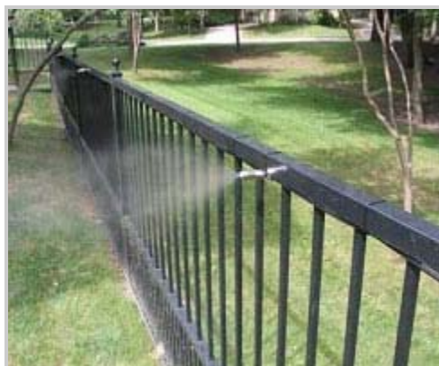
Mosquito Mister installed in fencing, Kansas State Univeristy
