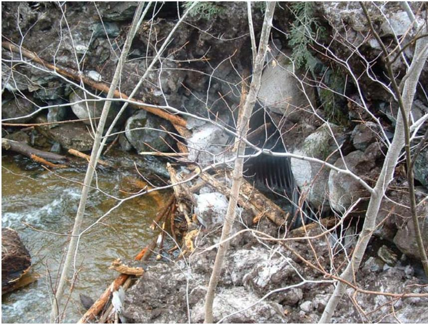
**Figure 42. Route 120 Washout in Andover Caused by Blocked Culvert, Maine April 5, 2005**
