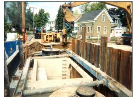
Spring Street Trunk Storm Drain in Saco, Maine
