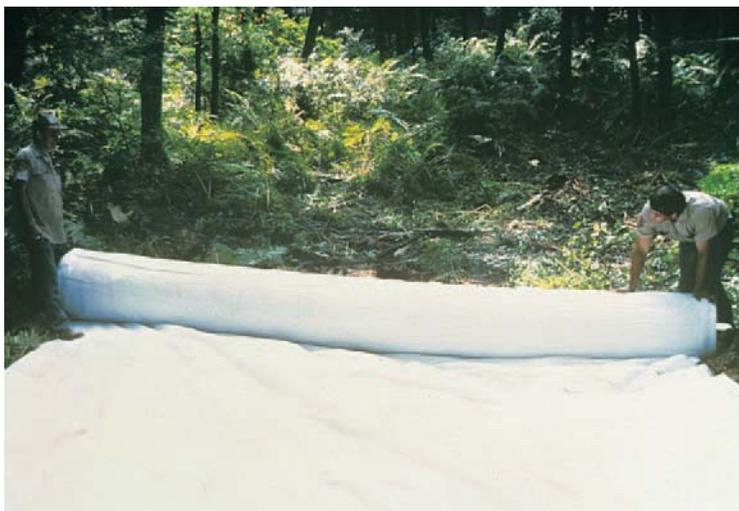
*Use geotextile to keep fill from mixing with the wetland soil.*
