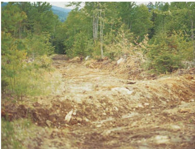
*Water bars move water out of the trail onto the forest floor.*
