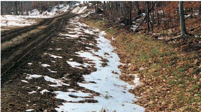
*Revegetated road ditches carry water without eroding.*
