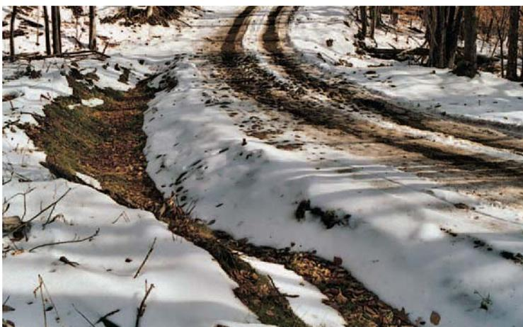
*Properly sized ditches capture and slow down runoff.*
