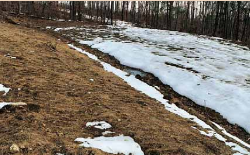
Hay mulch on landing.
