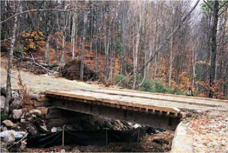
A permanent bridge on a truck road.
