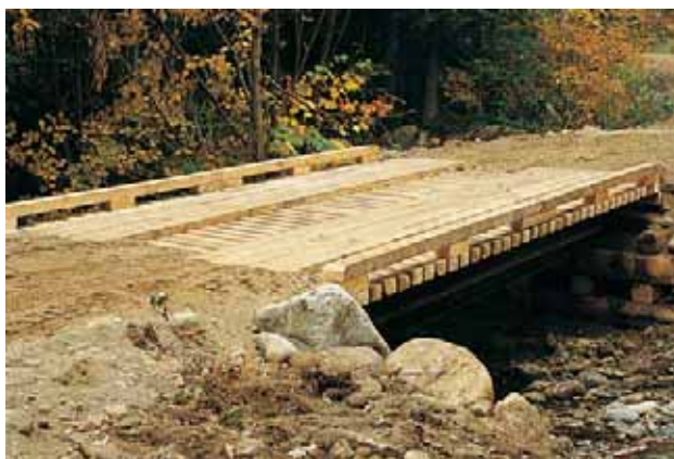
A permanent bridge.
