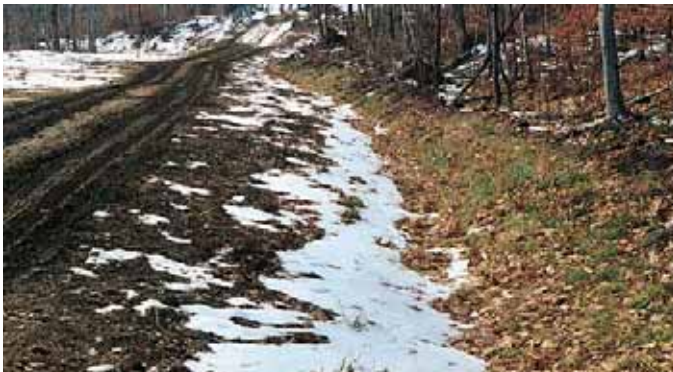
Revegetated road ditches carry water without eroding.
