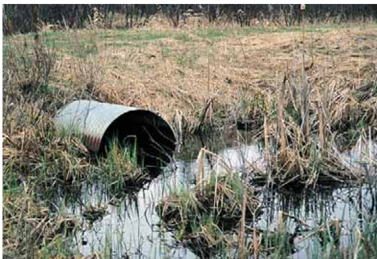
Wetland culverts allow for cross drainage if the road fill does not.
