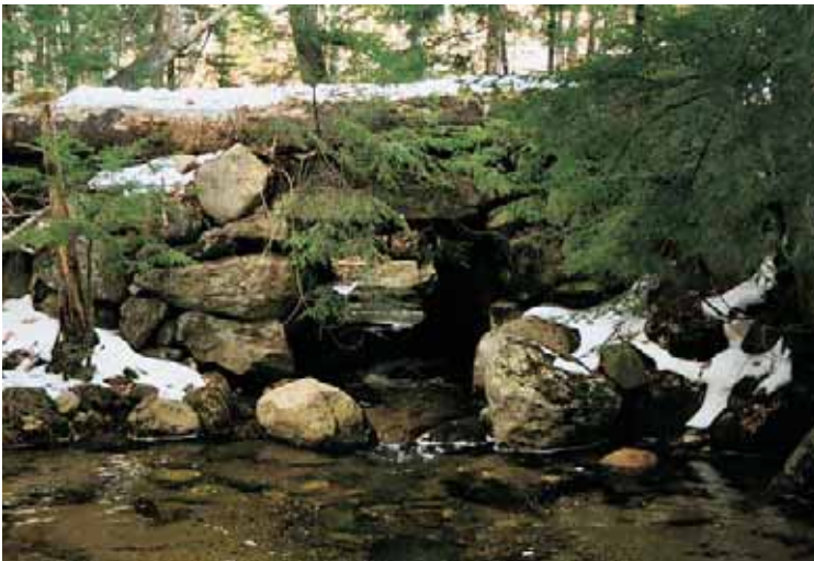
An old stone culvert still functioning.
