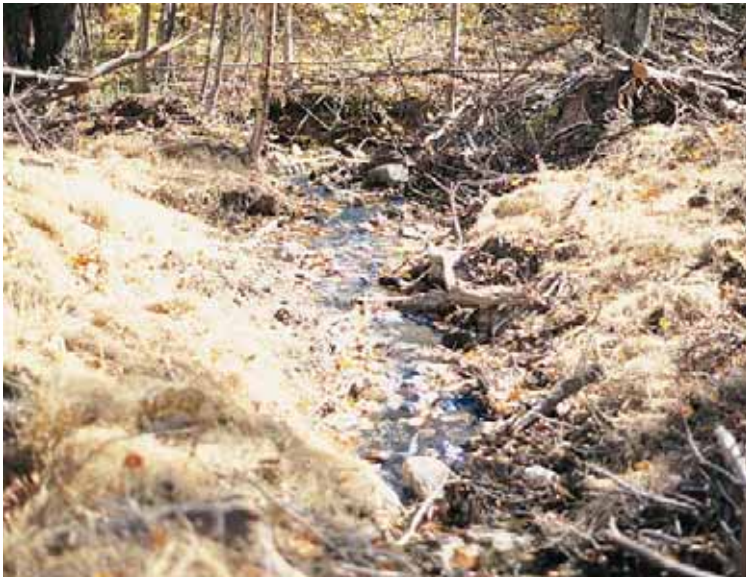
Closeout of a temporary stream crossing.
