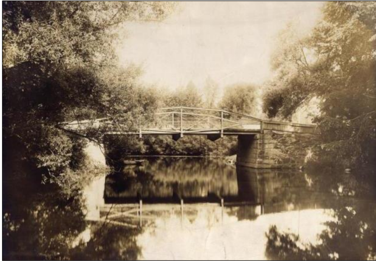
Figure 7: Former Presumpscot River Bridge
