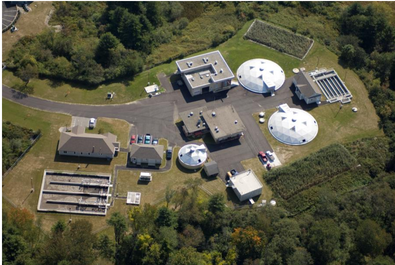
Figure 9: Richard B. Goodenow Wastewater Treatment Facility
