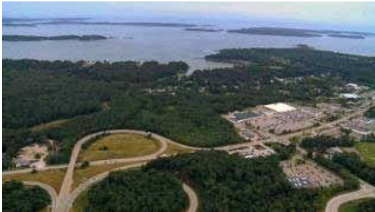
Figure 4: Aerial view of Route One, Falmouth Foreside and Casco Bay
