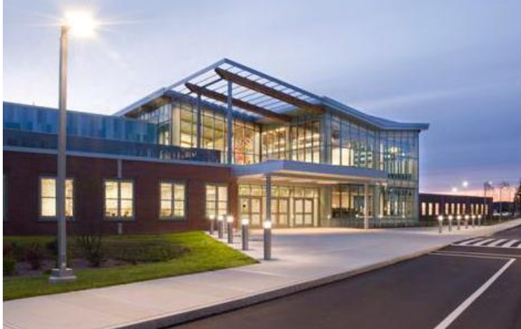
Figure 2: Falmouth Elementary School
