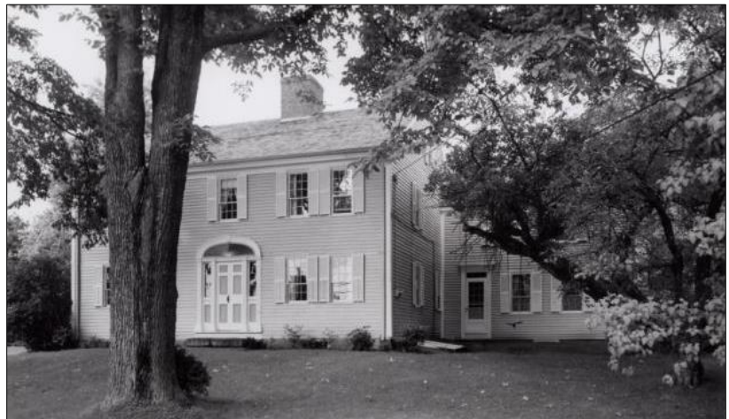
Figure 17: James Merrill House, Falmouth Road, reportedly built about 1738
