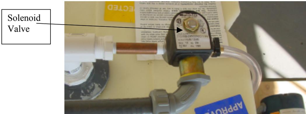
Figure 3: Normally closed solenoid valve
