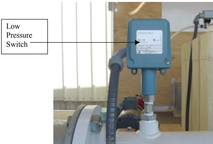
Figure 4: Pressure switch
