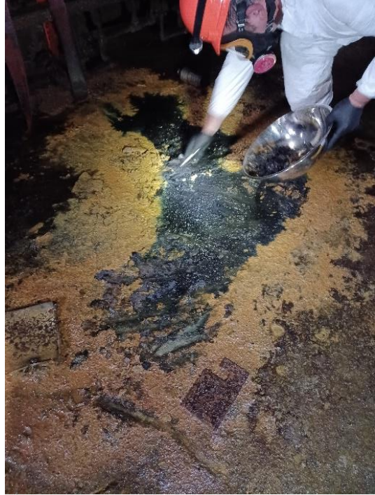
Photo 35: Floor Solids Sample Being Collected in Units 1 & 2
