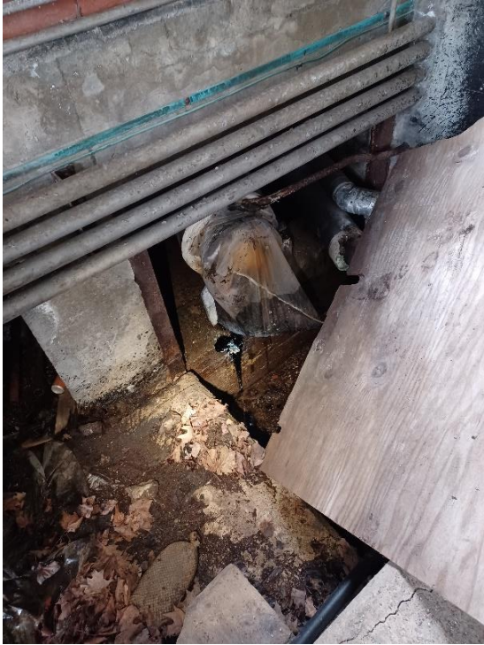
Photo 31: #6 Oil Release in Screenhouse #2
