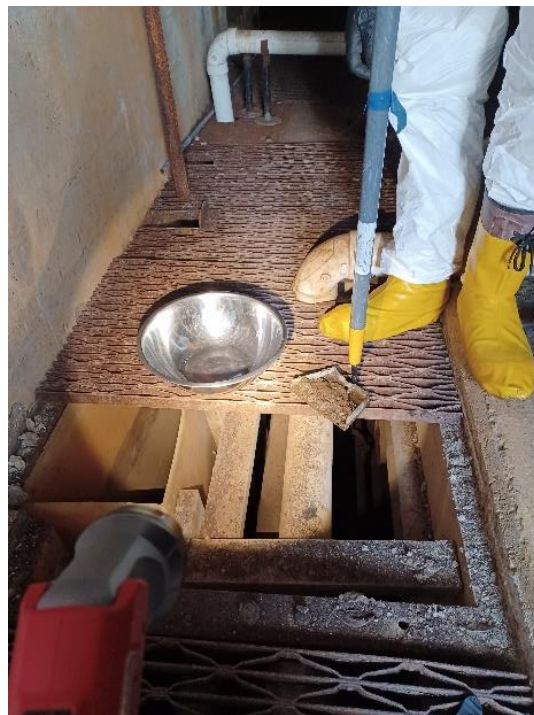
Photo 19: Collecting SD-418 from Units 1 & 2 Floor Trench
