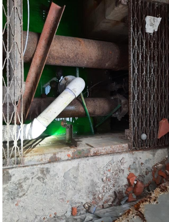
Photo 14: EF-05 Floor Trench After Tracer Dye Application
