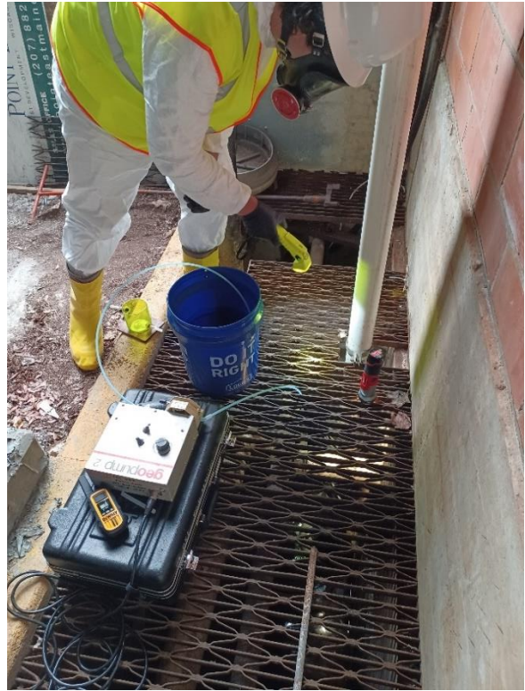
Photo 18: Adding dye to floor trench at EF-04 Units 1 & 2
