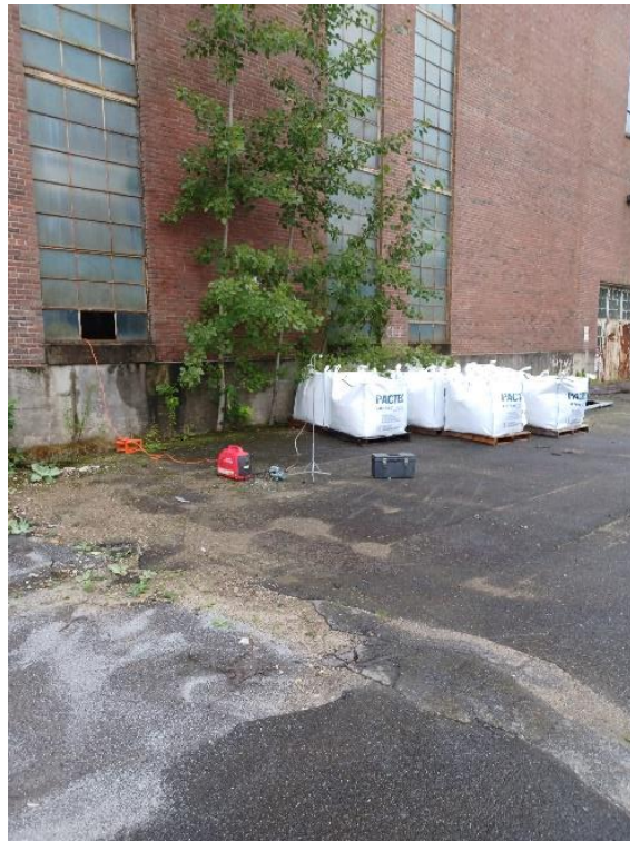
Photo 36: BE-A-04 Being Collected. Sacks of PCB Concrete in Background
