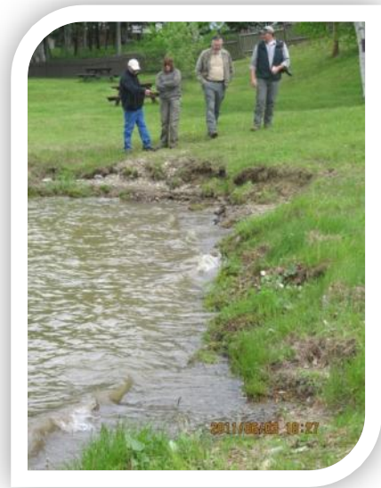
Sample 319 grant project: eroding lake shoreline before BMP implementation.
