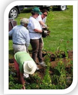
Local BMP implementation - planting a rain garden.
