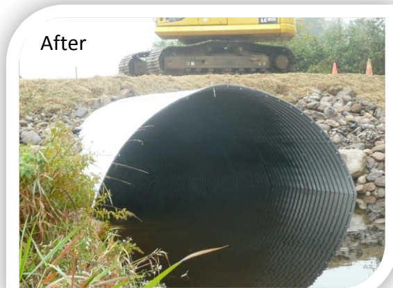
Sample 319 grant project: Undersized round culvert replaced with a much larger arch culvert; road no longer washes out during storm events.
