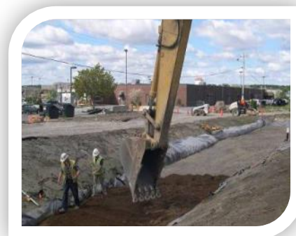
Watershed-based plan implementation - installation of bioretention swale.
