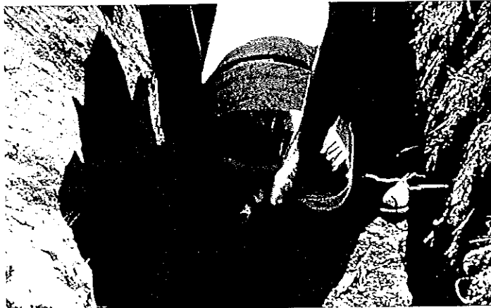
At the end of each line, place an ADS end cap and pull the Drain Guard over.
