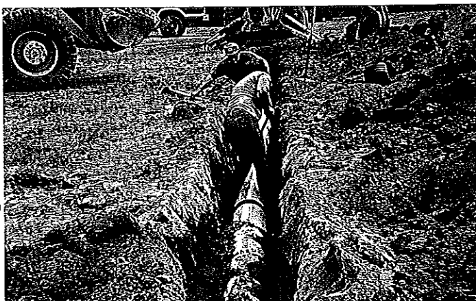
At the end of each line, place an ADS end cap and pull the Drain Guard over.
