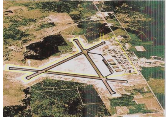
Figure 9. Pennfield NB solar drying site.
