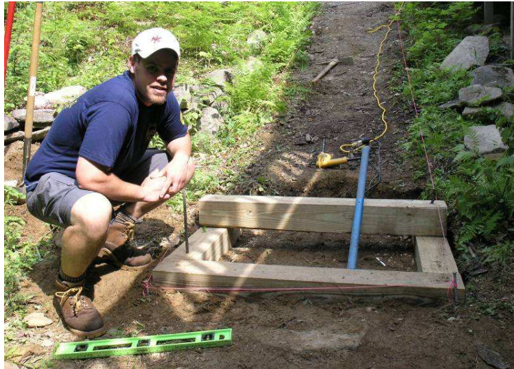
Freeman working on an infiltration steps project
