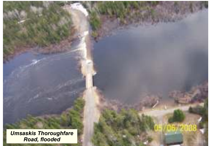
Lock Dam, flood stage
