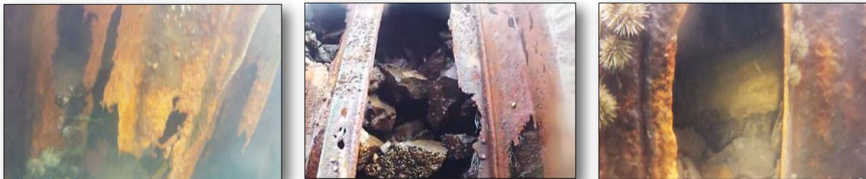
The steel sheet piles contain severe deterioration both above and below the water line. Note large holes in the steel sheet pile and significant loss of fill from behind the steel sheet piles.
