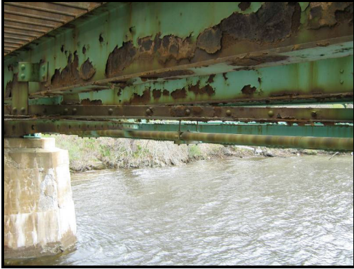
Paint System Failure and Resulting Steel Corrosion
