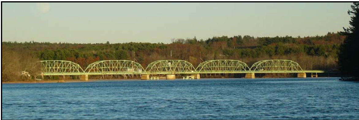
Center Bearing Swing Truss Span with Two Fixed Truss Spans on Each Side
