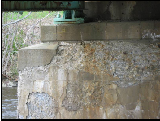
Substructure Deterioration.
