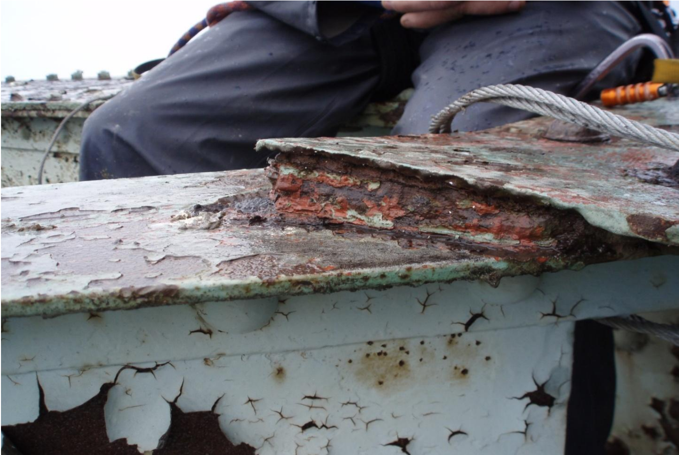
U1 Lateral bracing on top chord, typical example of 1" pack rust between gusset plate and framing members
