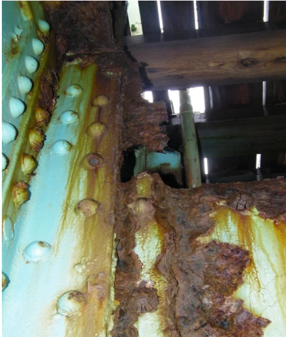
Span 3 Gusset Plate L9 East Interior face of bottom chord with severe deterioration
