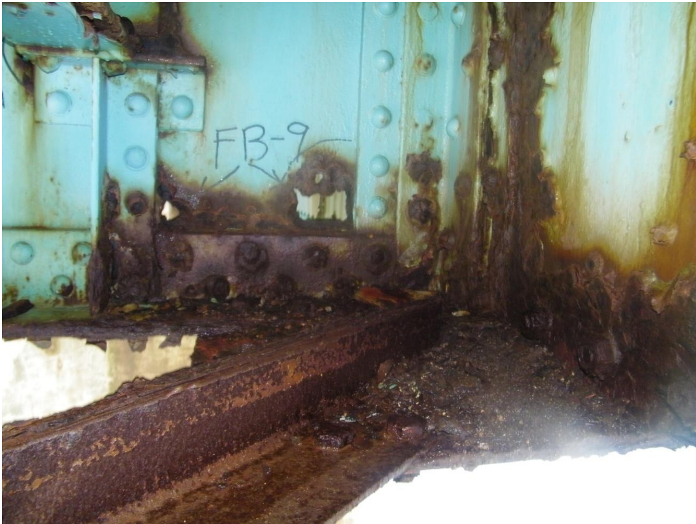
Span 3 Floorbeam 9, South Face, East End Heavily deteriorated with holes in web of roadway floor beam Roadway Floorbeam has been previously repaired as evidenced by bolts.
