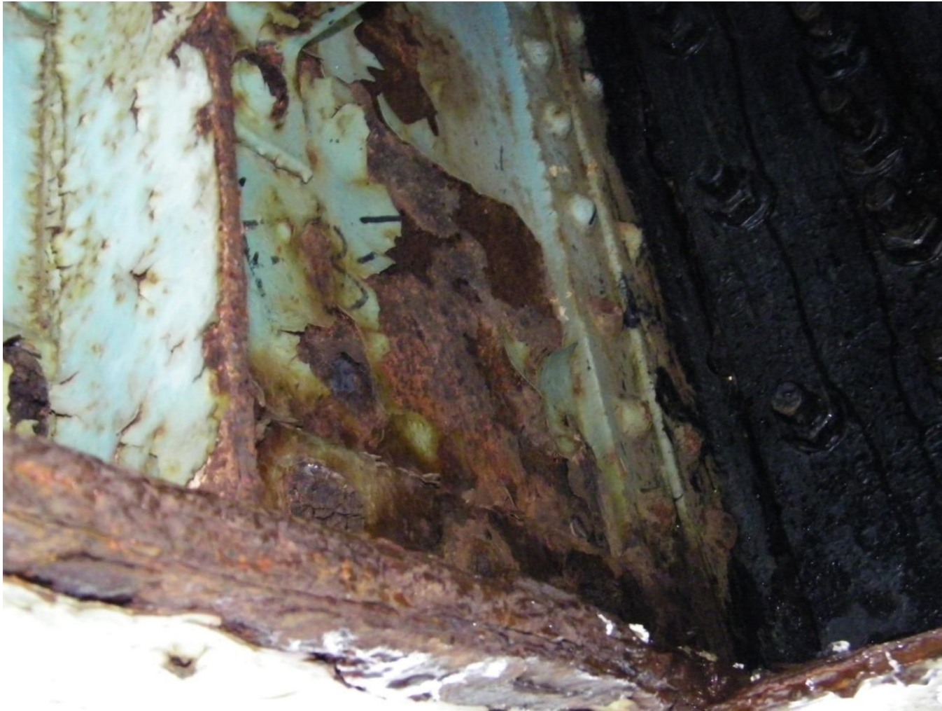
Span 1, Floorbeam 6, North Face Typical condition in roadway floor beams near chords
