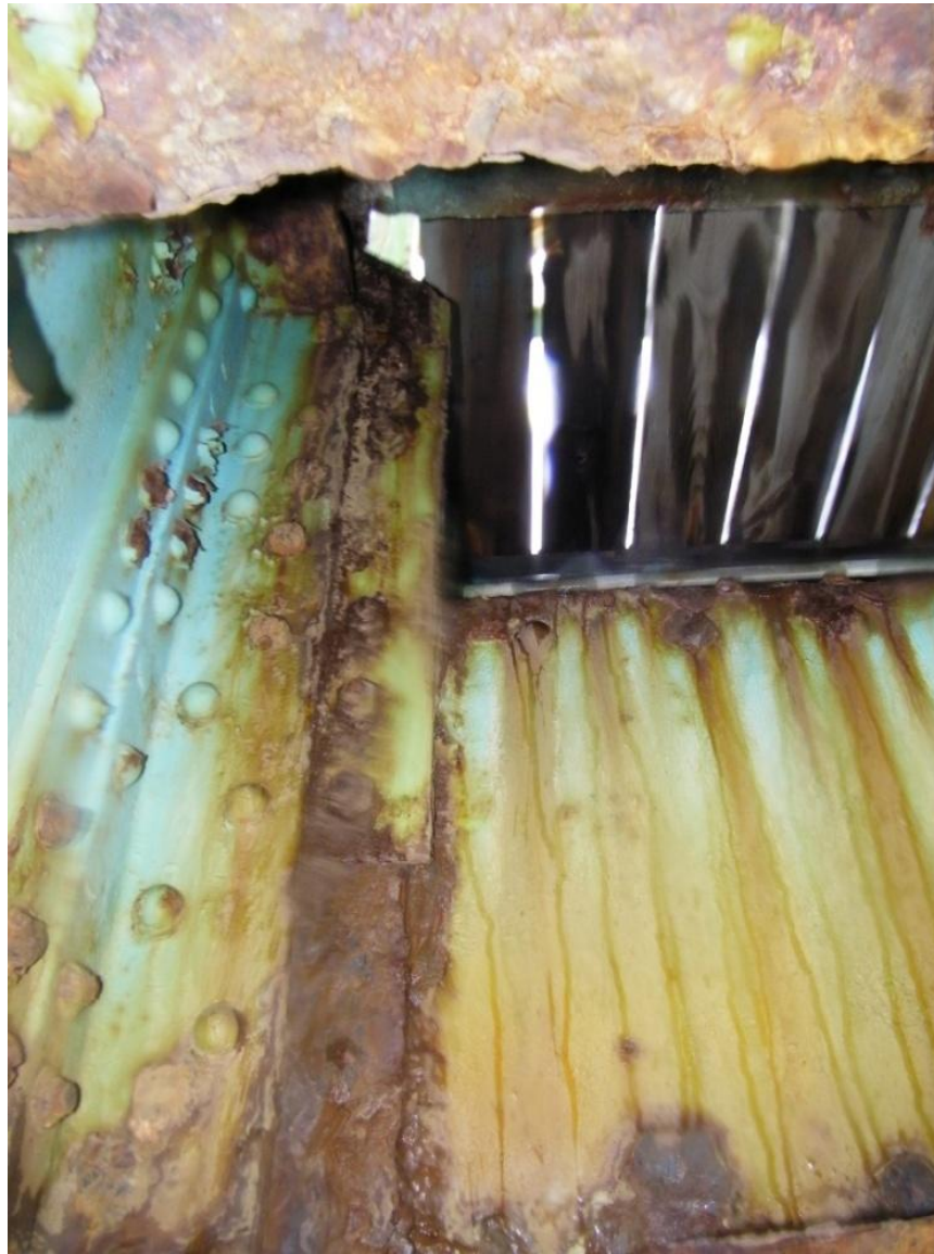
Span 1 Gusset Plate L9 East with repair, plate from previous repair Roadway floor beam (left) framing into interior face of bottom truss chord (right)
