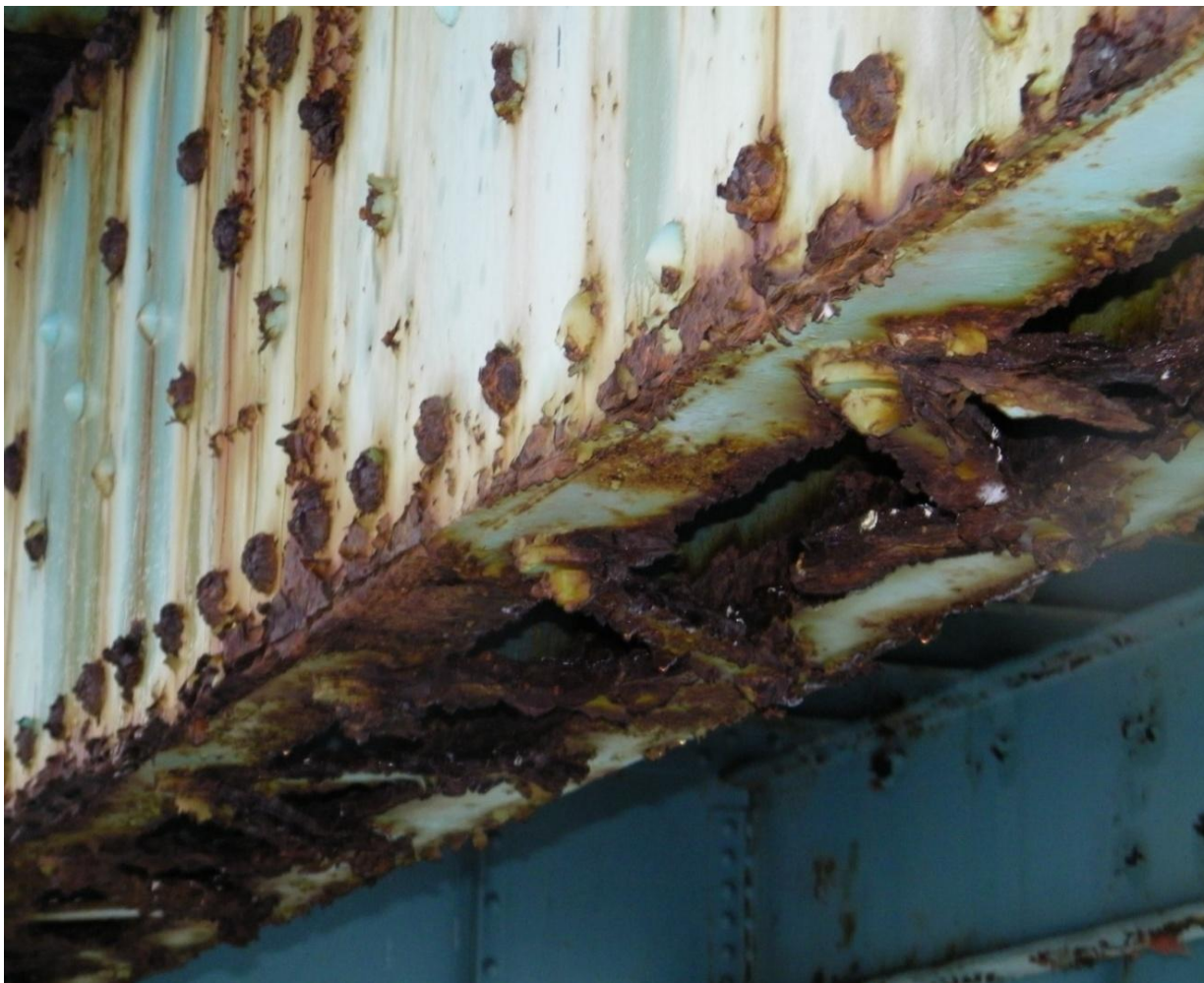
Span 3 Bottom Chord L3-L4, West Exterior Face Typical Lacing and rivet head Deterioration
