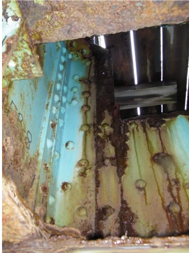
Span 1 Gusset Plate L7 East Roadway floorbeam/bottom truss chord connection - wooden sidewalk walking surface above
