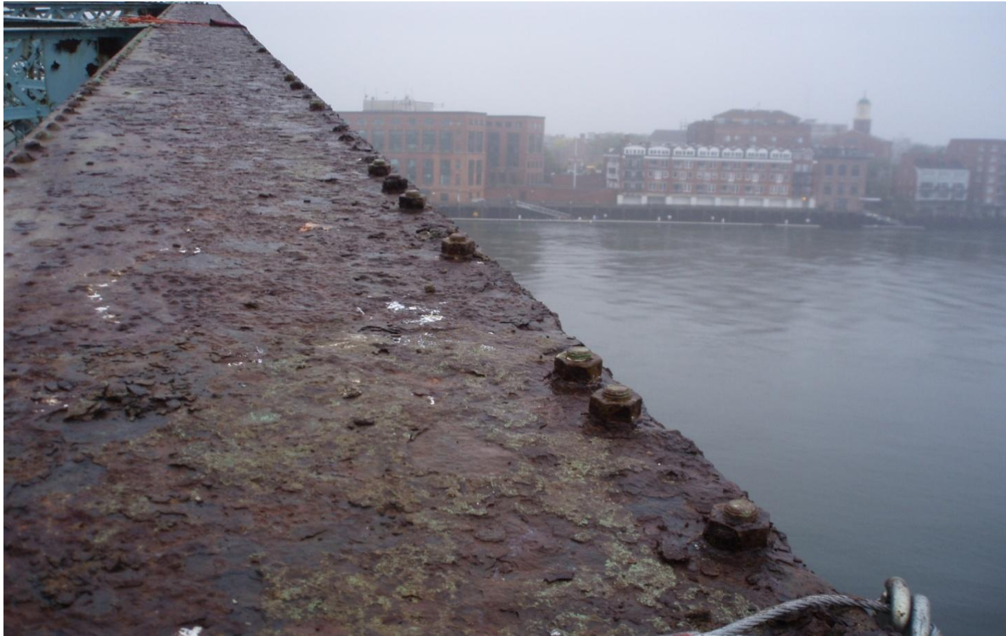
Top chord looking south from U2 looking towards Portsmouth. Rivets replaced by bolts in previous repair. Gaps between bolts suggest severely deteriorated rivet heads
