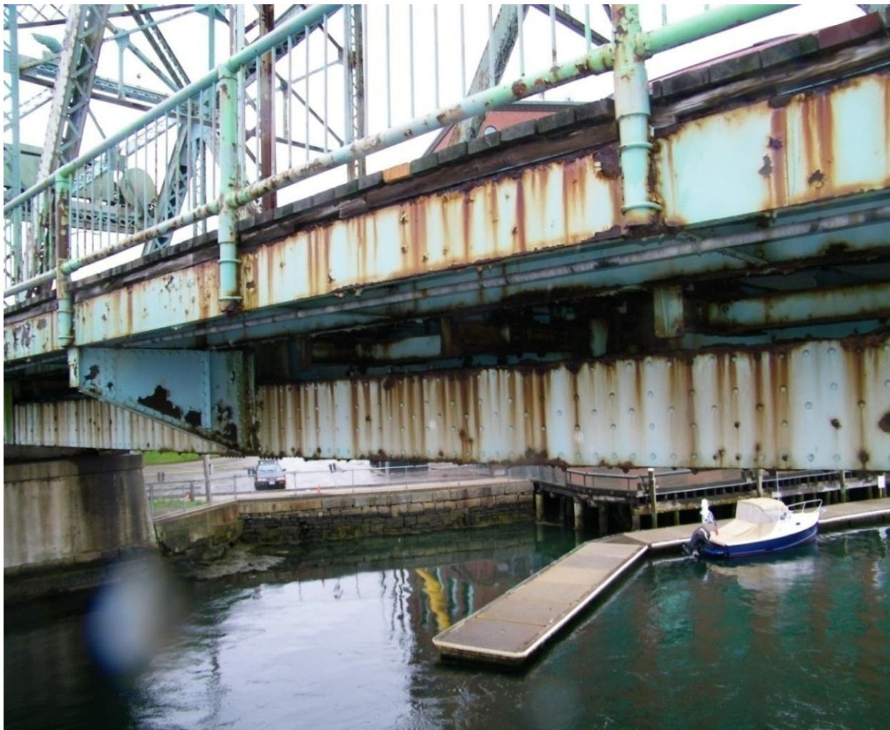
Span 1 Bottom Chord L2-L3, East Exterior Face Typical Fixed Span Bottom Chord Condition between truss panel points
