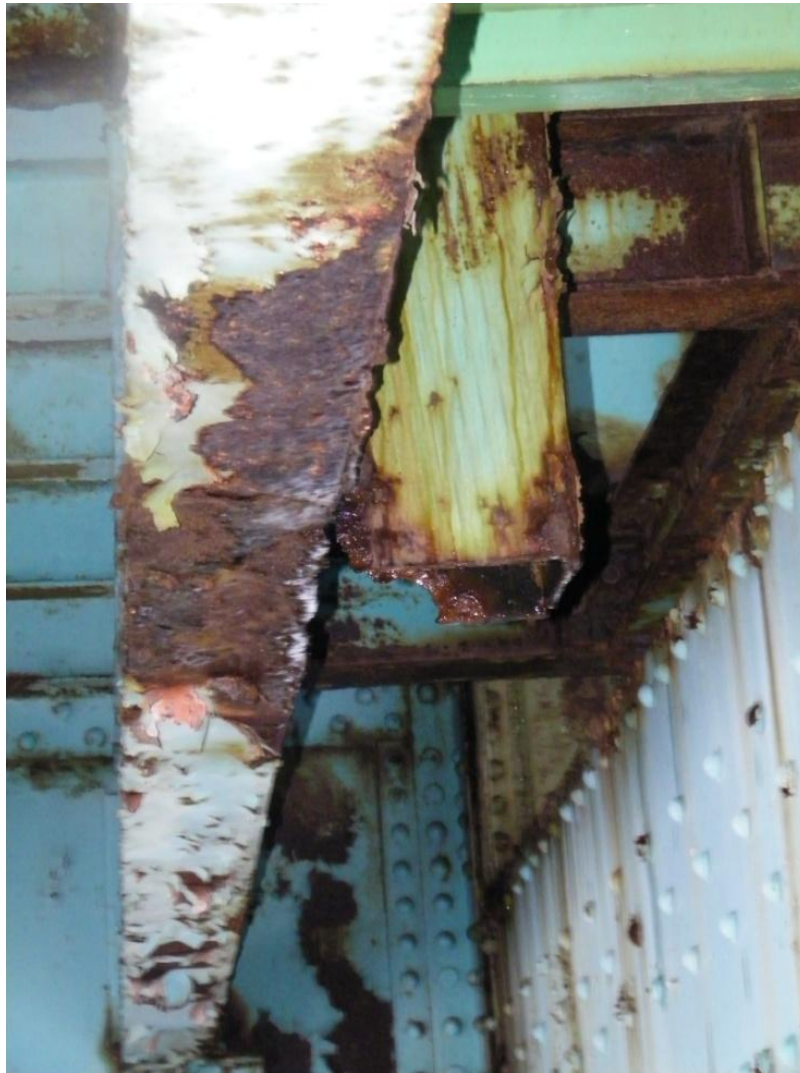
Span 1, Bay 8, Stringer 7 (East Roadway Stringer) Typical stringer condition at metal drain pipe
