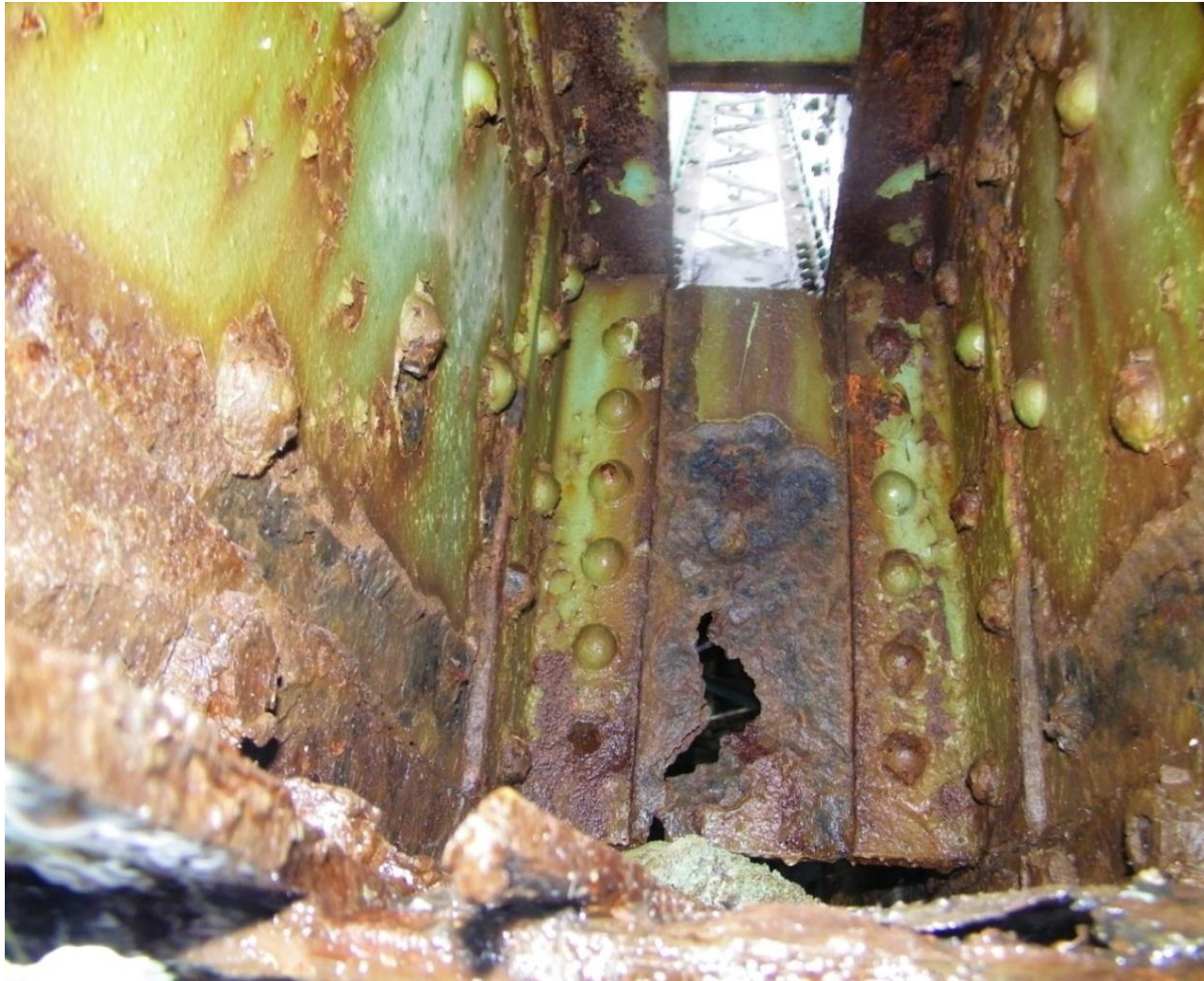
Inside of Chord at Gusset L9 in Span 3. Deteriorated lacing in the foreground and a deteriorated internal stiffener plate center. Truss diagonal seen just above internal stiffener plate
