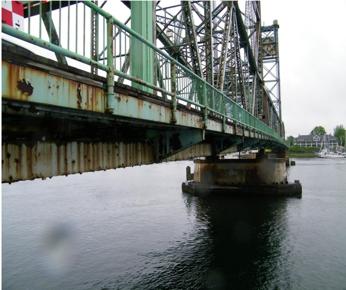
Span 1 Bottom Chord L4-L5, East Exterior Face Typical Fixed Span Bottom Chord Condition between truss panel points
