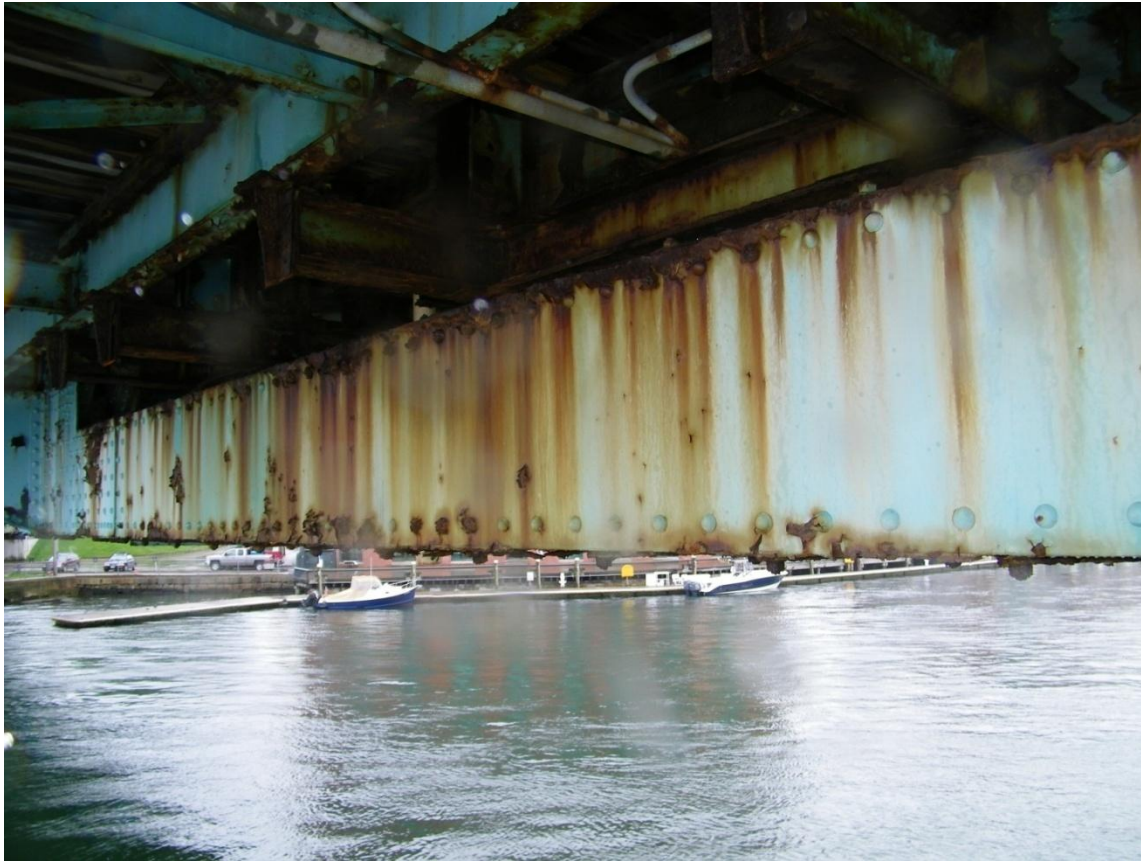
Span 1 Bottom Chord L8-L9, East Exterior Face Typical Condition at Fixed Span Bottom Chords between panel points
