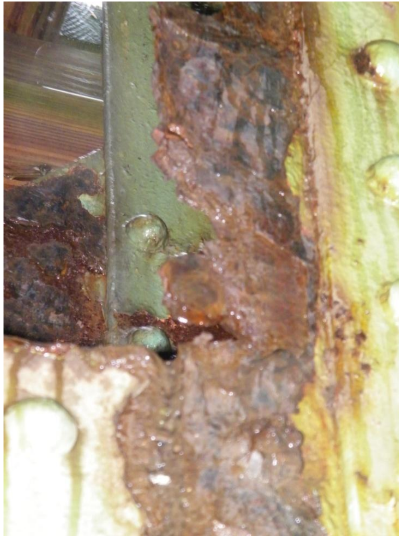
Span 3 Gusset Plate L3 East Interior with severe section loss Roadway beam (right) framing to the bottom truss chord (lower left)
