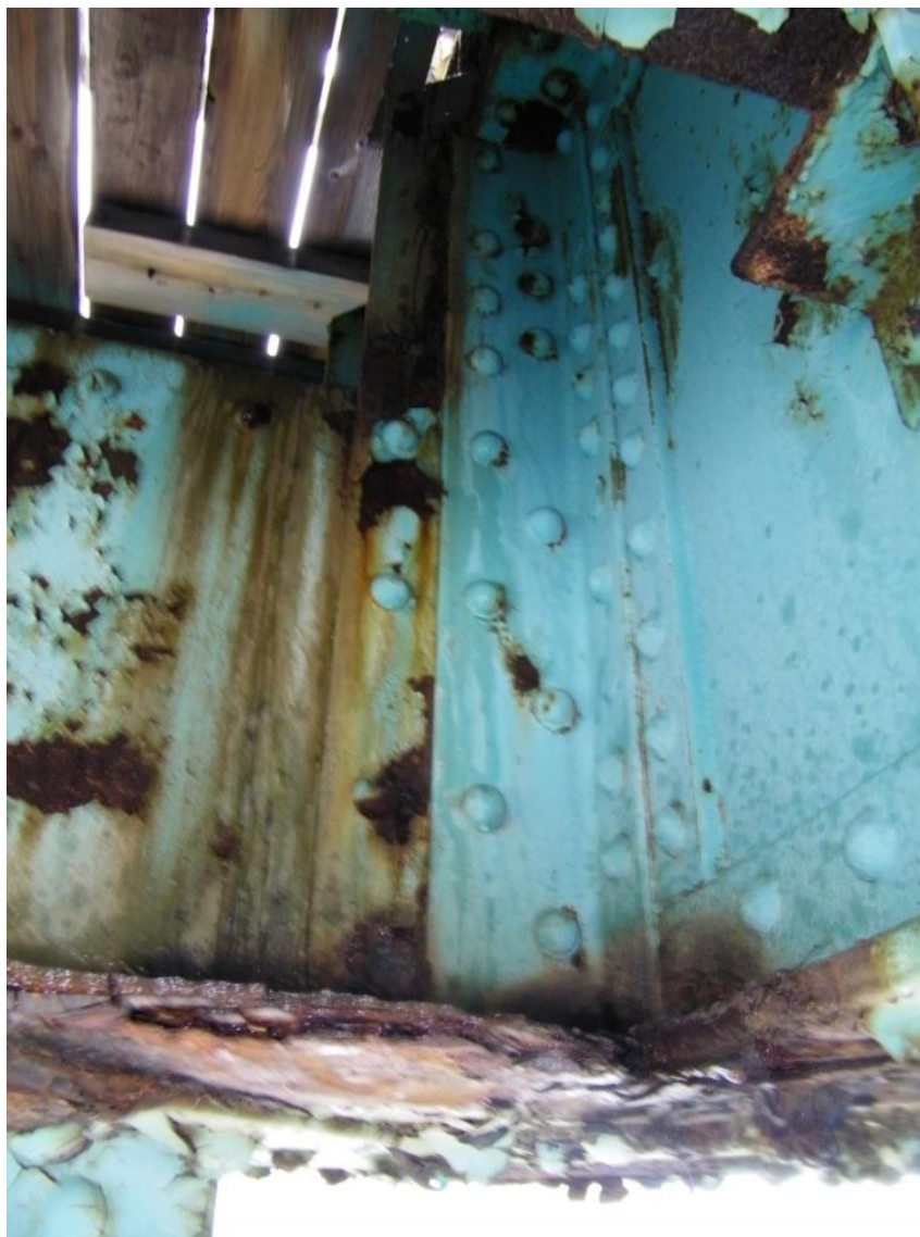
Span 1 Gusset Plate L7 East horizontal gusset plate between roadway floor beam and the fixed span truss bottom chord.
