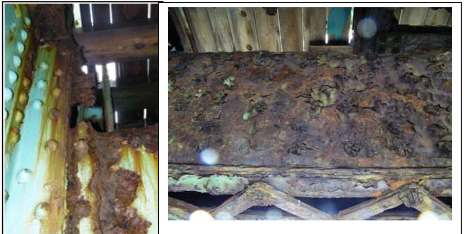
Corrosion of Steel Members on lift span
