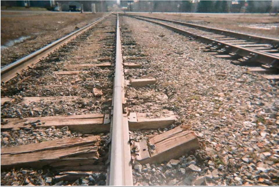
Figure I-4 Example of center bound track condition
