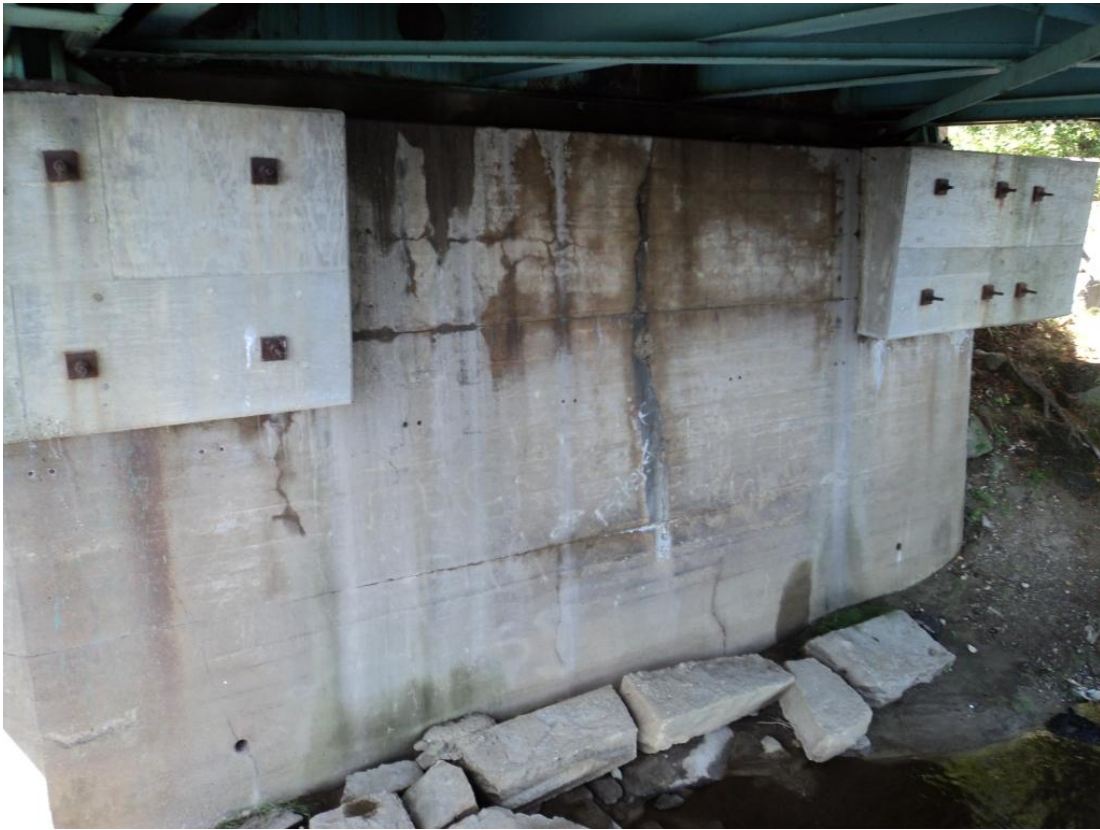
Photo 67 – Both abutments have been retrofitted with Dywidag post-tensioned concrete encasement repairs immediately below both truss bearings. View at south abutment. Also note wide vertical crack in breastwall at centerline of bridge and two lower cracks.
