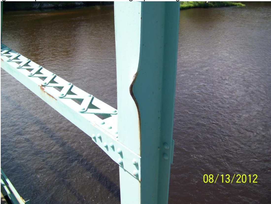
Photo 46 – At L2 in the Span 2 roadway truss the vertical U2-L2 has sustained impact damage and a permanent bend in the flange tip of 1 ½ inches over a length of two feet.
