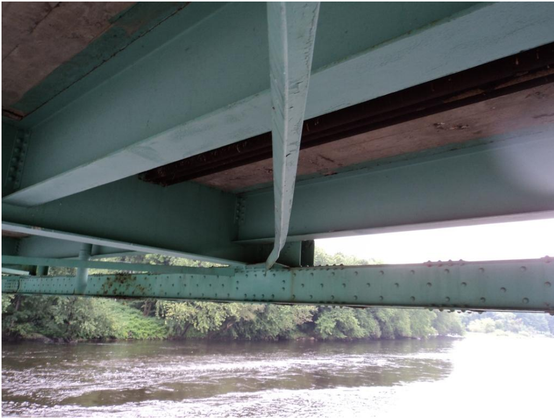
Photo 59 – The lower lateral bracing angle in Span 2 connecting FB4 sidewalk truss and FB5 roadway truss is displaced laterally in the horizontal plane by 6 inches.
