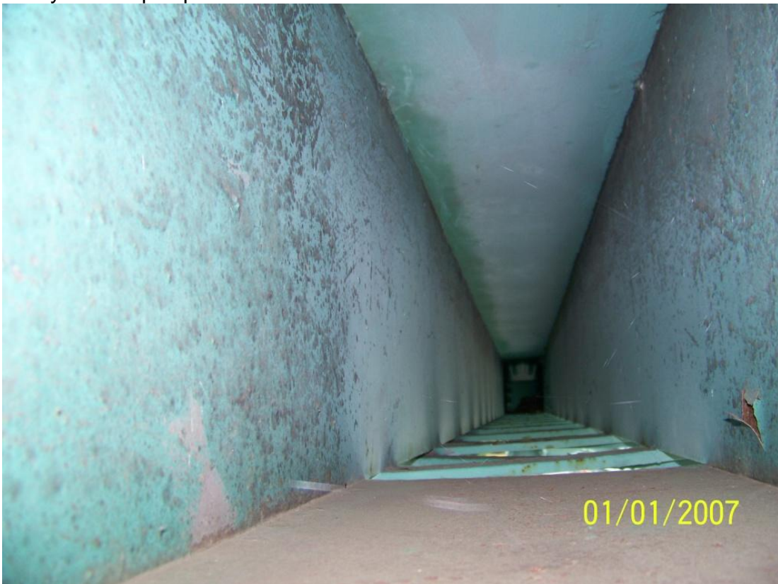
Photo 30 – Paint system is generally intact with minimal failures throughout exterior and interior surfaces of upper chords. View inside Span 3 sidewalk truss U3-U4.
