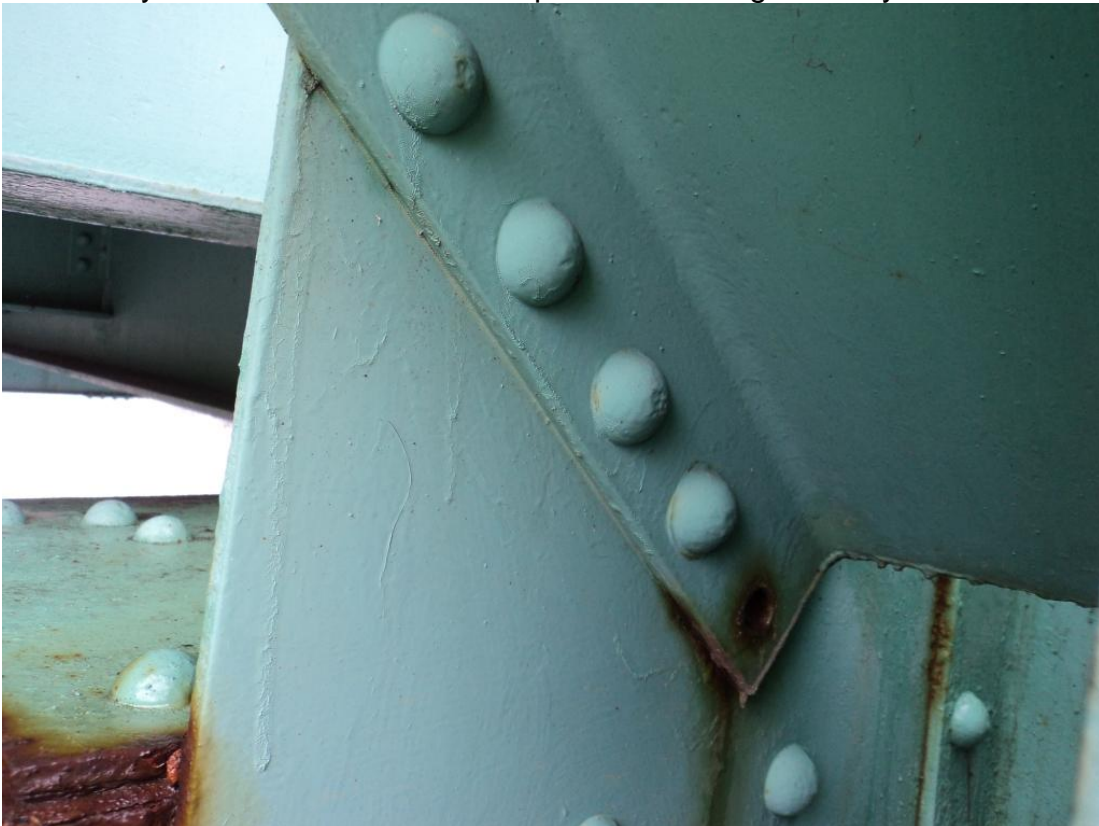
Photo 48 – The Span 2 roadway truss diagonal U1-L2 is missing a single rivet in the east face L2 gusset, leaving 19 of the original total of 20 rivets to resist the member loads.
