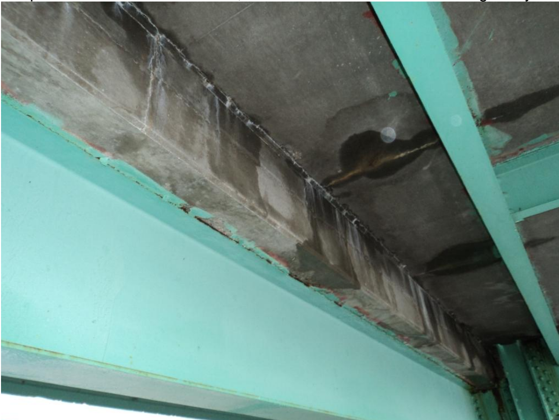
Photo 12 – In Span 2 between FB1 and FB2 two cracks with efflorescence in sidewalk slab and a longitudinal crack with efflor. along sidewalk horizontal construction joint .
