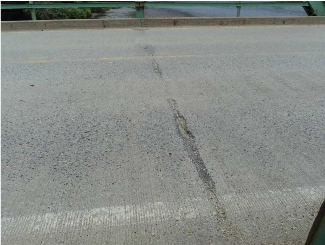
Photo 7 – Above FB1 in Span 3 the transverse construction joint has three small spalls patched with bituminous material.
