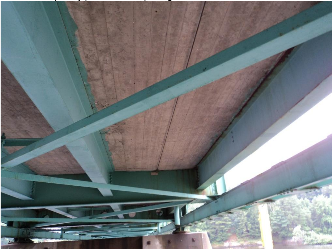
Photo 78 – Between S5 and S6 in Span 1 there is an abandoned former messenger cable which extends over portions of the bridge length. Looking south.
