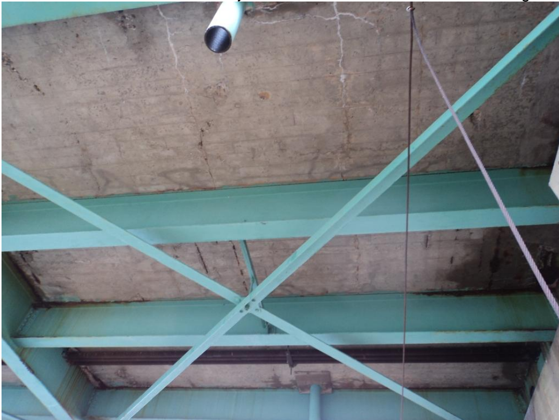
Photo 14 – In Span 2 between FB7 and FB8 four transverse cracks with efflorescence were noted between S5 and S6 in top portion of photo. Looking east.
