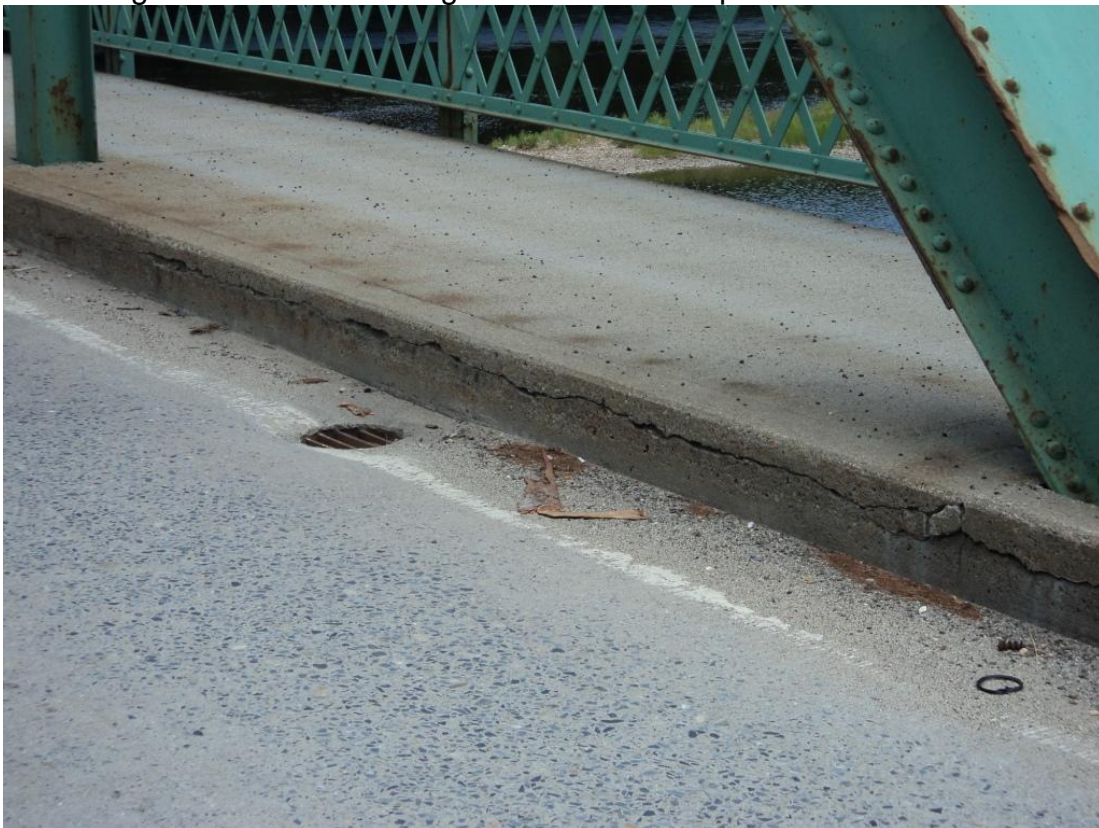
Photo 24 – East sidewalk curb face has a wide horizontal crack at south end of Span 3 which extends along mid-height of curb for nearly half of the length of the span.
