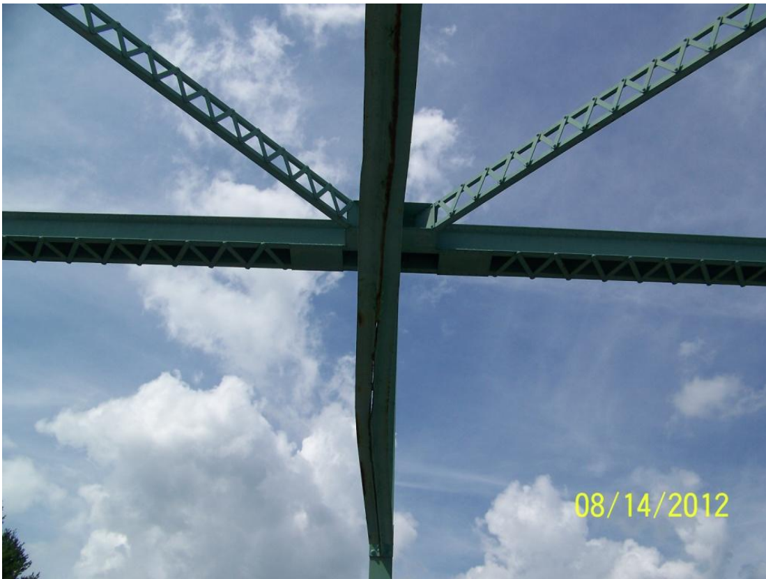
Photo 55 – Impact damage to Span 3 U4 sway frame lower transverse member along with twisting and local vertical bends in edges of horizontal legs of angles over both lanes.
