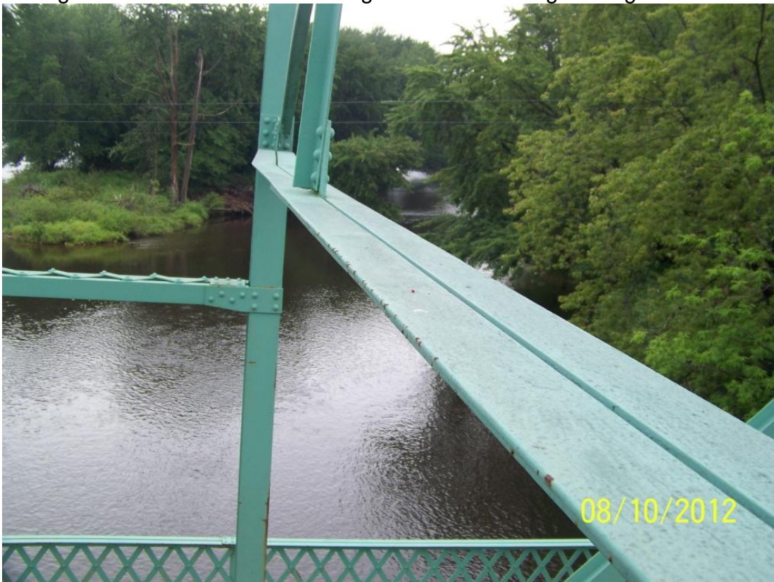
Photo 56 – Impact damage to the sway frame lower transverse member along with lateral displacement in the horizontal plane of more than 3 inches was observed at Span 3 U6.
