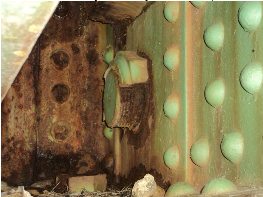
Photo 66 – The bearing pin nut on the east side of the roadway truss bearing is cracked and the lower half of the nut has fallen away completely from the face of the chord.
