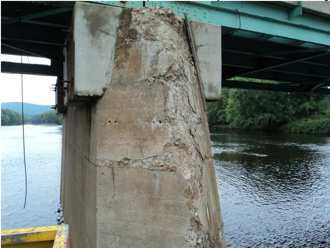
Photo 72 – The west end of Pier 2 has a zone of spalls and scaling along the full height of the icebreaker edge. Looking east in the downstream direction at upstream end of pier.
