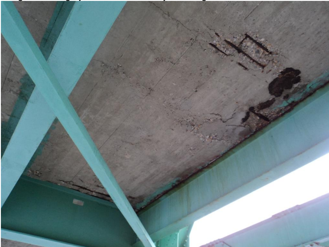
Photo 18 –In Span 2 between S5 and S6 two spalls with exposed reinforcing measuring approximately 2 feet square each, near mid-panel and at FB3. View is looking south.
