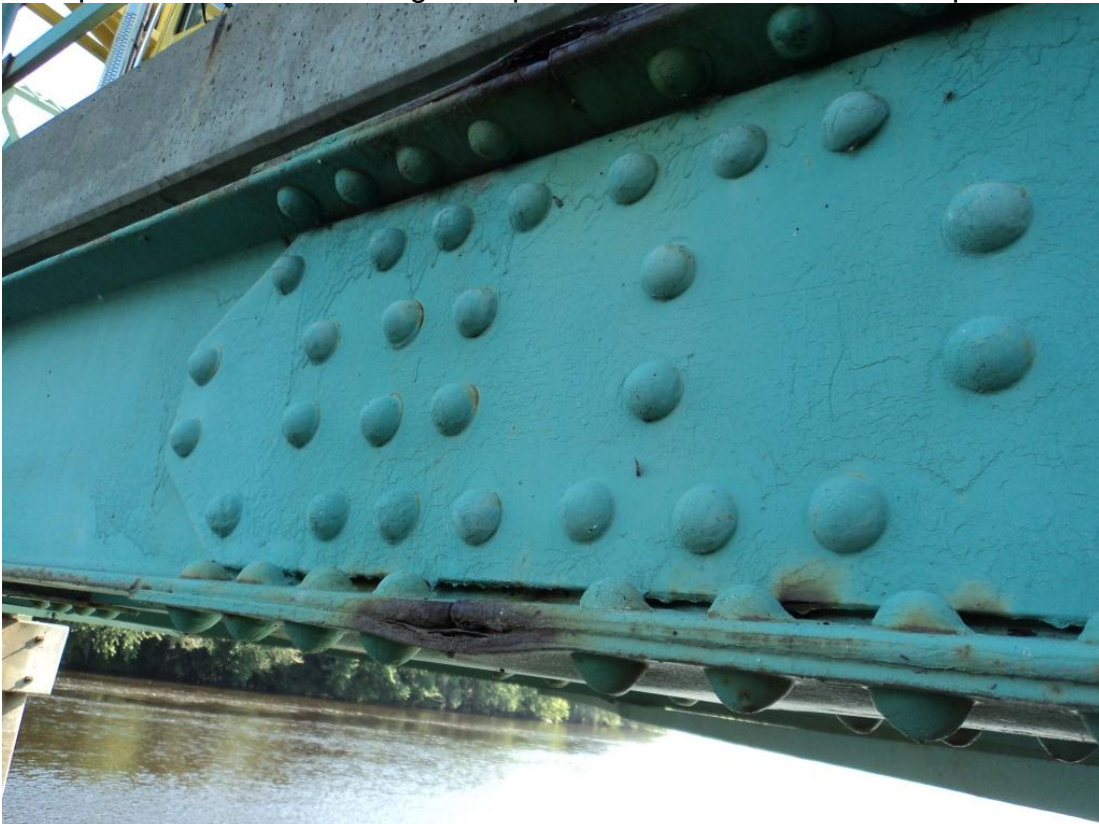
Photo 34 – Minor pack rust of the top and bottom splice plates with one inch vertical deformation was observed in the Span 3 roadway truss at the L3 lower chord splice.
