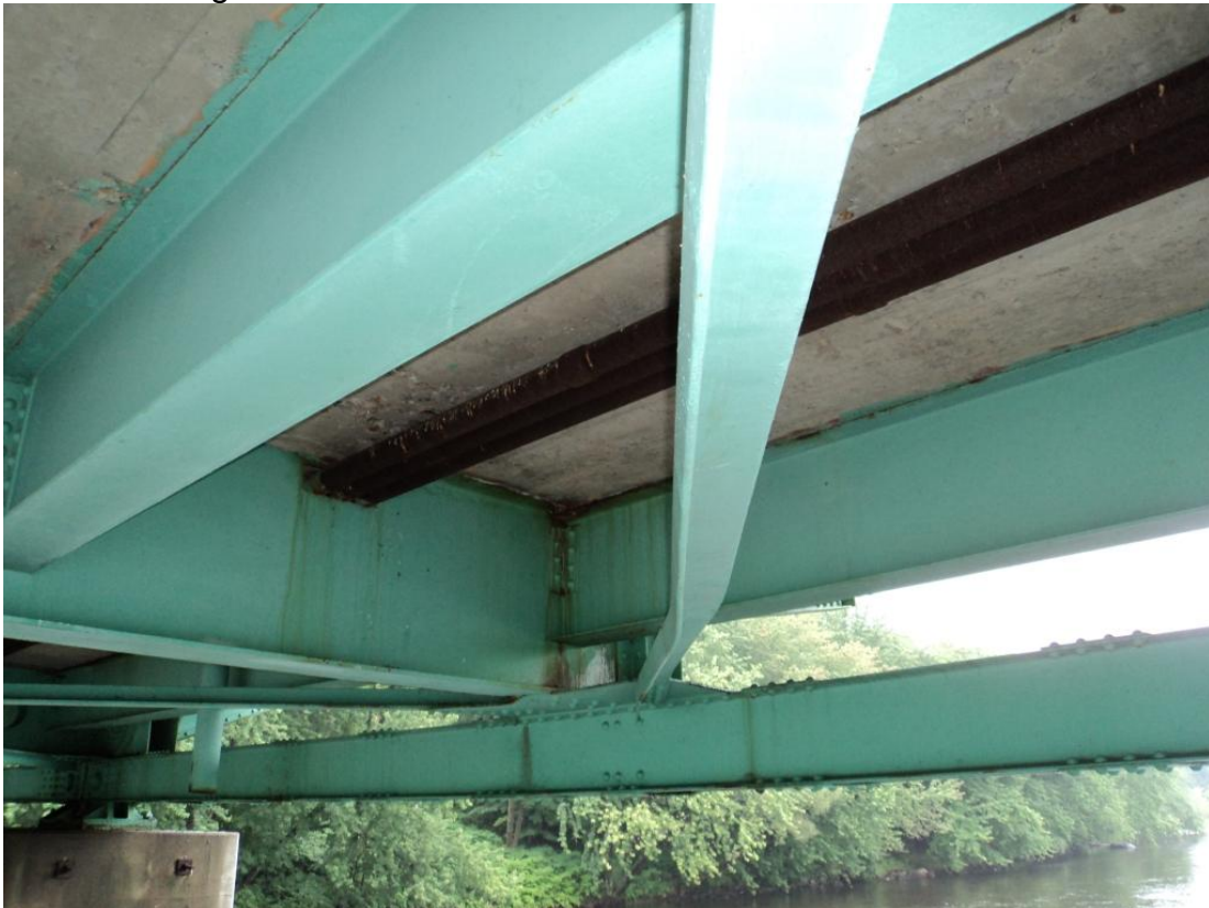
Photo 50 – Stringers generally in satisfactory condition with few defects. Note displacement in Span 2 bracing connecting FB1 sidewalk and FB2 roadway trusses.
