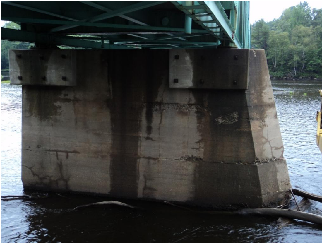
Photo 71 – Both faces of both piers have been previously retrofitted with Dywidag post-tensioned concrete encasement repairs immediately below both truss bearings.
