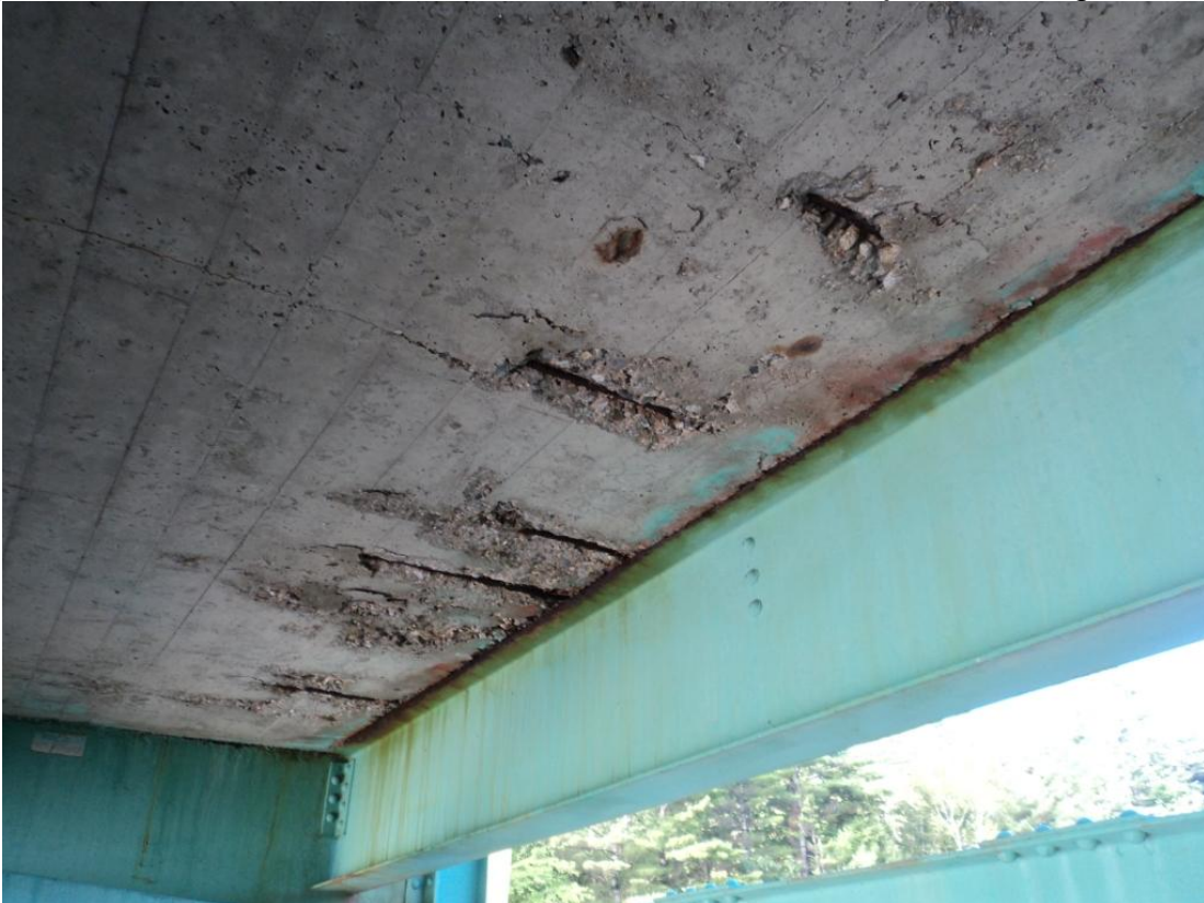
Photo 16 – In Span 3 between FB0 and FB1 five spalls with exposed reinforcing were noted between S5 and S6. View is looking south.
