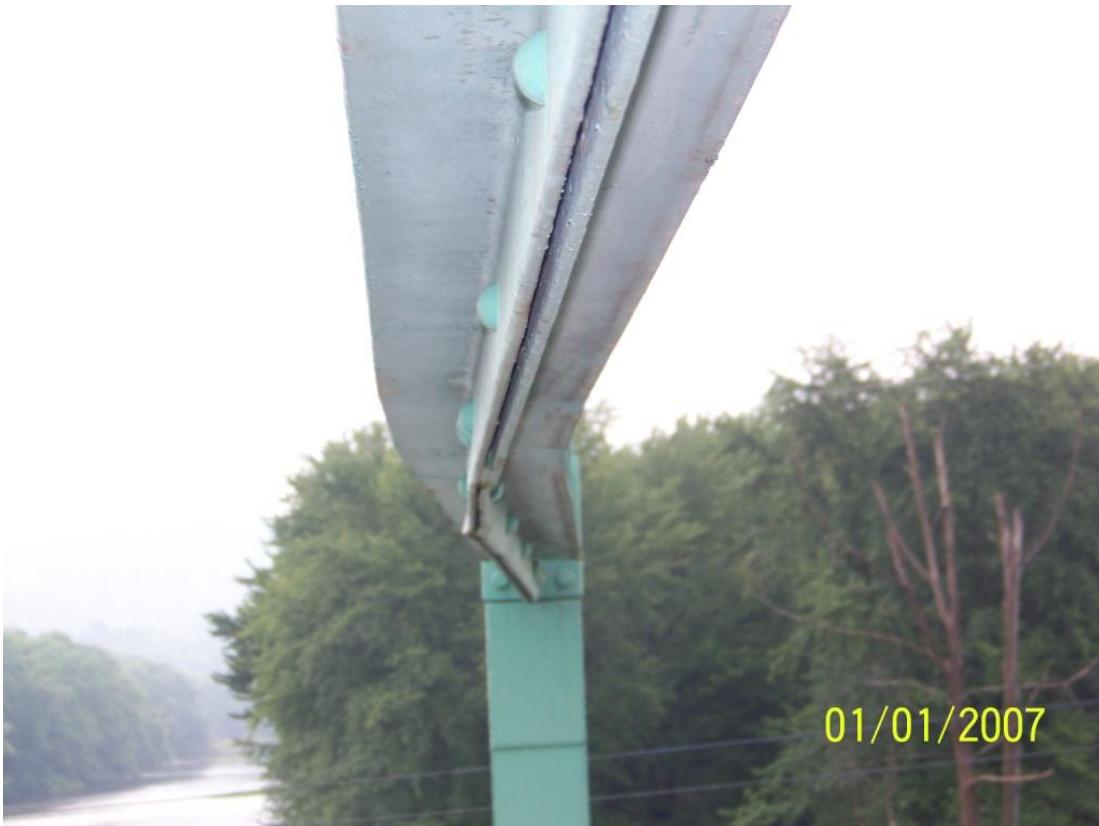
Photo 54 – Impact damage to the sway frame lower transverse member along with lateral displacement of 6 inches in the horizontal plane was observed at Span 3 U3.
