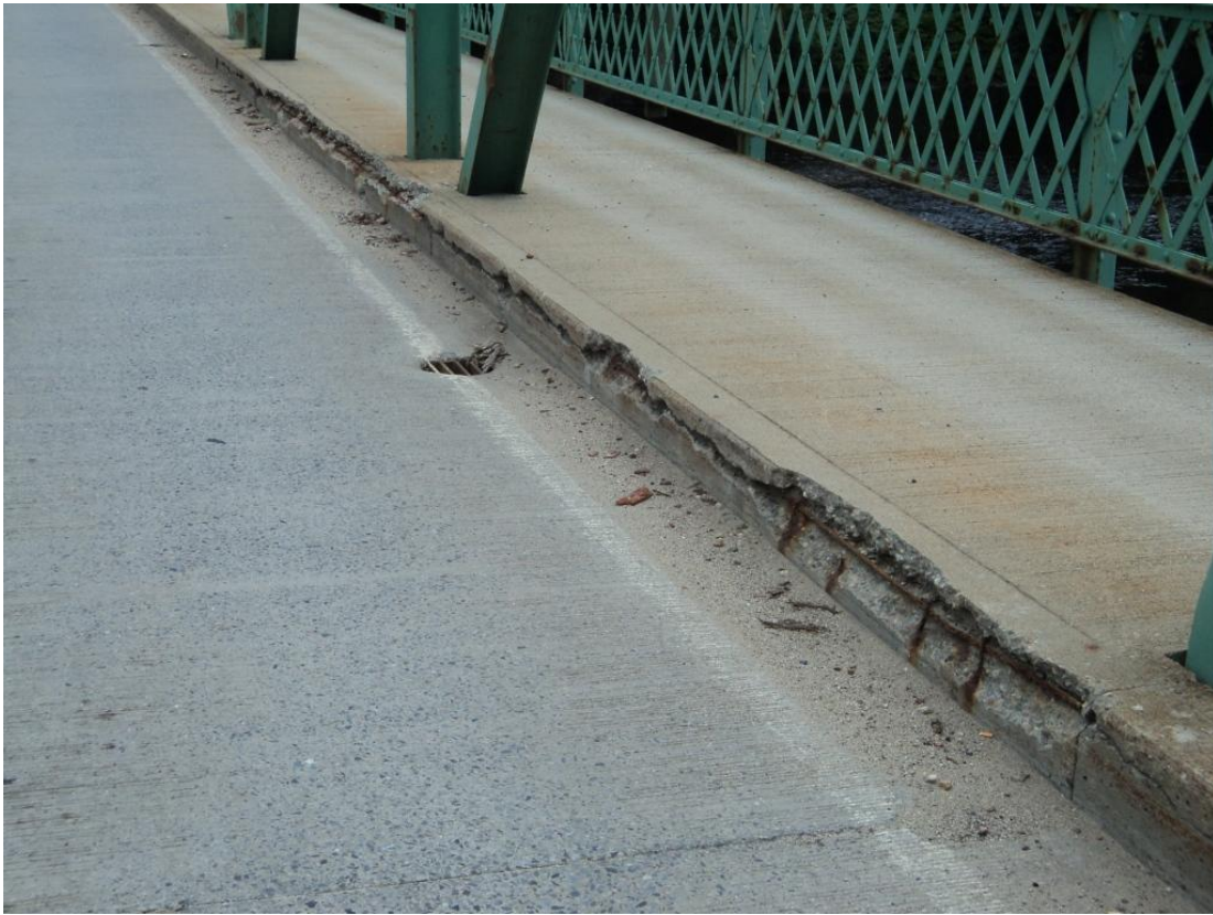
Photo 25 – The east sidewalk curb face in Span 2 has a long spall with exposed reinforcing extending from L4 to L6. Looking northeast.
