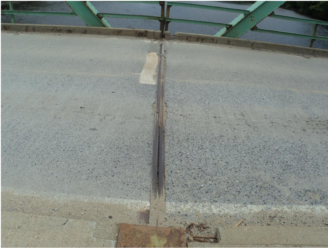
Photo 29 – The deck joint at Pier 1 has minor spalling in the near northbound lane and a one foot by 6 foot spall patched with concrete in the far southbound lane.
