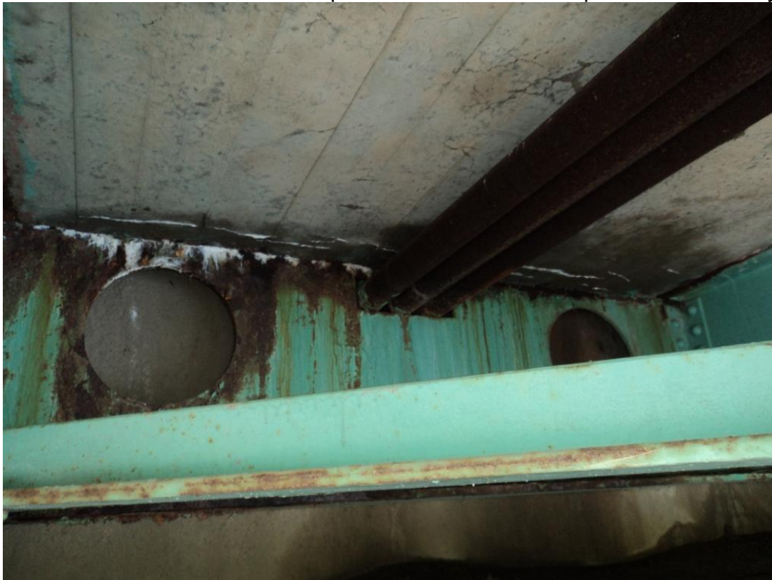
Photo 20 – Transverse cracks with heavy efflorescence were observed above FB8 in Span 3 in all bays between S3 and S6. Looking south at south abutment.
