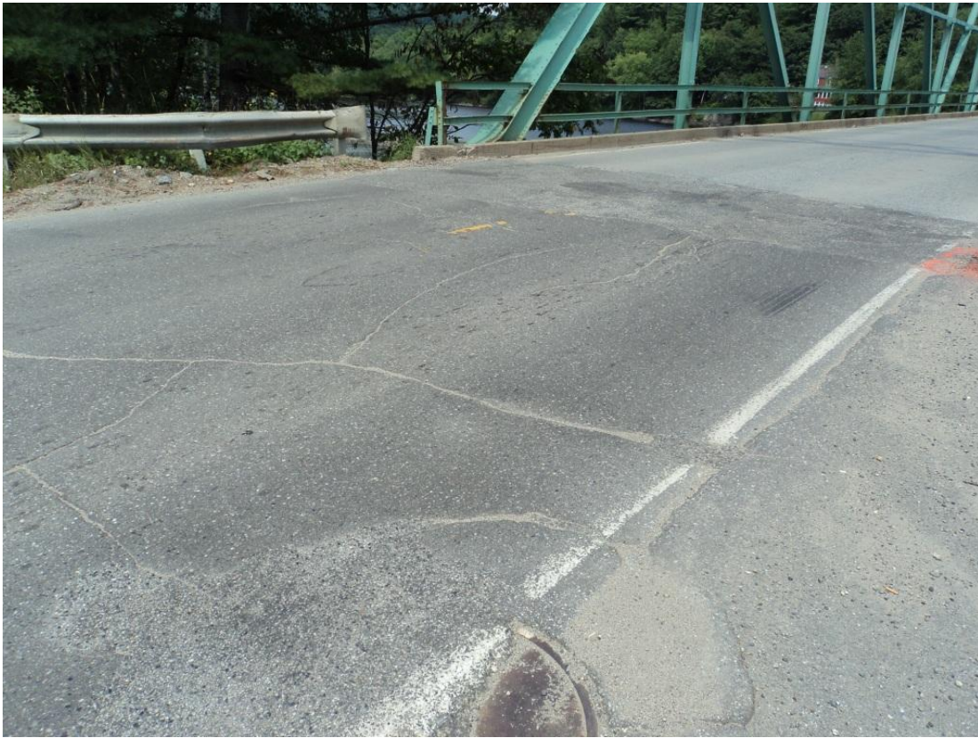
Photo 73 – The south approach pavement has numerous wide cracks and depressions which result in a rough surface. Also note substandard southwest corner guiderail.
