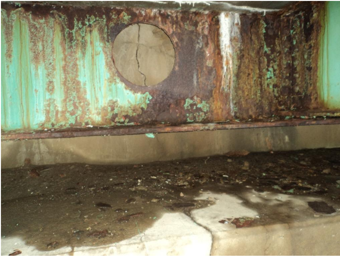
Photo 49 – The Span 3 FB8 end floorbeam has failed paint on the web and active corrosion. Looking south at south abutment between S4 & S5. Note crack in backwall.
