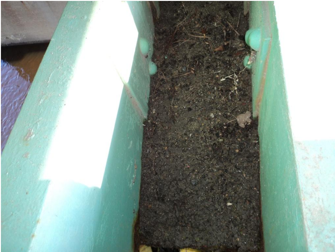
Photo 31 – The Span 3 L1-L2 sidewalk truss has up to 8 inch deep debris accumulations between the side channels on the top of the L1 lower tie plate.
