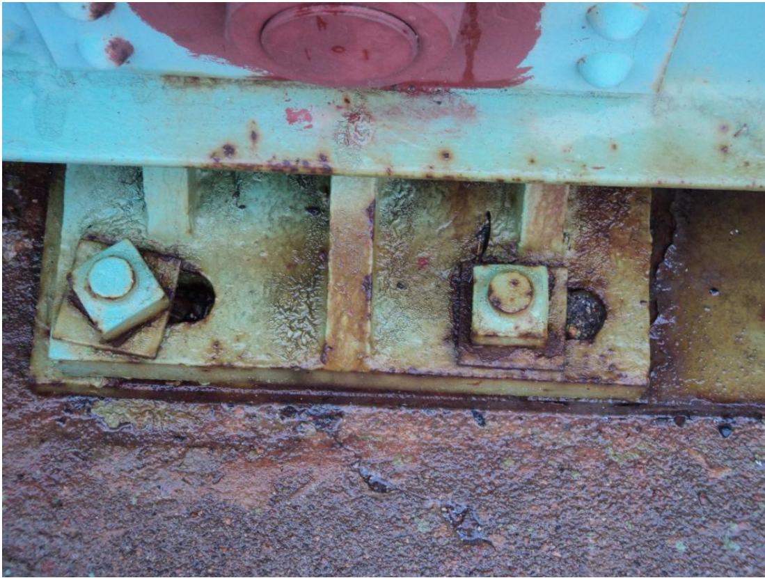
Photo 61 – The Span 1 roadway truss expansion bearing at Pier 1 has debris accumulations filling the slot for the southwest anchor bolt, inhibiting free movements.
