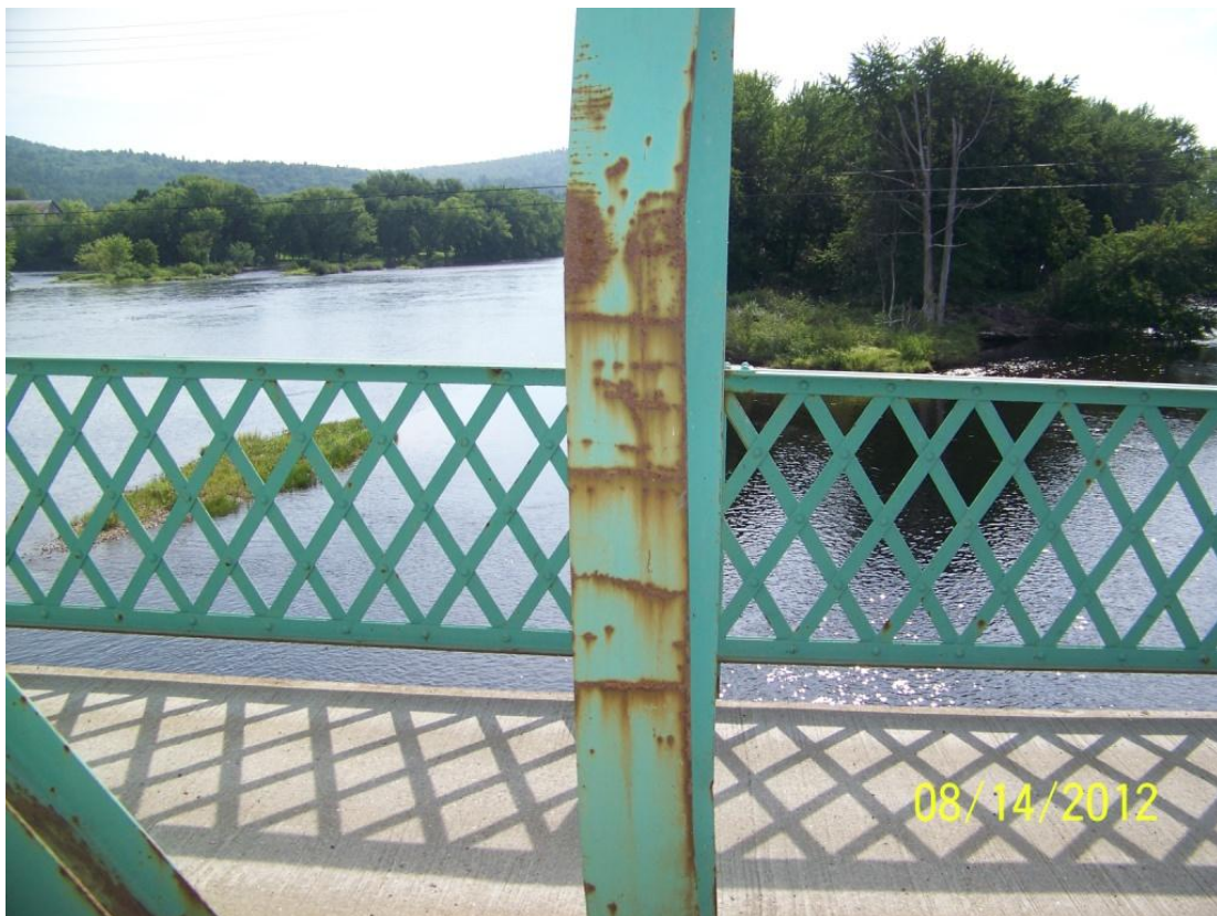
Photo 43 – Span 3 sidewalk truss U3-L3 has impact damage with up to 3 inches of lateral displacement in longitudinal direction and up to 1 1/2 inches in the transverse direction.
