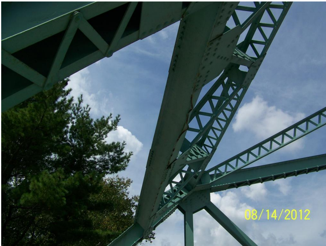
Photo 53 – Impact damage to the portal bracing at the south end of Span 3 over the northbound lane was observed.
