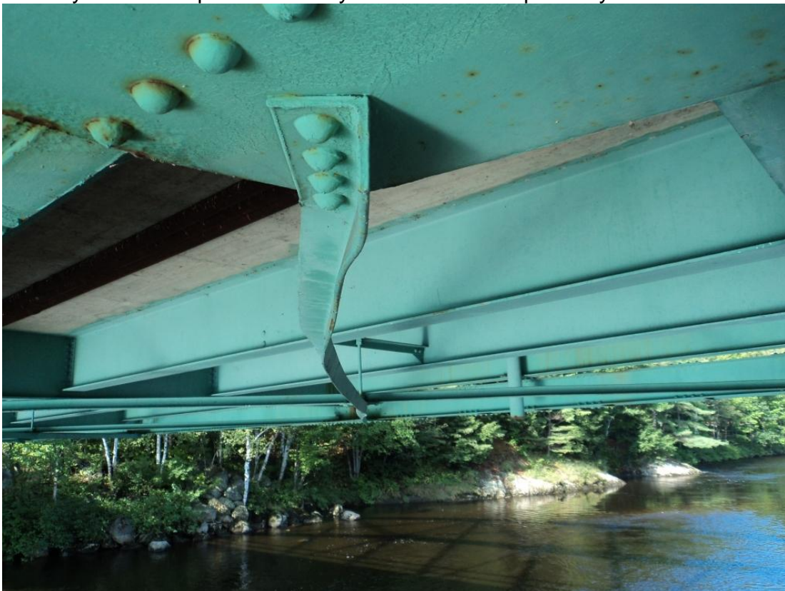
Photo 60 – The lower lateral bracing angle in Span 3 connecting the FB3 sidewalk truss and FB4 roadway truss is displaced laterally in the horizontal plane by 9 inches.
