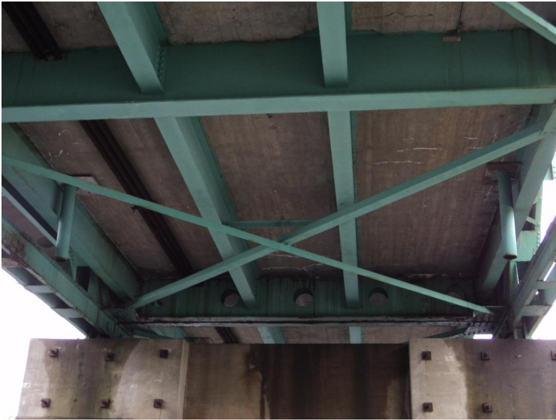
Photo 11 – Approximately ten transverse cracks with efflorescence in the underside of deck in Span 1 between FB7 and FB8, distributed in three different stringer bays.
