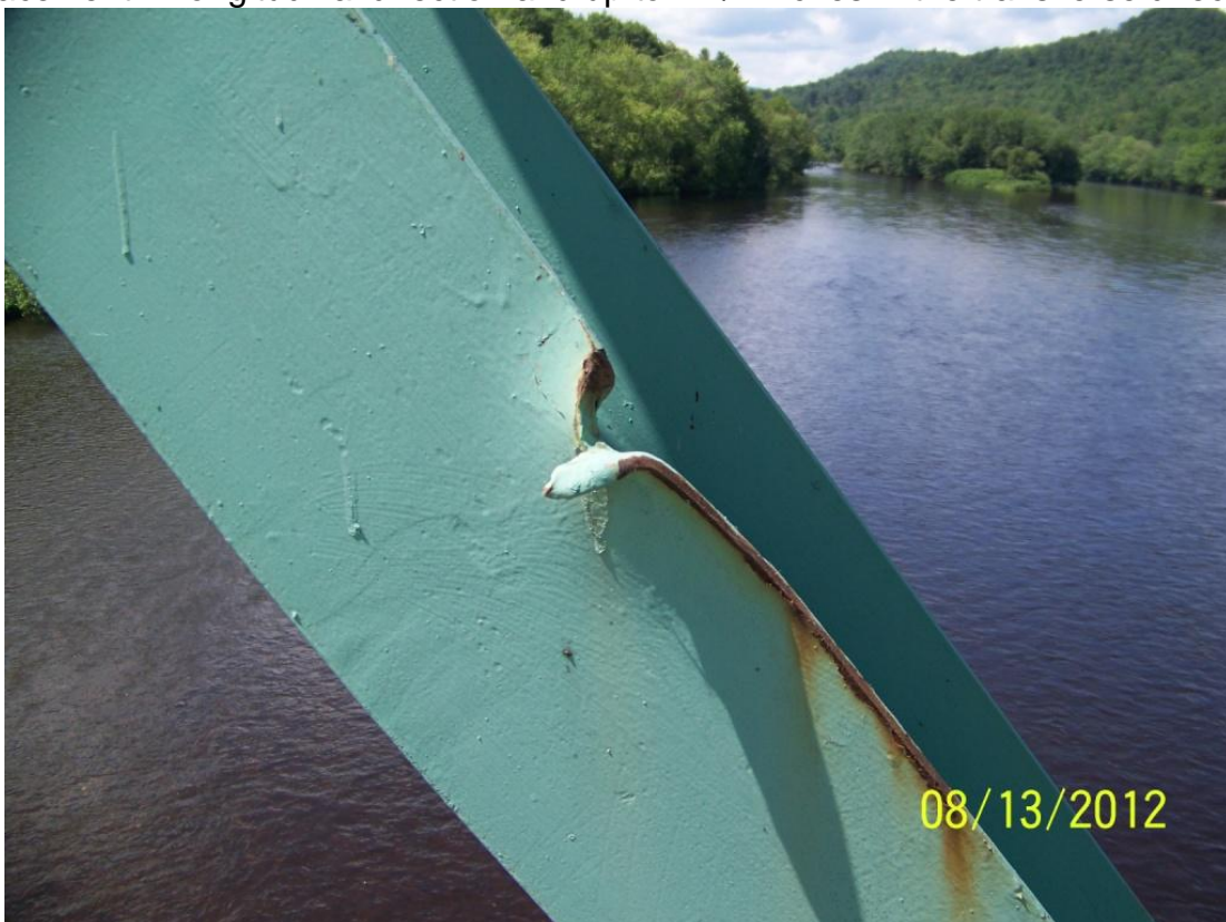
Photo 44 – Impact damage to the Span 2 roadway truss L5-U6 diagonal has resulted in a notch in the flange tip which is approximately 2 inches deep.
