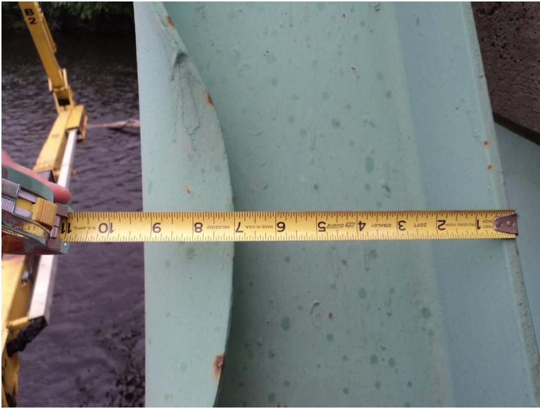
Photo 37 – The west flange of the Span 2 roadway truss diagonal U2-L3 is permanently deformed and bent inward by 2-1/2 inches. Looking north.
