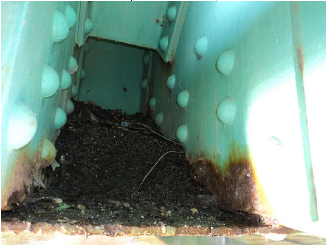
Photo 32 – The Span 3 sidewalk truss at L2 has 9-12 inch deep debris accumulations between the side channels on the lower lateral connection plate.
