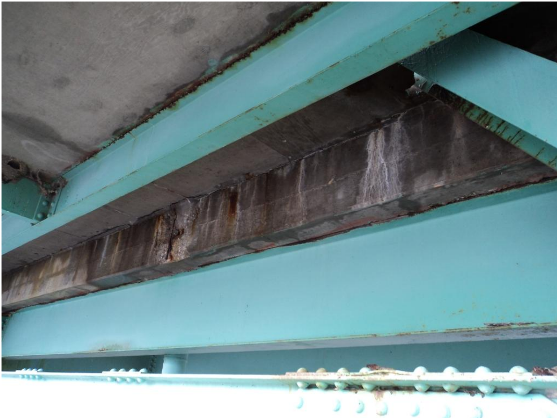
Photo 15 – A 2 foot square spall with exposed reinforcing in Span 2 between FB5 & FB6 along with efflorescence at sidewalk to deck slab construction joint. Looking southwest.
