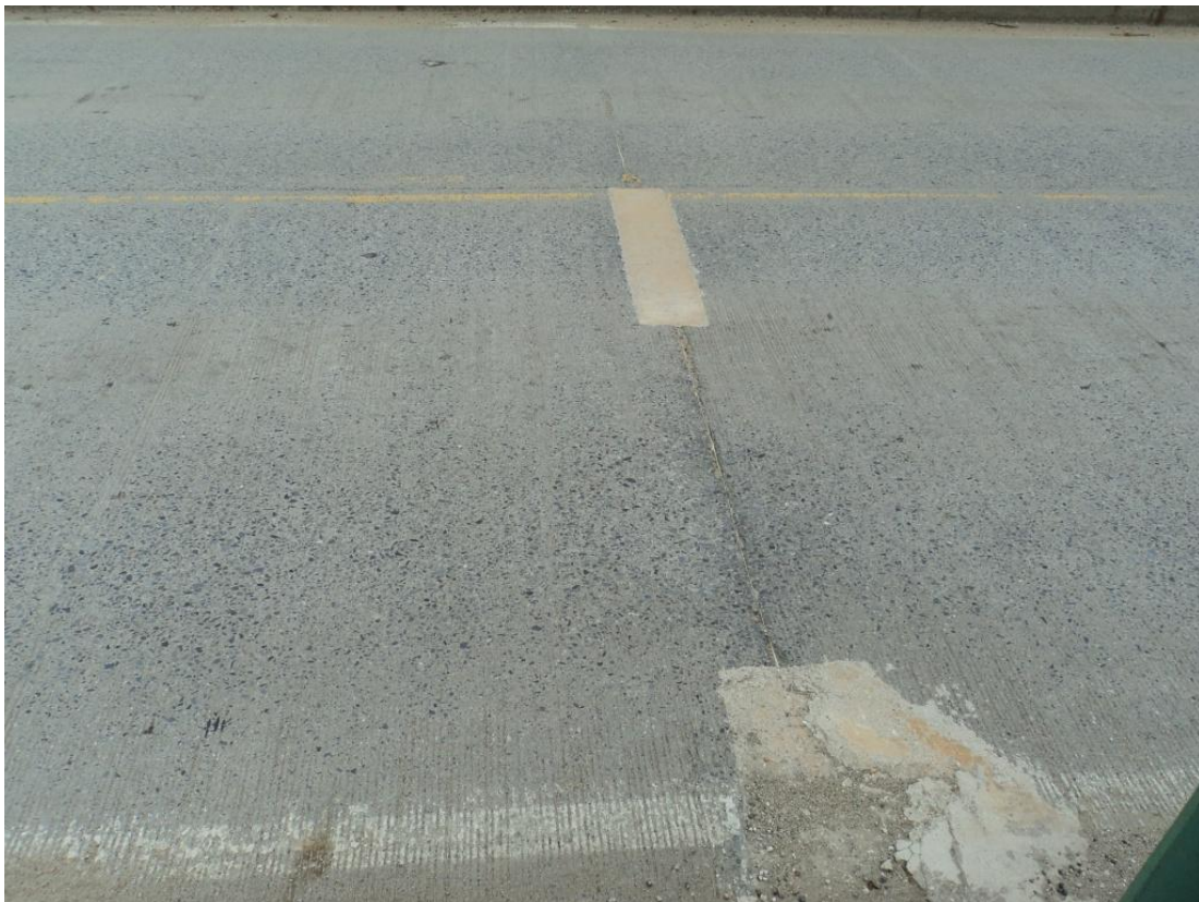
Photo 8 – Above FB7 in Span 2 the transverse construction joint has two spalls in the northbound lane measuring 1 to 2 SF in size, each patched with concrete.
