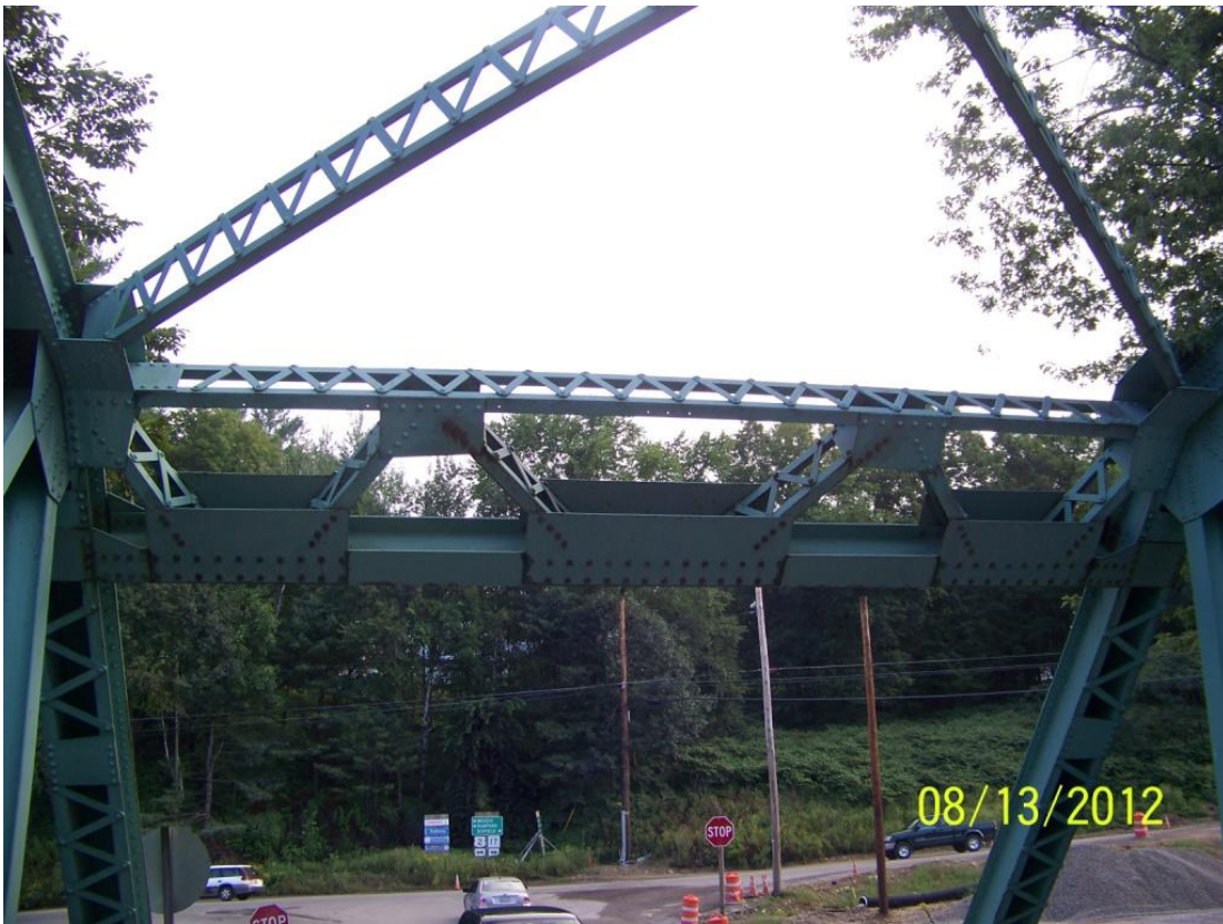
Photo 51 – The lower transverse members at portal bracing have been replaced with bolted rolled shapes at both ends of all three spans. View at north portal of Span 1.
