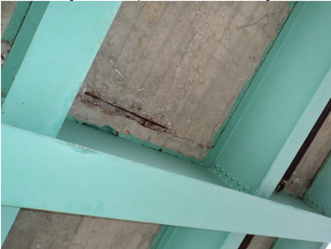
Photo 10 – Three minor spalls in the underside of deck were noted in the floorbeam haunch zones of FB6 in Span 1 in various stringer bays. View between S4 and S5.
