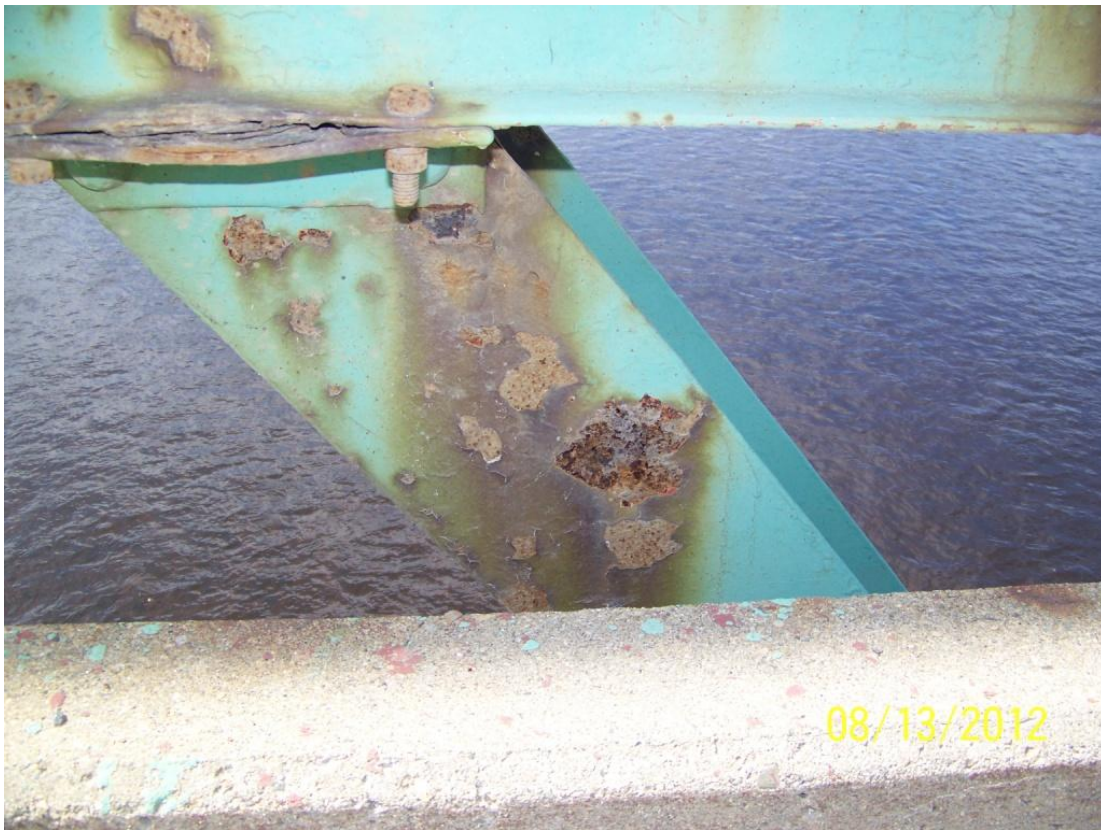
Photo 41 – Span 2 roadway truss L5-U6 diagonal has section loss on the east face of the flange up to 3/16 inch deep and 4 inches wide located at top of curb level.
