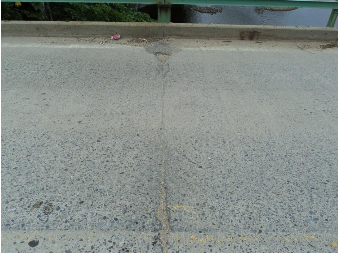
Photo 6 – Above FB4 in Span 3 the transverse construction joint has a one foot square spall patched with bituminous material along the west curb. Looking west.
