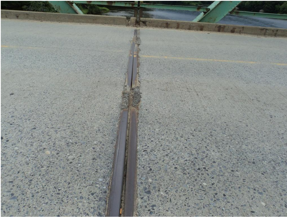
Photo 27 – Pier 2 deck joint has minor spalling with bituminous patches and the joint opening varies along the length of the joint from \frac{3}{4} inches to zero at roadway centerline.
