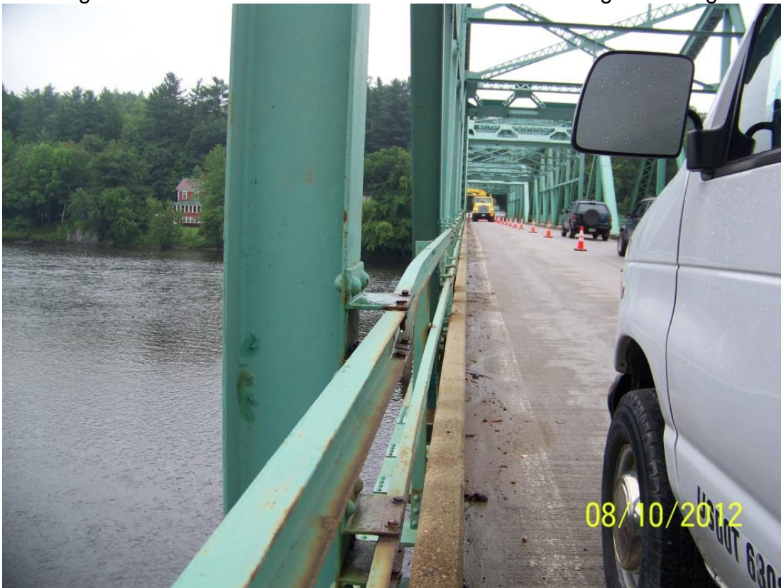
Photo 22 – Impact damage to the west traffic railing was observed in Span 3 at L5. Looking north in southbound lane.
