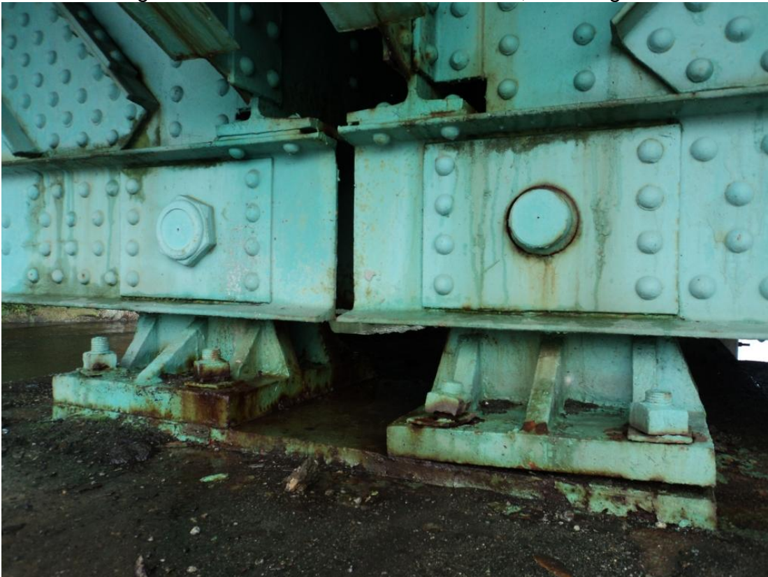
Photo 62 – The bearing pin nuts are missing on the east faces of both truss line lower chords at Span 2 expansion bearings on Pier 2. Looking west with Span 2 on right.
