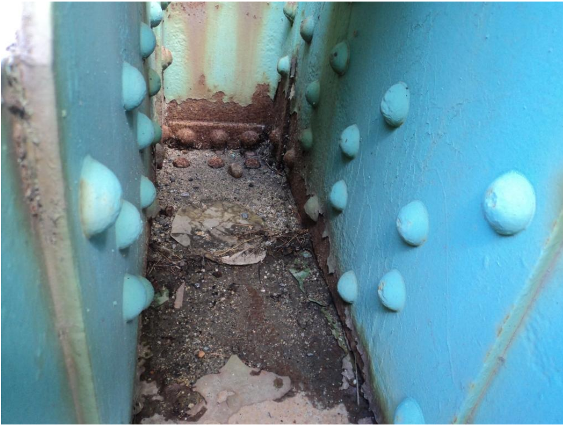
Photo 33 – Active corrosion was observed in lower chord bottom interior surfaces along with lower portions of vertical and gusset plates at sidewalk truss L6 in Span 3.
