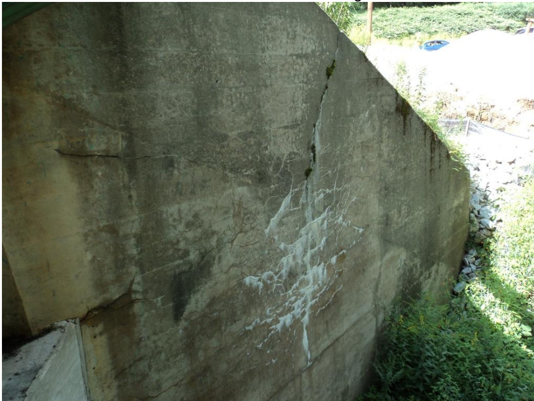
Photo 68 – The northeast wingwall has map cracking with efflorescence.
