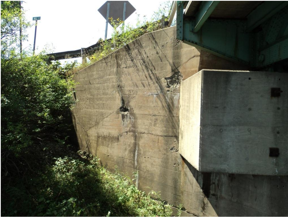
Photo 69 – The southeast wingwall is in fair condition with two spalls less than 2 SF each in size and a medium vertical crack extending from the top to the base.
