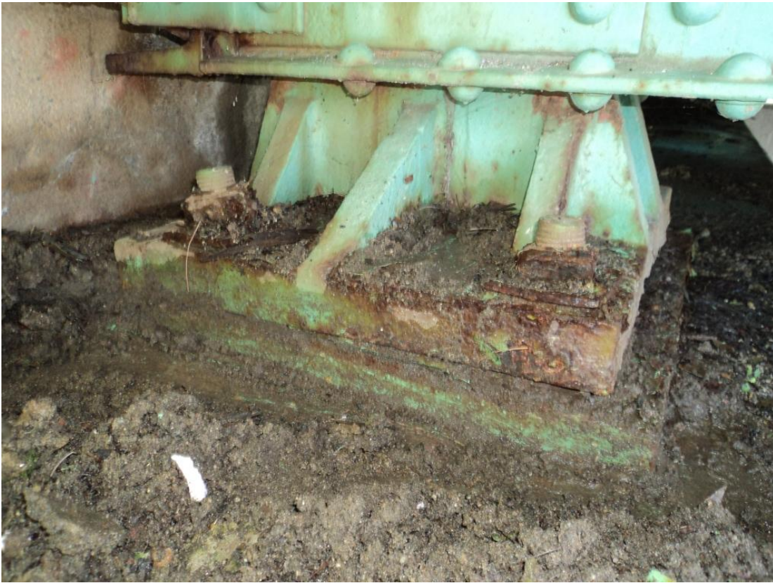
Photo 65 – South abutment expansion bearings have heavy 3-4 inch deep debris accumulations around the bearing and also filling the anchor bolt expansion slots.
