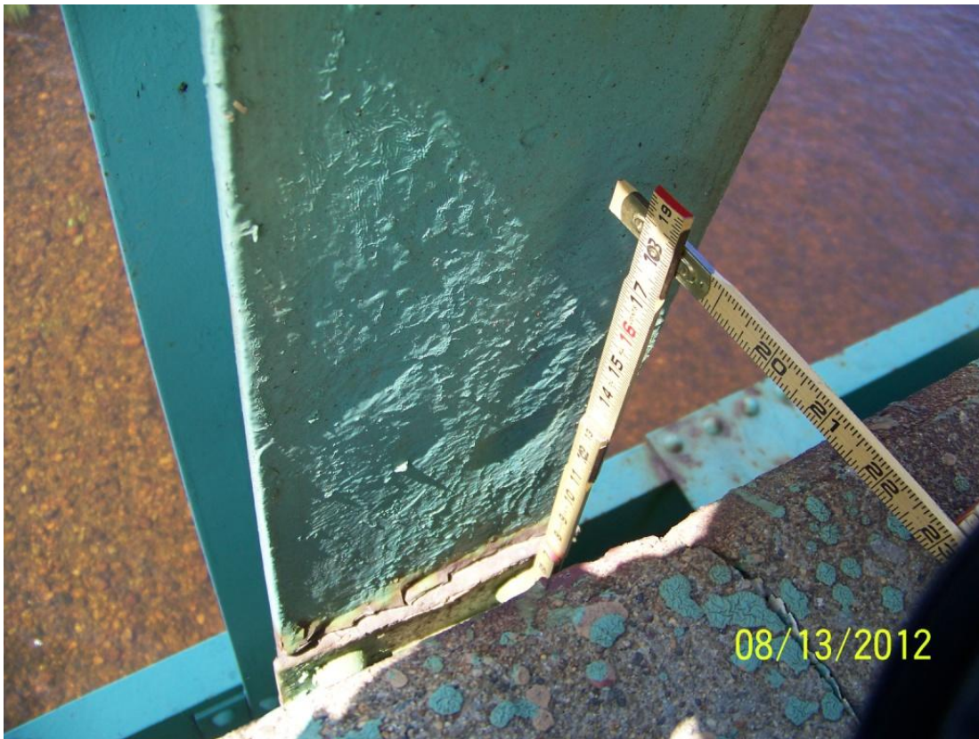
Photo 39 – The Span 2 roadway truss U7-L7 vertical has section loss on east face of flange up to 3/16 inch deep and 2 inches wide located a foot above top of the floorbeam.
