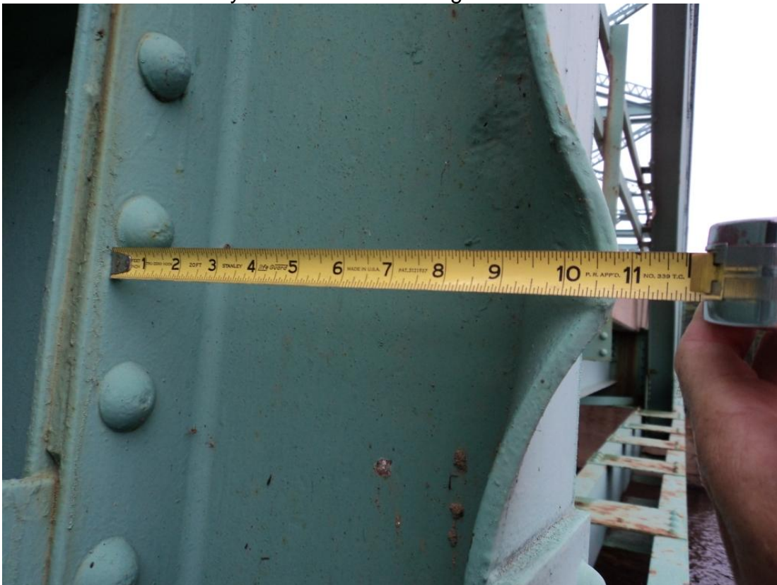
Photo 38 – The west flange of the Span 2 roadway truss vertical U3-L3 is permanently deformed and bent outward by 1-1/2 inches. Looking south.
