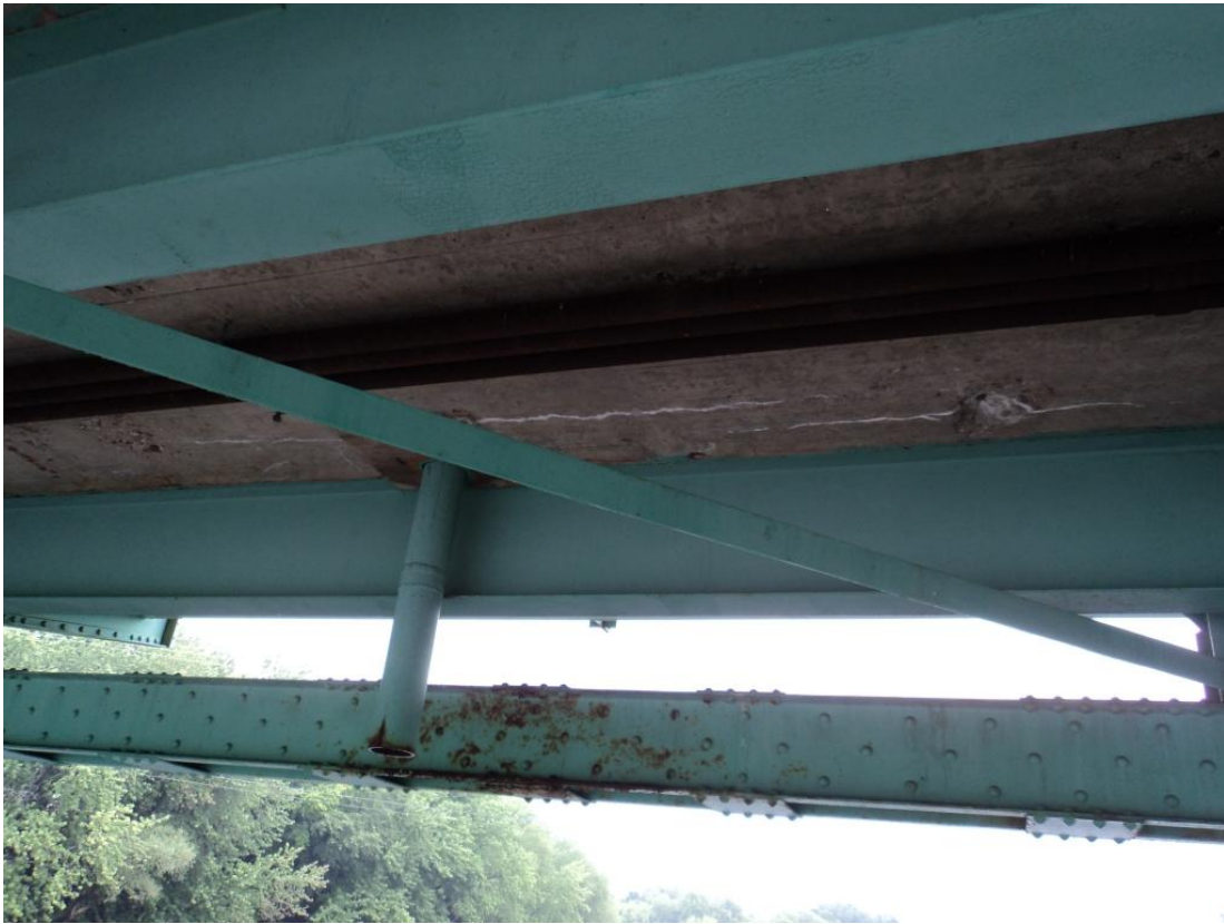
Photo 13 – In Span 2 between FB3 and FB4 a longitudinal crack with efflorescence was observed between S3 and S4 located just inboard of the east curbline. Looking east.
