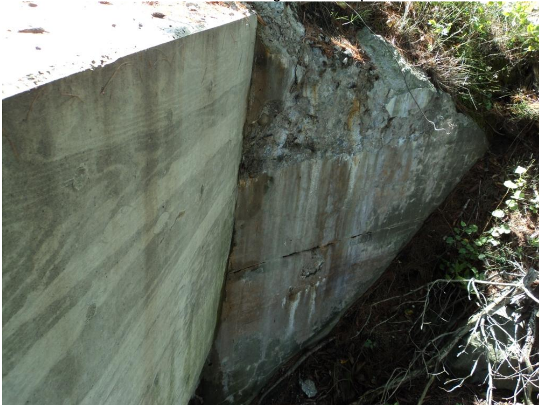
Photo 70 – The southwest wingwall is in poor condition with a large deep spall continuous along the top for full length of the wingwall.
