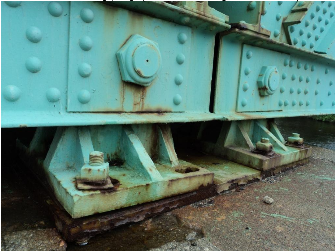
Photo 64 – The Span 2 roadway truss expansion bearing on Pier 2 is missing the southwest corner anchor bolt. Looking southeast with Span 2 on left, Span 3 on right.
