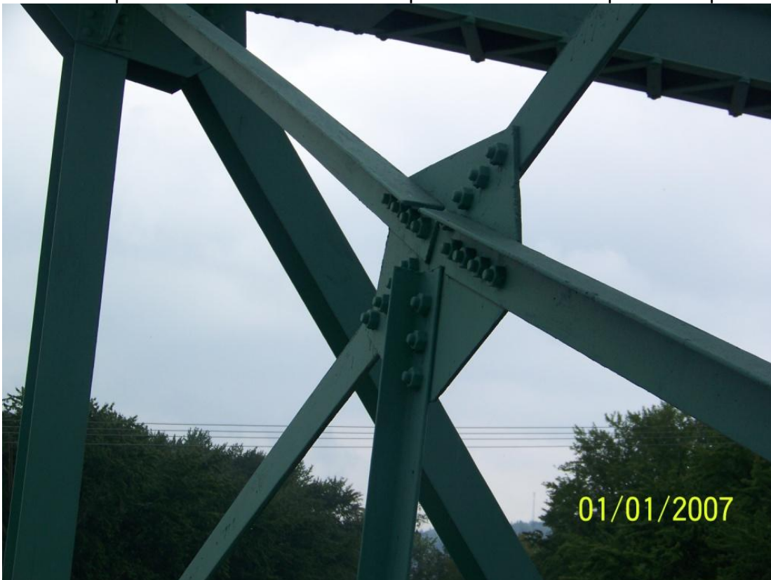
Photo 52 – High strength bolted repairs were observed in various sway frame connections including the diagonal intersection connection plate at Span 3 U3.
