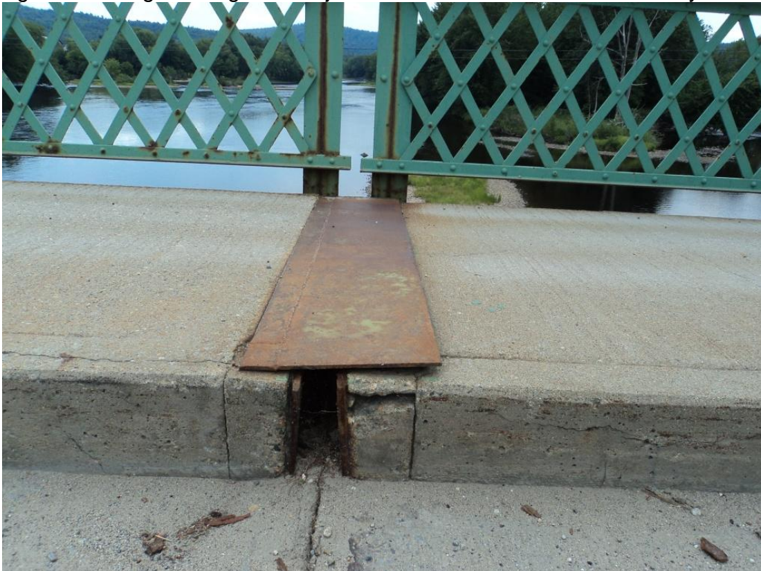
Photo 28 – The sidewalk sliding plate joint at Pier 2 projects upward \frac{3}{4} to one inch at plate corner, creating a tripping hazard. Similar condition was observed at Pier 1 joint.
