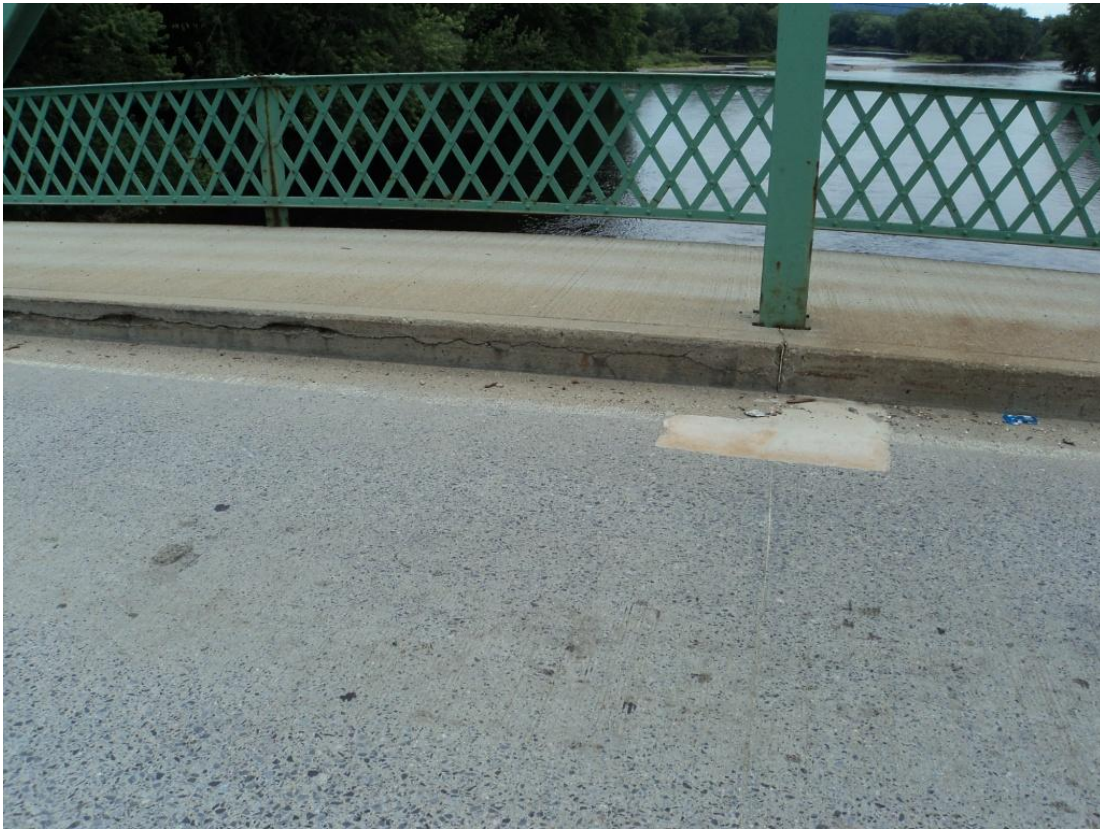
Photo 9 – Above FB7 in Span 1 the transverse construction joint has a 4 SF spall in the northbound lane along the east curb, patched with concrete. Looking east.
