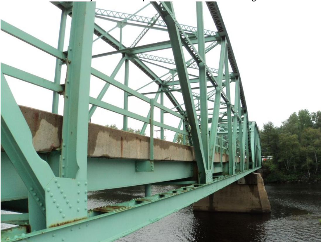
Photo 36 – At L3 in Span 2 roadway truss the vertical and diagonal have sustained damage at 2 feet above the lower chord, with localized twisting of the flanges.
