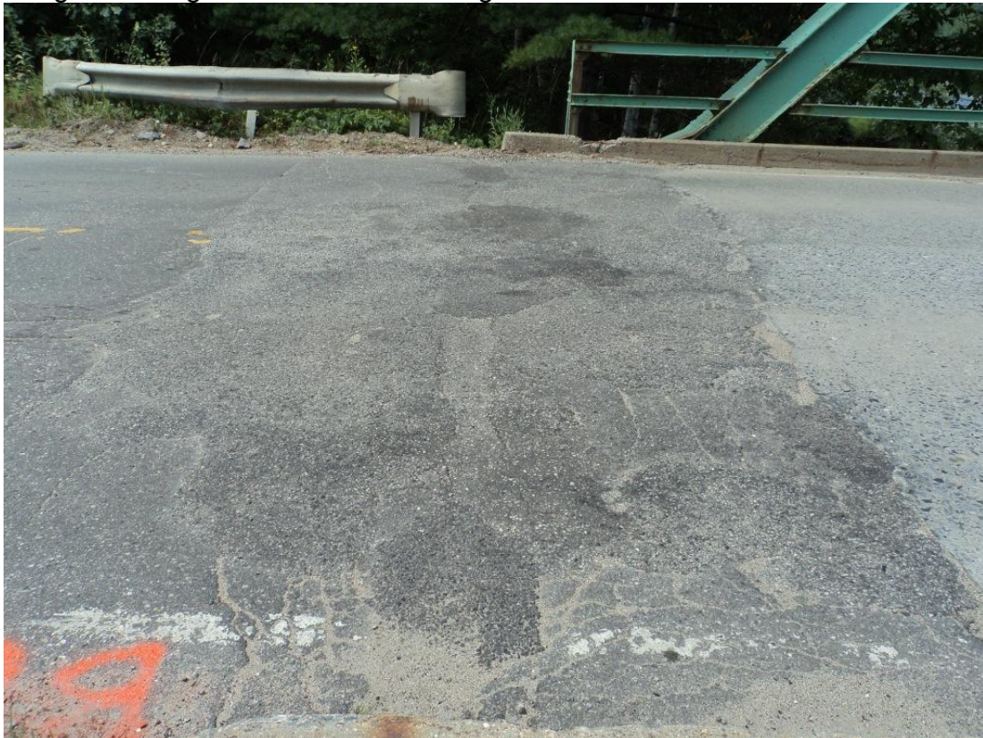
Photo 26 – South abutment bituminous pavement patch is deteriorated with extensive successive patches, resulting in a rough riding surface at the concrete bridge deck.
