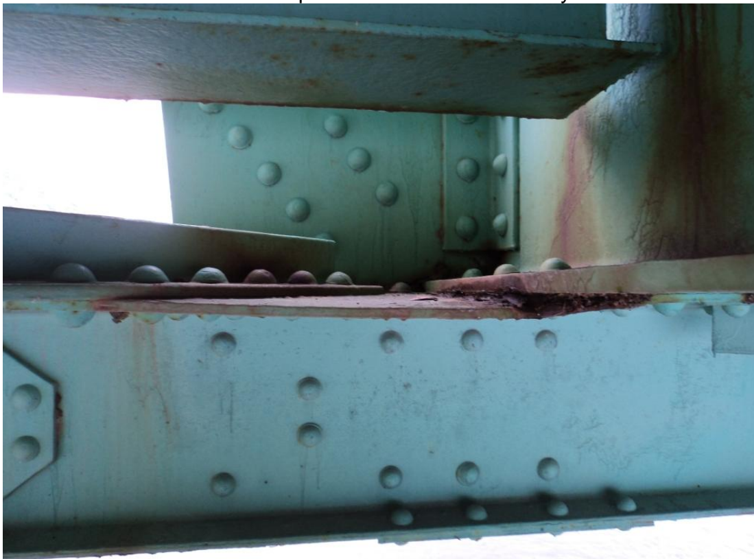
Photo 58 – In Span 2 at FB5 roadway truss lower lateral connection pack rust at floorbeam flange edge has bent the connection plate down by approximately one inch.
