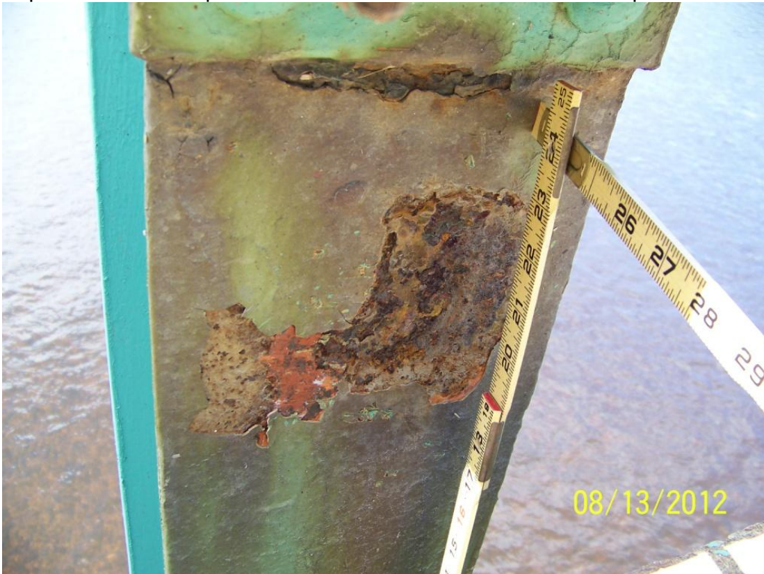
Photo 40 – Span 2 roadway truss U6-L6 vertical has section loss on east face of flange up to 1/4 inch deep and 4 1/2 inches wide located two feet above top of floorbeam.
