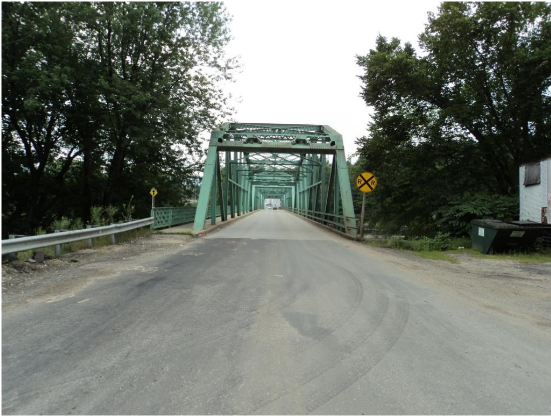
Photo 75 – Approach guiderail at the northeast corner is substandard due to lack of stiffening and proper attachment to bridge railing. Northwest corner is missing guiderail.
