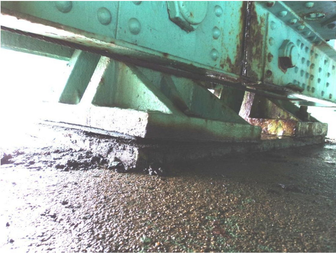
Photo 63 – Span 3 sidewalk truss bearing at Pier 2 has a cracked bearing pin nut and lower half of the nut is missing (at right). Also note missing anchor bolt in Span 2 bearing.
