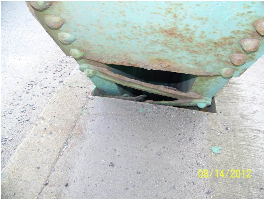
Photo 35 – At the Span 1 L0-U1 sidewalk truss end post, a severed lacing bar due to section loss was observed just below top of sidewalk level. Looking north.
