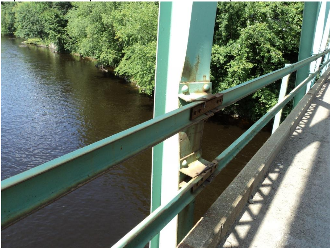
Photo 42 –The Span 1 roadway truss U5-L5 has sustained impact damage at railing level with localized twisting over a three foot length and a permanent bend in the flange tip.
