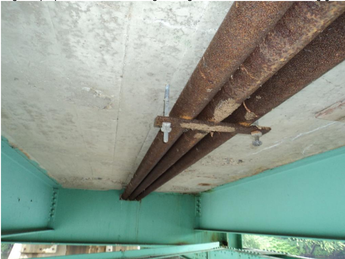
Photo 76 – Three under-deck utility pipe conduits are located between S3 and S4 running full length of the bridge. Looking north. Note hanger rods embedded in deck.
