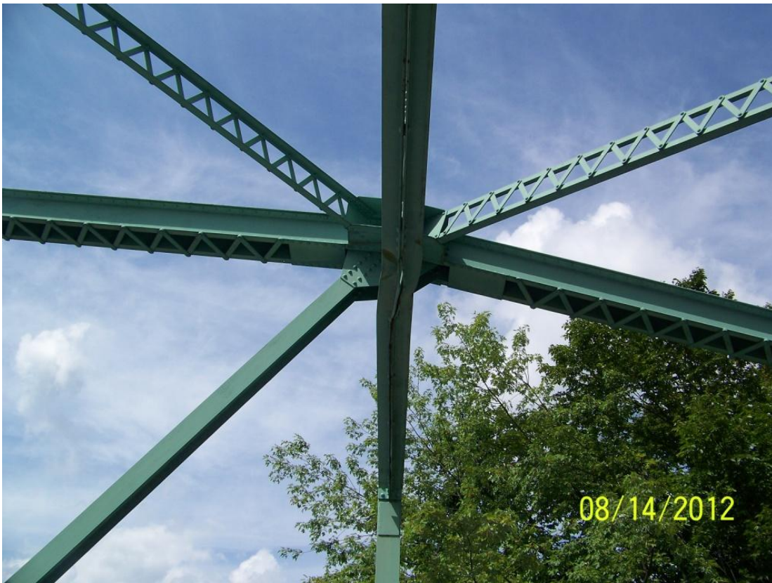
Photo 57 – Sway frame lower transverse member impact damage at Span 1 U2 over southbound lane. Also note welded plate on vertical below sway frame strut.
