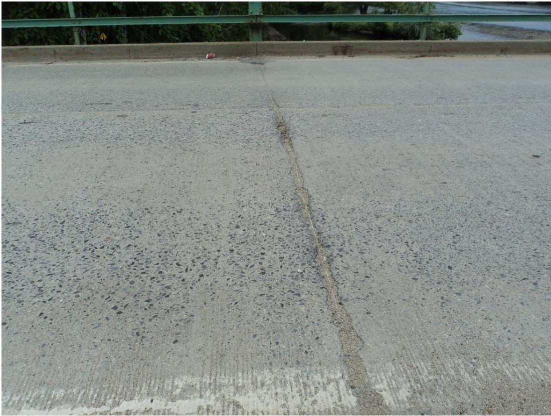
Photo 5 – The transverse construction joint above FB7 in Span 3 has minor spalling of the edges of the joint for the full width of the northbound lane. Looking west.
