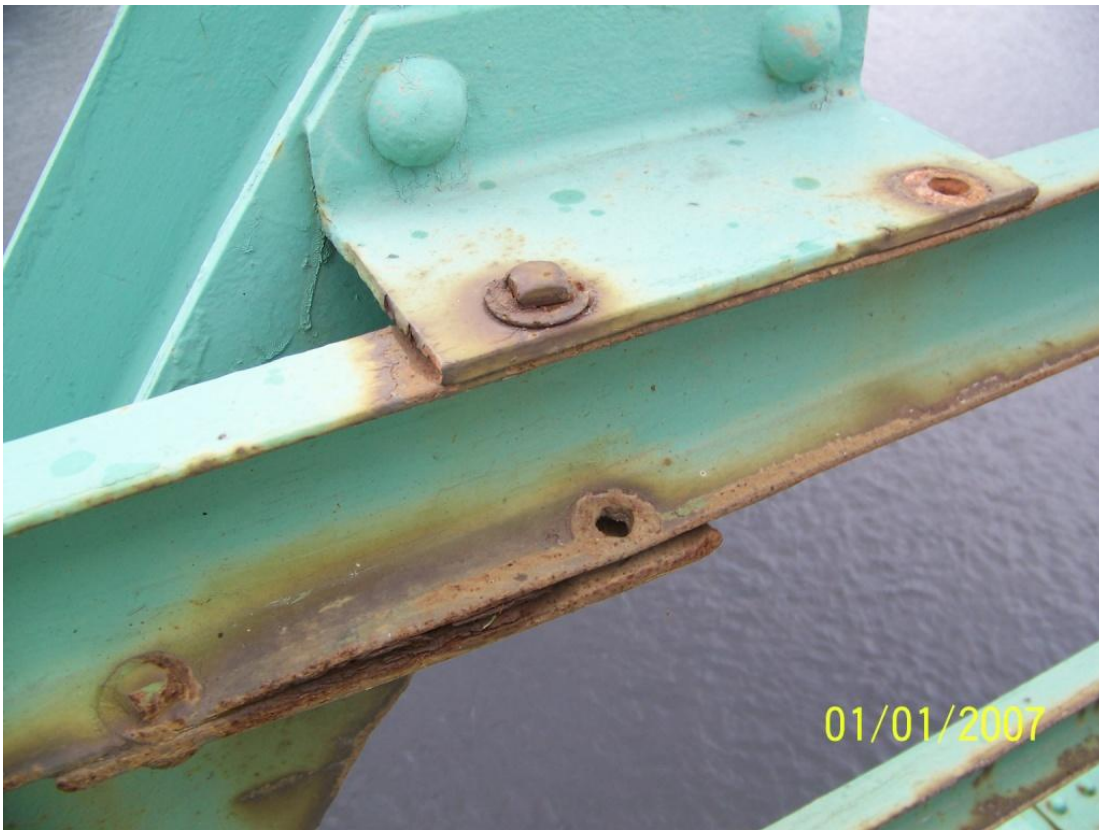
Photo 23 – A few missing bolts were observed at the connections of the railings to the attachment angles at verticals or diagonals. View is at Span 3 U3-L4.
