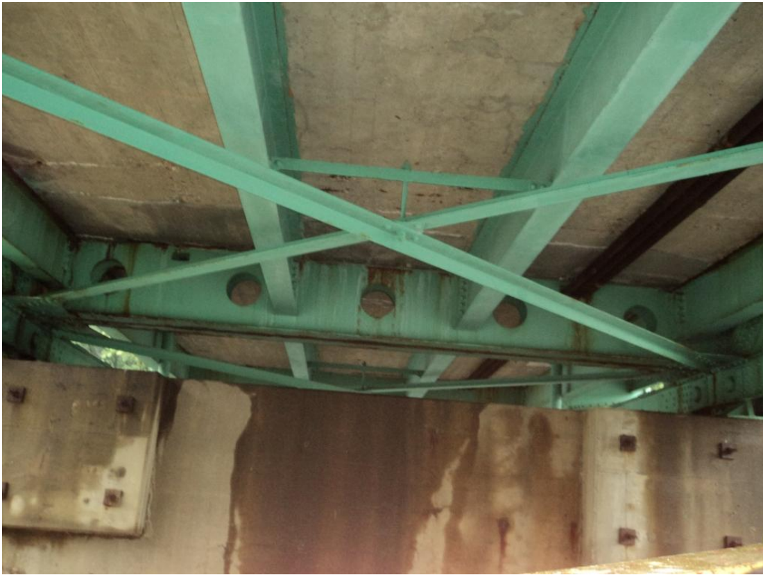
Photo 17 – Above FB0 in Span 2 all three stringer bays have been patched with repairs measuring 4 feet long by full width of the bay. Looking north at Pier 1.
