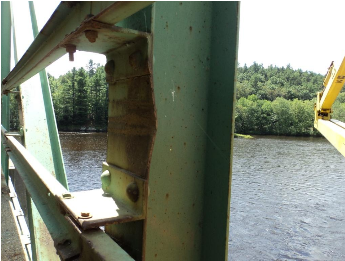
Photo 45 – At L6 in the Span 1 roadway truss the vertical U6-L6 has sustained impact damage and a permanent bend in the flange tip. Looking south.
