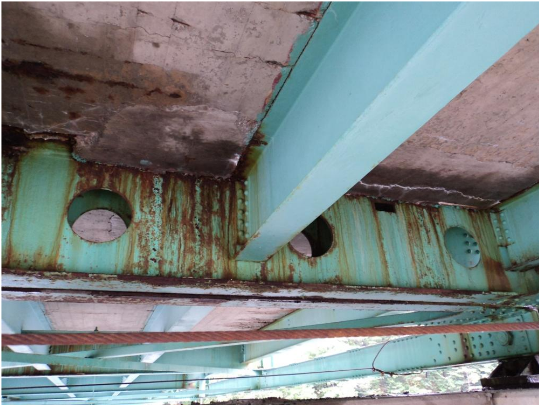
Photo 19 – Above FB8 in Span 2 a 1 foot by 2 foot spall was observed in the floorbeam haunch zone between S4 and S5 at top left. Also note concrete patches in both bays.
