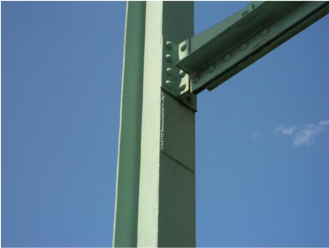
Photo 47 – Field-welded plates added to many verticals just below existing lower transverse sway frame members to cover open holes of original sway frame connections.
