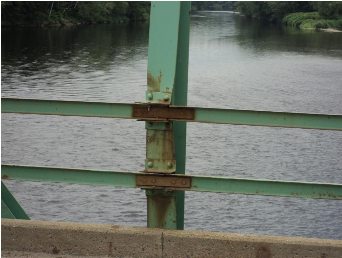
Photo 21 – West traffic railing in Span 1 at L5 has a splice in both rails to repair previous impact damage. Note truss vertical is rotated from collision damage. Looking west.
