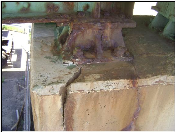
Pier 12: Cracking at East Girder Bearing.
