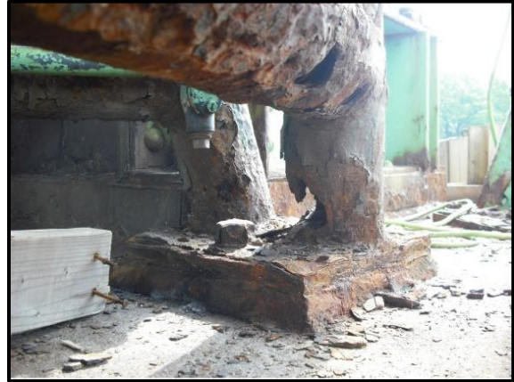
West Screw Housing Brace at Pier 21: Severe deterioration with up to 50 percent of cross-sectional area lost.
