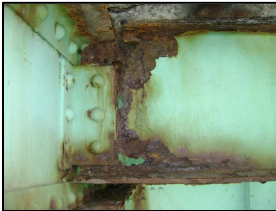
Span 10, Bay 3: Curb Stringer S1 (West) Deterioration.
