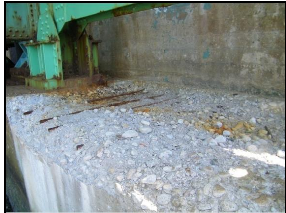
Pier 13, Bridge Seat: Up to 4 inches of erosion on the bridge seat with exposed rebar.
