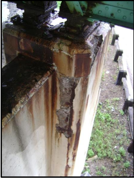
Pier 3, West Column: Concrete Deterioration with Exposed Reinforcing.
