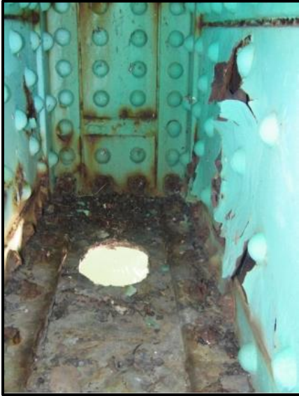
Truss Span 1, Joint L2 West: Interior of Bottom Chord at joint. Vertical web and splice plate shown in back of photo. Conditions typical of interior of bottom chord at joints.
