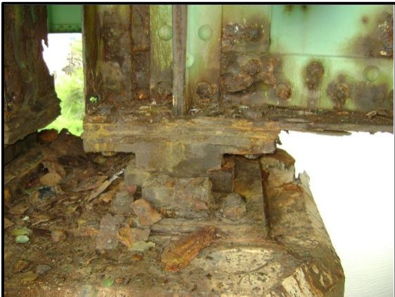
West Girder, Span 3: Bearing Deterioration at Pier 3.
