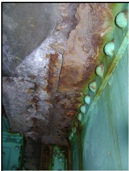
Span 6, Floor Beam 3: West Cantilever Top Flange Deterioration at End of Tie Plate.
