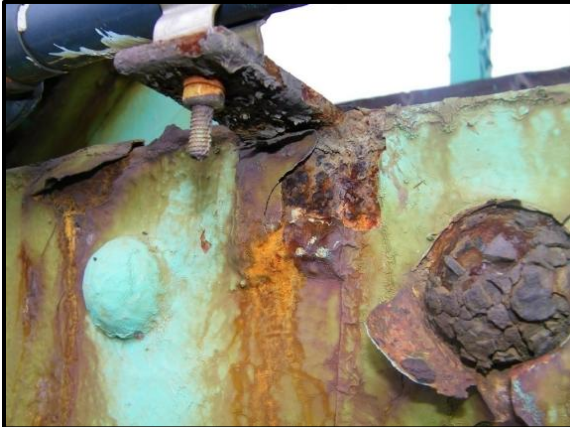
Truss Span 3, Bottom Chord L3-L4 West: Welded utility connection to bottom chord. Surface rust on top flange and web. Heavy corrosion on rivet head.
