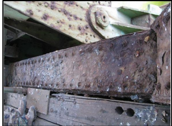
Pier 17 (South Tower), South Cross Girder: Laminar corrosion with corrosion holes on top flange. Condition typical of Cross Girders at Towers.
