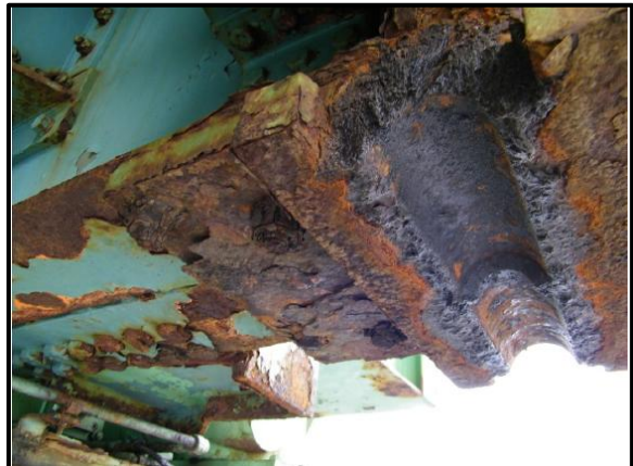
Retractable Railroad Approach Span Bearing. Northwest bearing shown. Laminar corrosion and section loss to bolt nuts typical of Bearing Plates.
