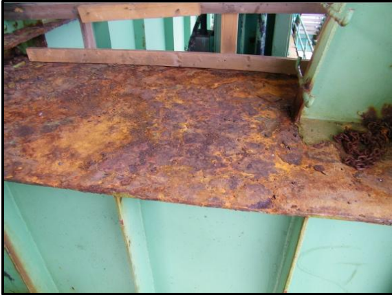
Retractable Railroad Approach Span 21, North Lifting Girder: Laminar corrosion on top flange over full-length, with more severe corrosion at ends, adjacent to knee brace.
