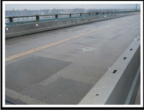
Existing Typical Deck Repairs: Walk-way at left is not a public sidewalk. Note jersey barriers at left and steel beam at right, added in 2012 due to inadequate stringer end connections. (Source: 2013 Bridge Report).
