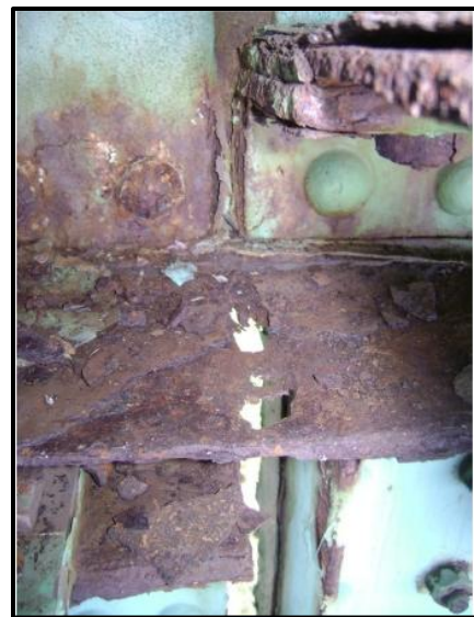
Span 13, West Girder: Bottom Flange Hole at Hinge near Pier 13.
