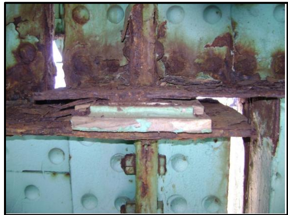
Span 13, East Girder: Bottom Flange Deterioration at Hinge near Pier 13.
