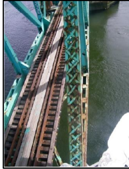
Truss Span 4, Diagonal U3-L4 West: Surface rust on top flange and lacing bars. Condition typical of diagonals.
