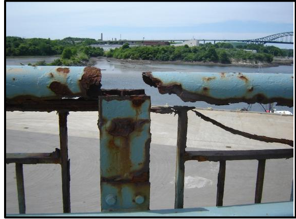
Typical Deterioration at Bridge Rail.
