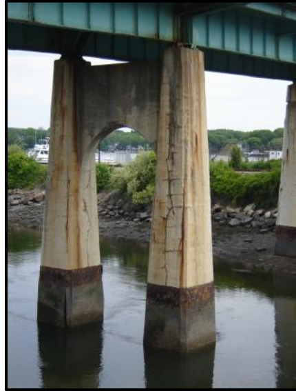
Pier 6: South Face Deterioration.
