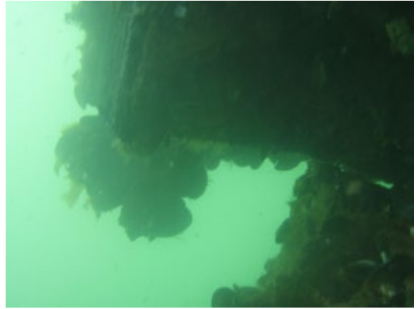
Severed H-Pile pier #6 corner Pile #7
