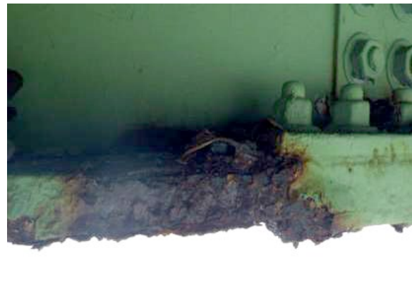
Corrosion and pitting at splice connection
