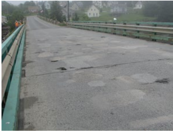
Concrete wearing surface deterioration
