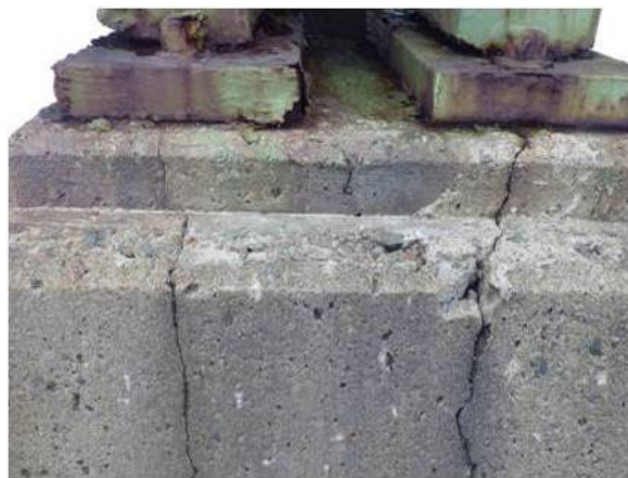
Cracking at end of pier cap
