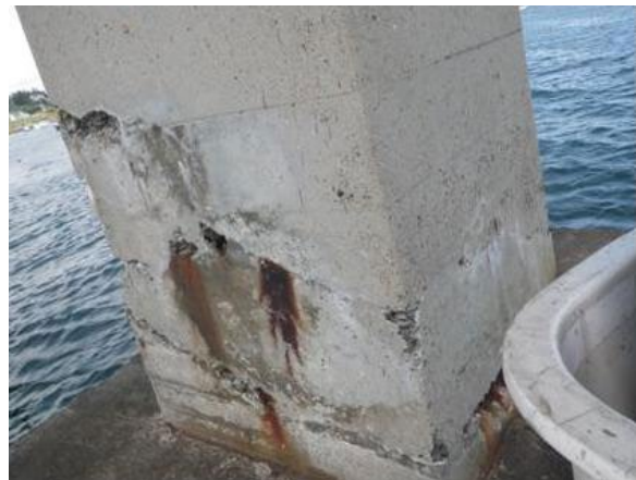
Concrete deterioration and rebar corrosion at base of #9 pier column
