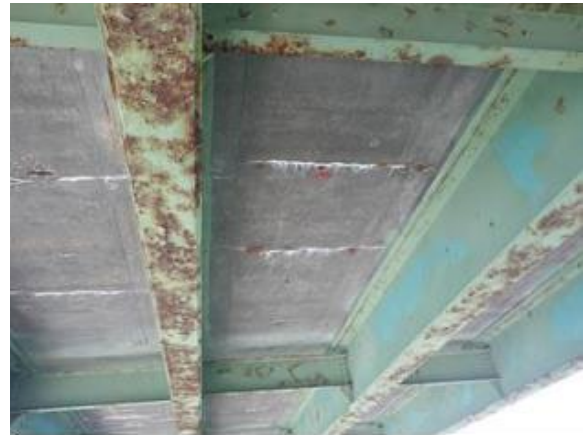
Transverse deck cracking with efflorescence
