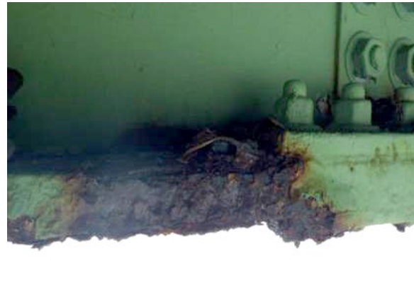
Corrosion and pitting at splice connection
