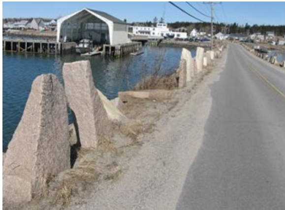
Missing guard stones on Jonesport approach. United States Coast Guard Station in background (looking northerly from bridge).
