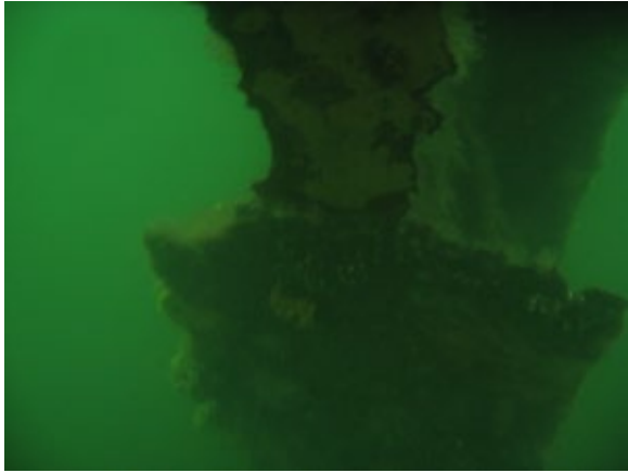
Typical H-Pile section loss at flange
