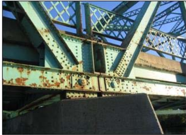
Truss connections - Upstream side
