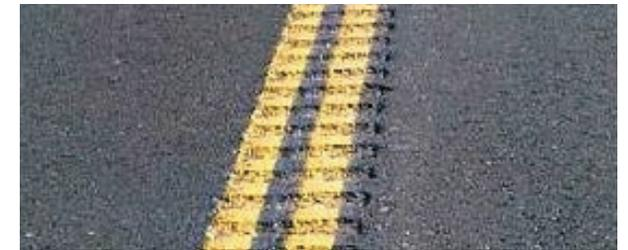
Maine rumble strips will be selectively installed on roads with speed limits of 45 mph or greater. Skips in the rumble strip pattern facilitate motorcycle lane changes.
