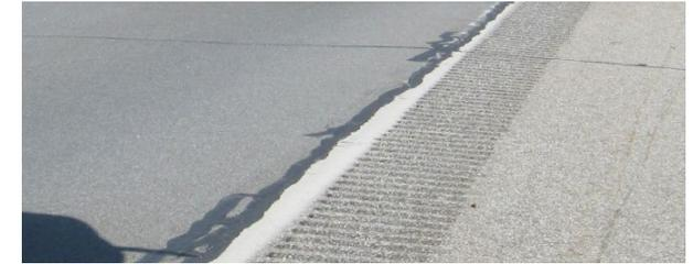
**Centerline rumble strips** are the most common treatment installed on Maine's two-lane roads. They are designed to alert drivers who may be heading for a potentially deadly head-on collision.
