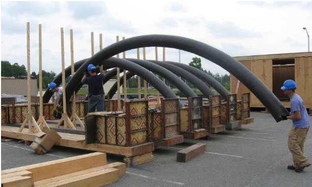
Figure 1. Installation of 22' Span Arch Tubes by Three Laborers
