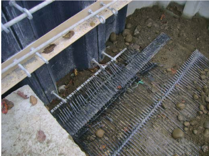
Figure 4 - MSE Retaining wall
