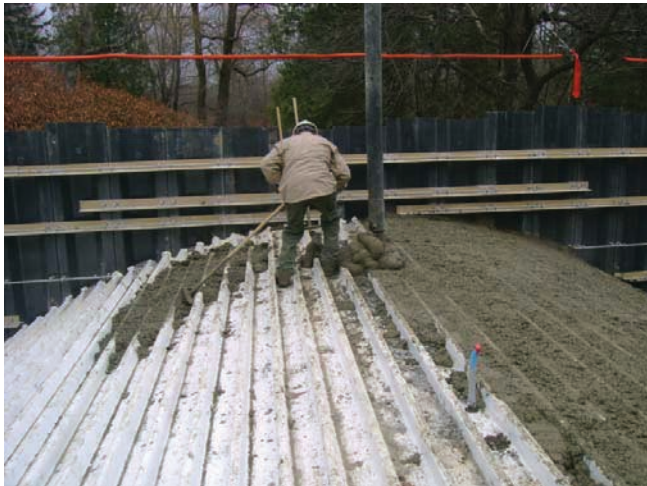
Figure 5 - Concrete placement
