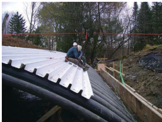
Figure 2 - Installing composite decking
