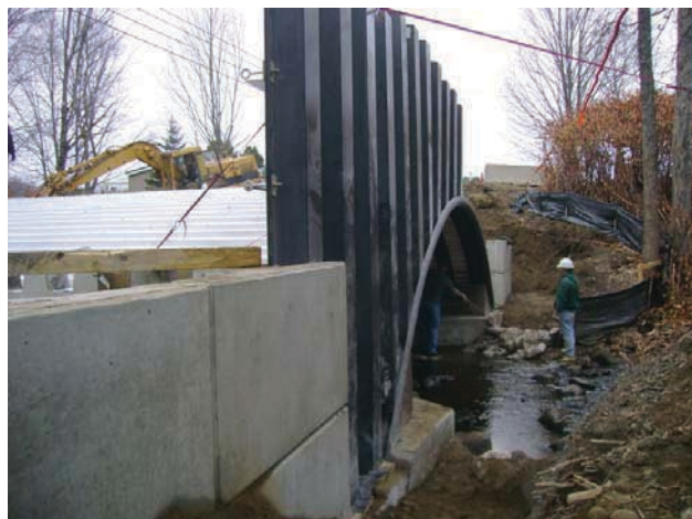
Figure 3 - Installation of composite retaining wall
