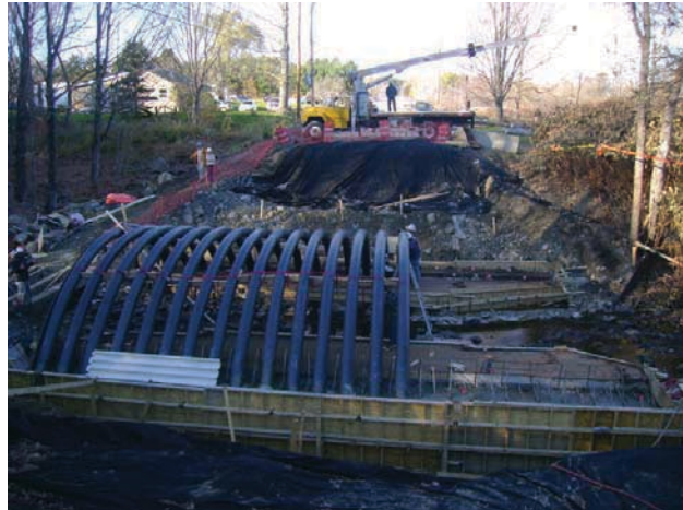
Figure 1 - Installing Composite Arches
