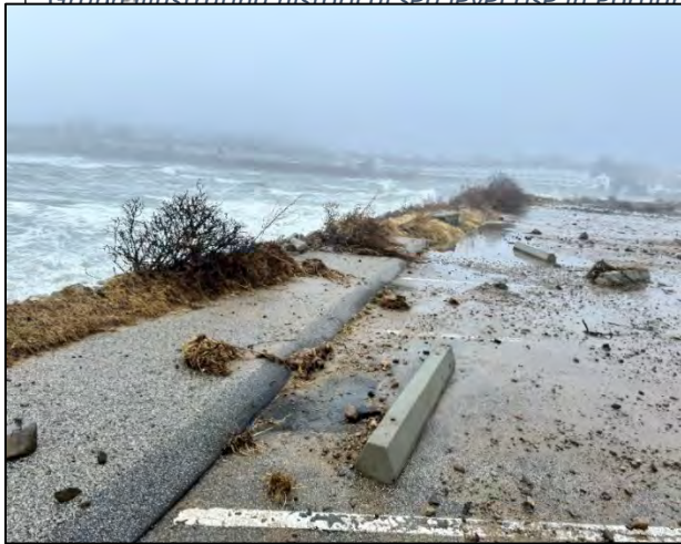
Main Beach Parking Lot 1/24 storm
