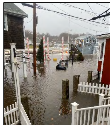
Flooding in Perkins Cove 1/24 storm
