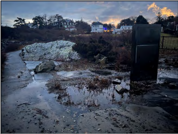
Main beach, Marginal Way, and Perkins Cove flooding after 1/24 storm
