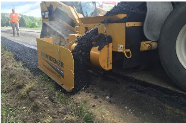
Laying down asphalt using the Road Widener.
