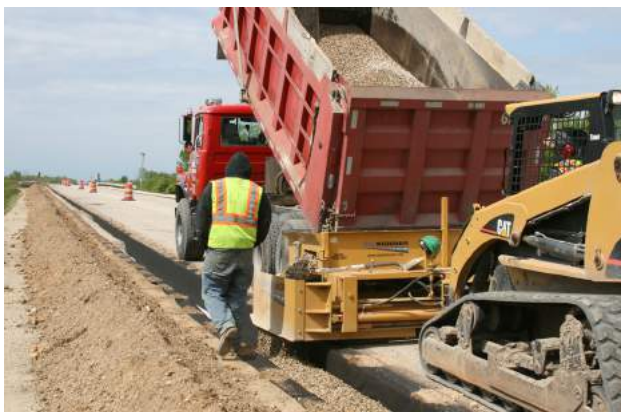
Trenching using the Road Widener.
