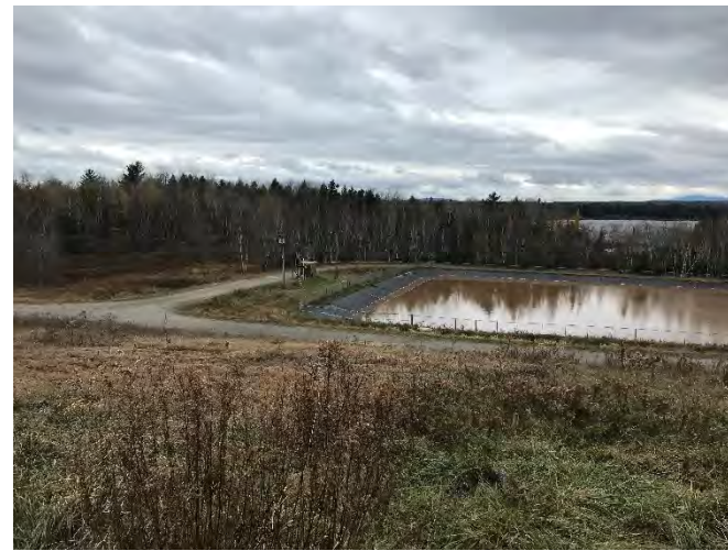
Leachate Pond & Pump Station
