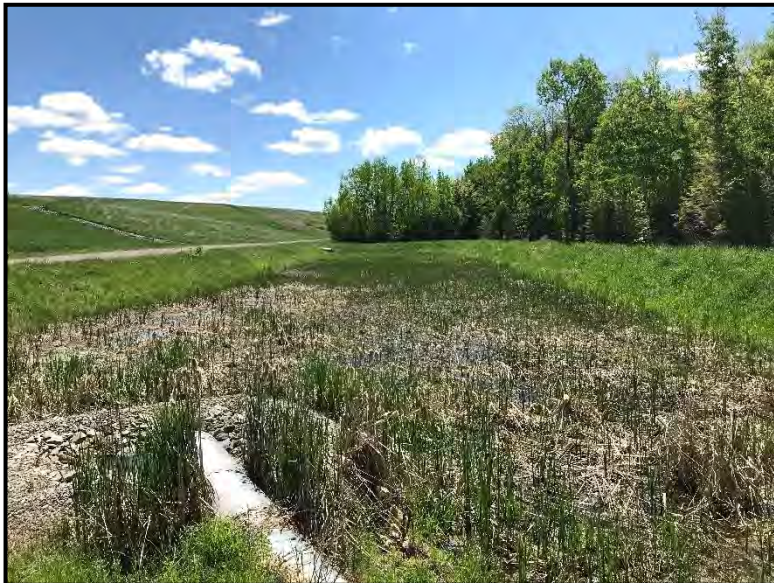
Northwest Sediment Pond (Pond 3)
