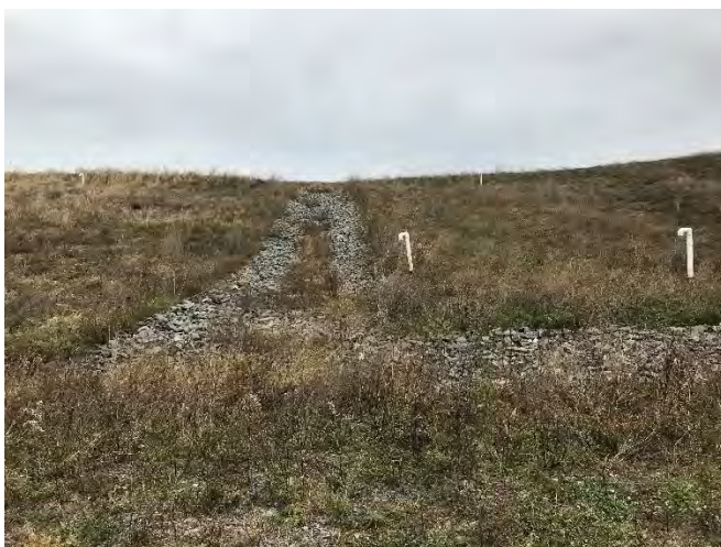
Dolby III Downspout – West Side
