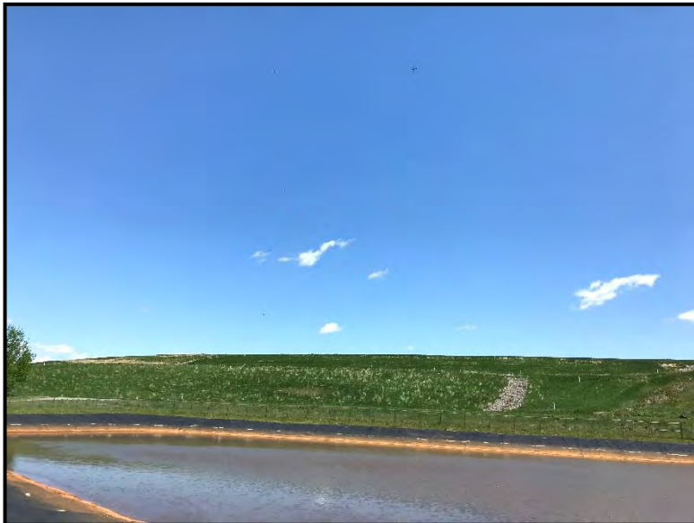
Dolby III West Side and Leachate Pond
