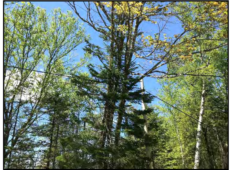
Transition Station Power Line
