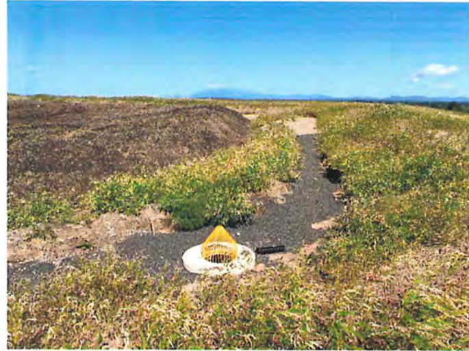
Dolby III Temporary Cell for Lagoon
