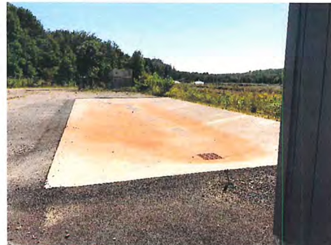
Emergency Leachate Disposal Pad
