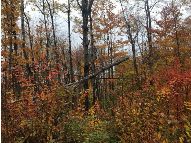
Leachate Pipeline Communications Cable
