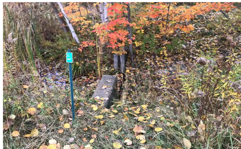
West Sediment Pond Outlet
