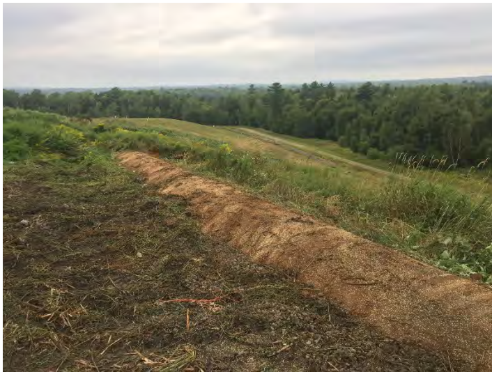
Item 6: Containment berm maintenance
