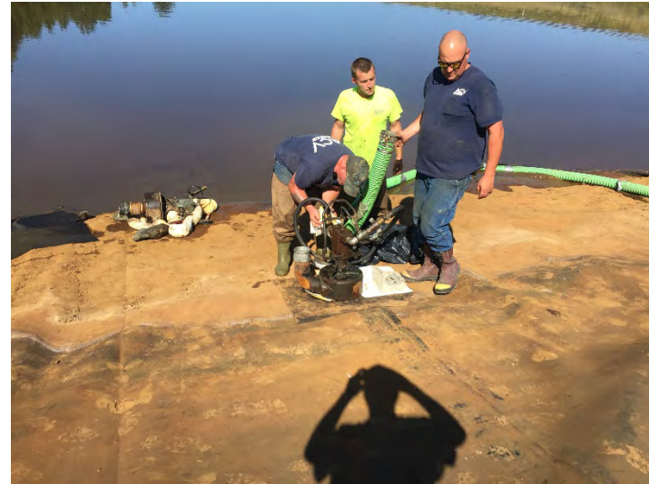
Setting up pump to drain leachate pond
