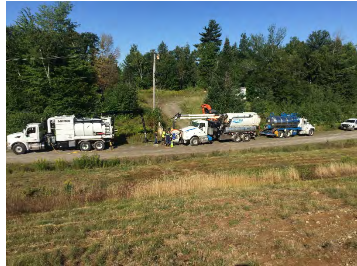
Cleaning at MH-3
