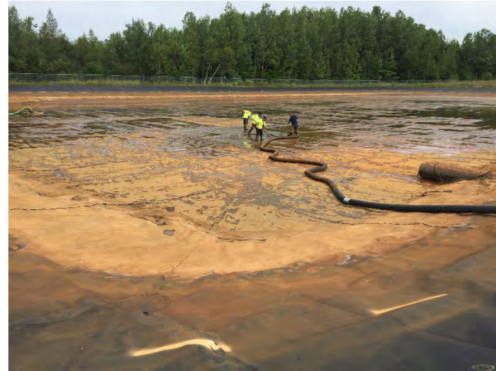
Leachate pond cleaning
