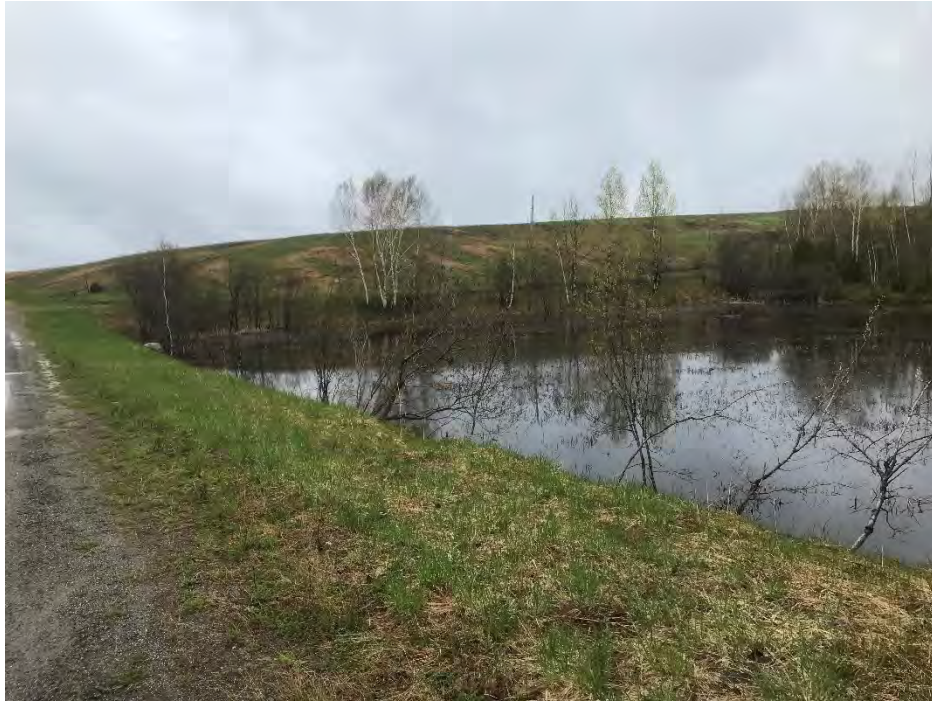
Southwest Sediment Basin
