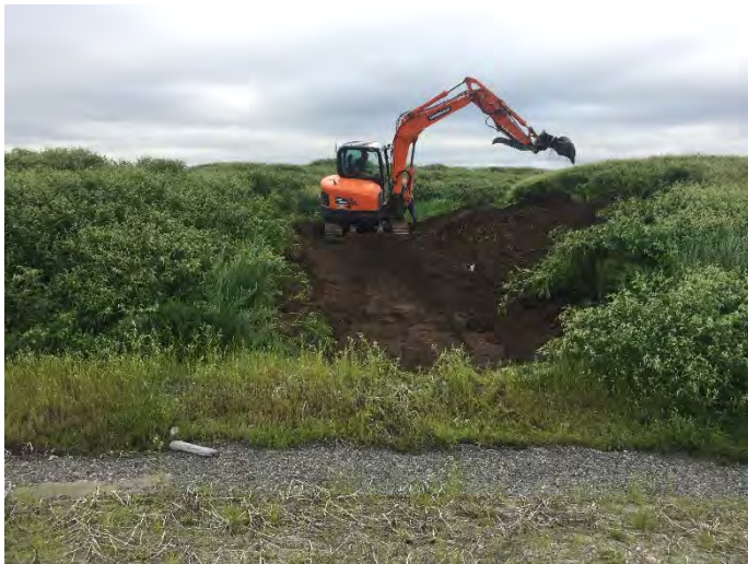
Item 8: Regrade of temporary disposal cell to allow improved drainage
