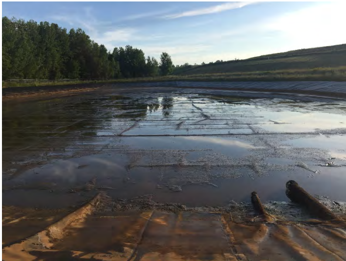
Sediment at leachate pond outlet
