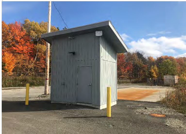
Flow Meter Building
