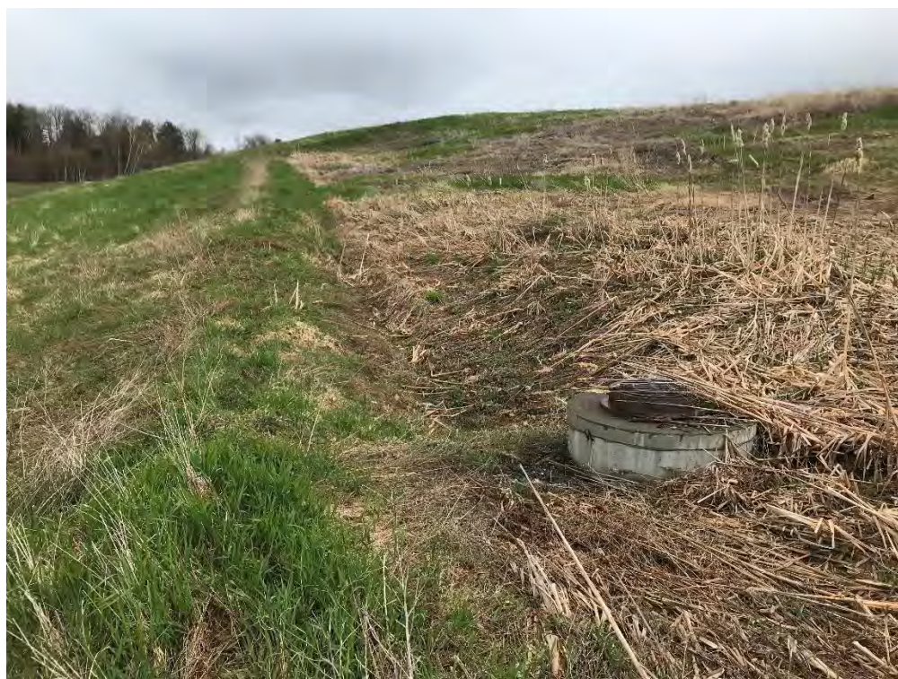
Dolby III North Side Containment Berm (Item 6)
