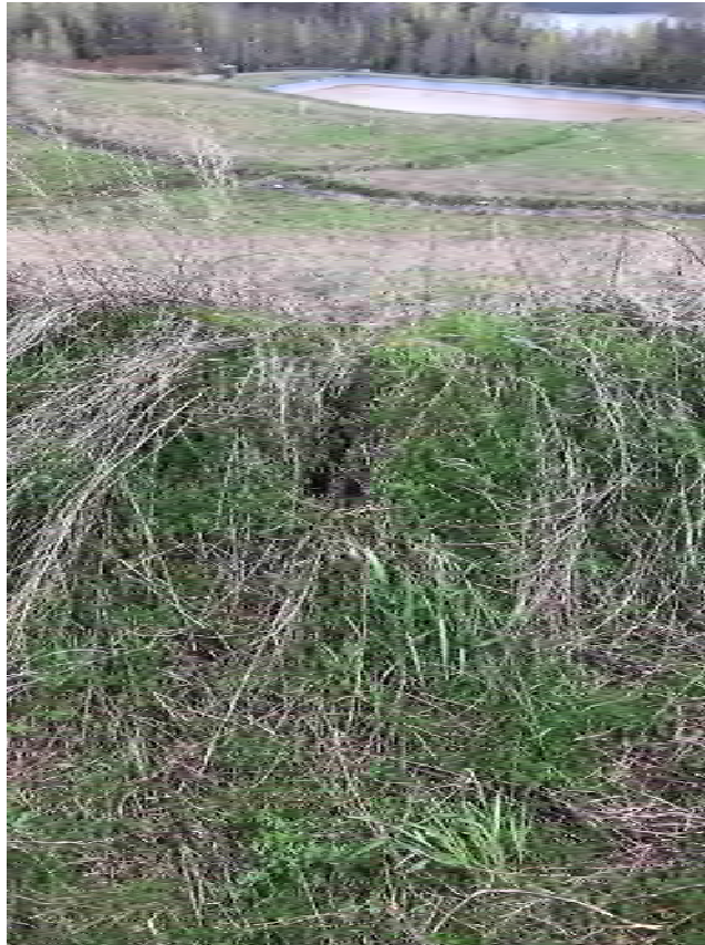
Dolby III Phase 1 Cover Upgrade Erosion Repair (Item 2)
