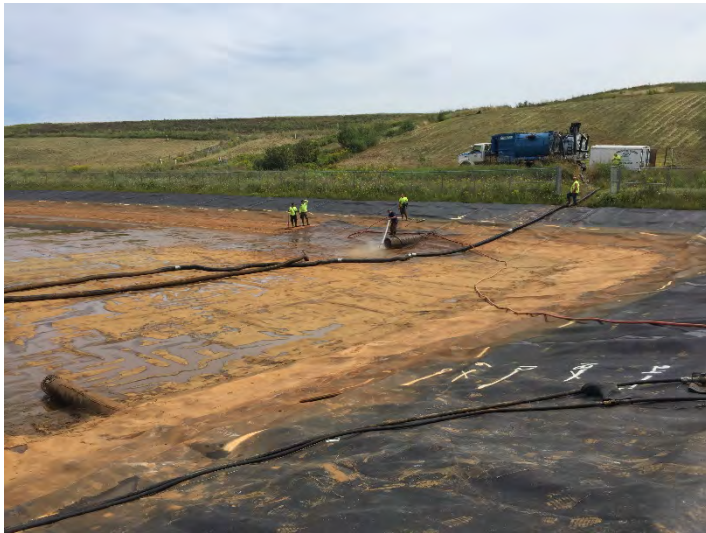
Leachate pond cleaning
