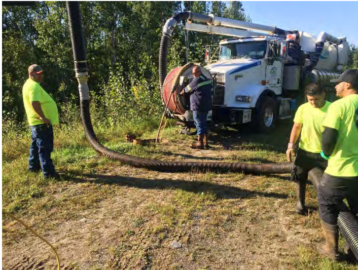
Cleaning from MH-4 to MH-3
