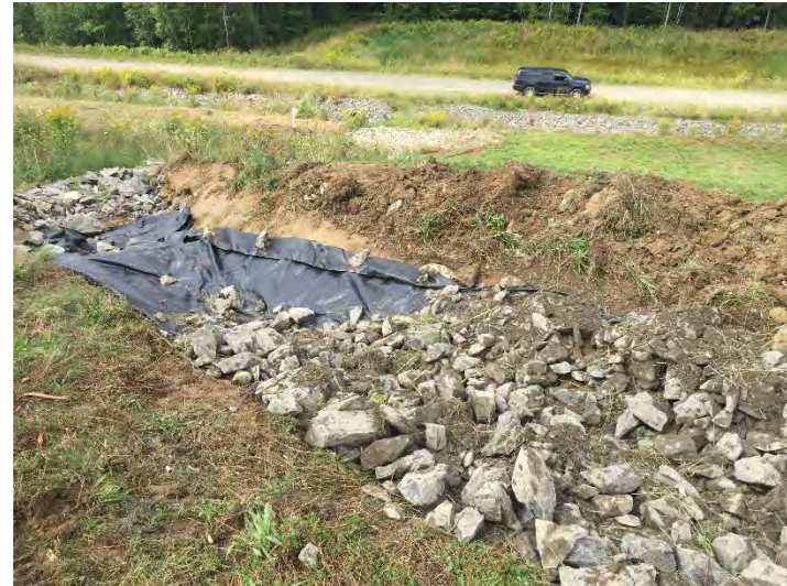
Item 5: Ditch erosion repair
