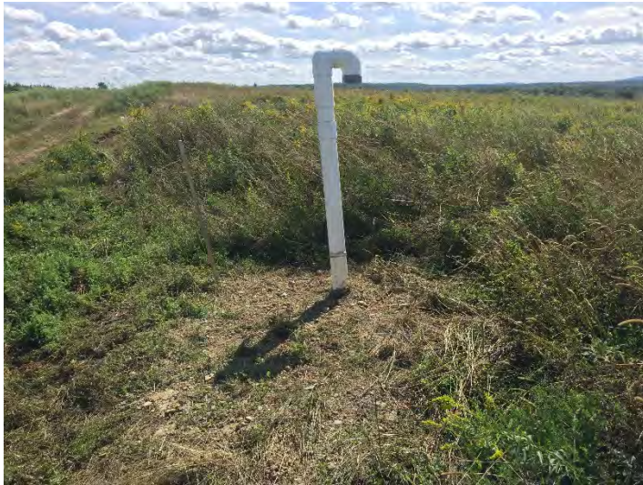
Item 3: Gas vent repair
