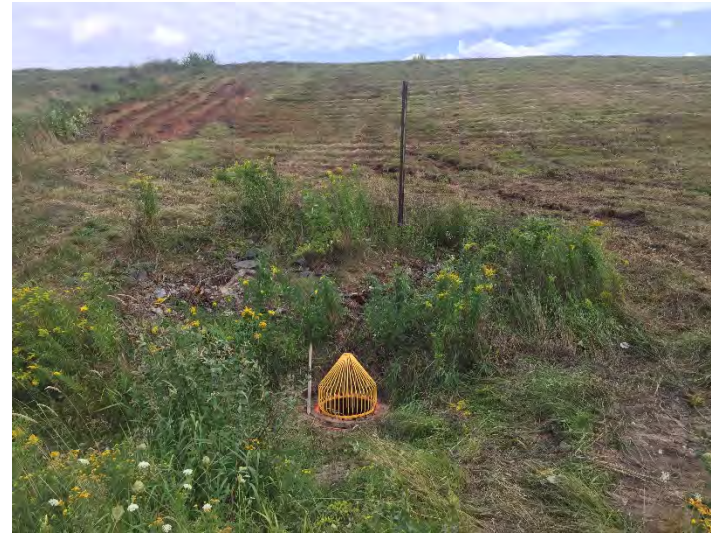
Item 10: Catch basin inlet modification
