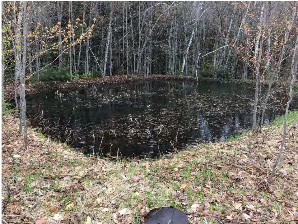
Dolby I Stormwater Basin
