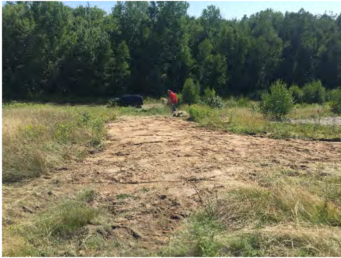
Item 7: Cover soil repair
