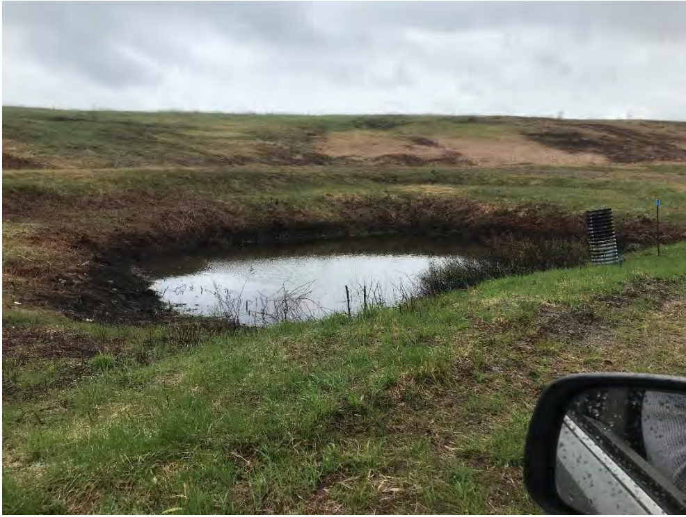
Dolby II Leachate Pond
