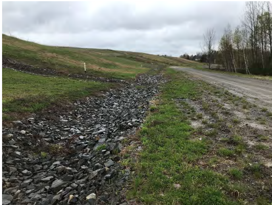
East Side of Dolby III Phase 1 Cover Upgrade
