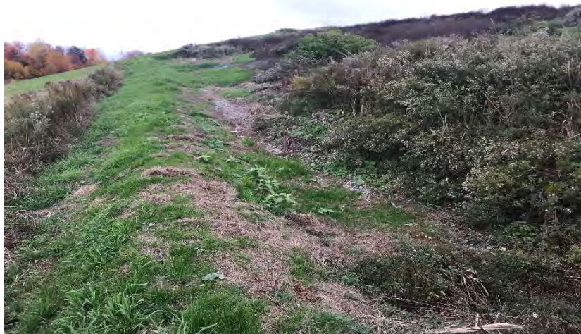
Dolby III 2019 Containment Berm Repair Area
