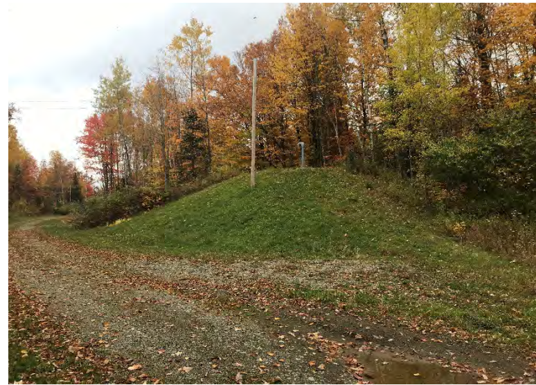
Leachate Pipeline Transition Station
