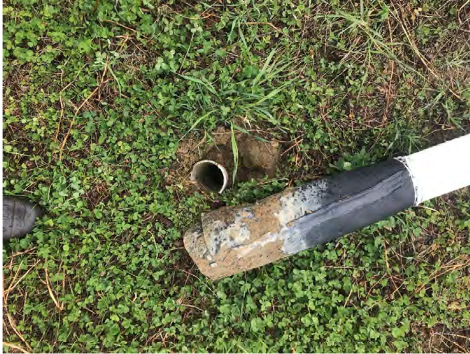
Dolby III Phase 1 Cover Upgrade – Gas Vent (Item 3)
