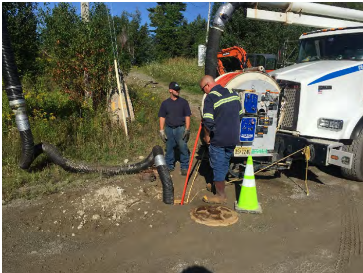
Cleaning from MH-3 to MH-4
