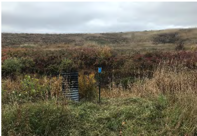
Dolby II Leachate Pond
