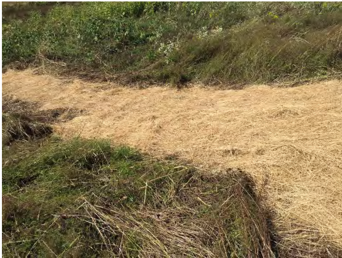
Item 2: Repairing a 60' length of eroded cover soil
