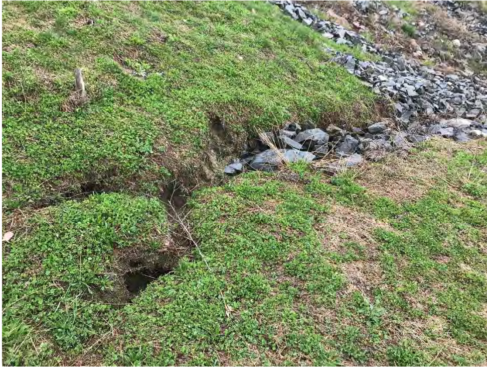
Dolby III Phase 1 Cover Upgrade Erosion Repair (Item 5)
