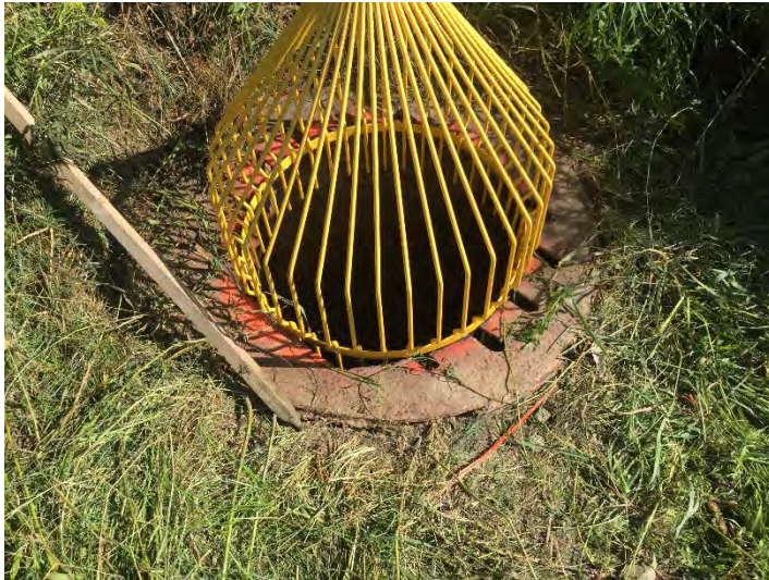
Item 10: Catch basin inlet modification
