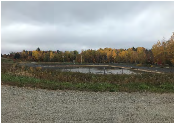
Leachate Pond (looking south)
