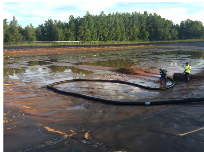
Sediment removal at the leachate pond inlet pipe
