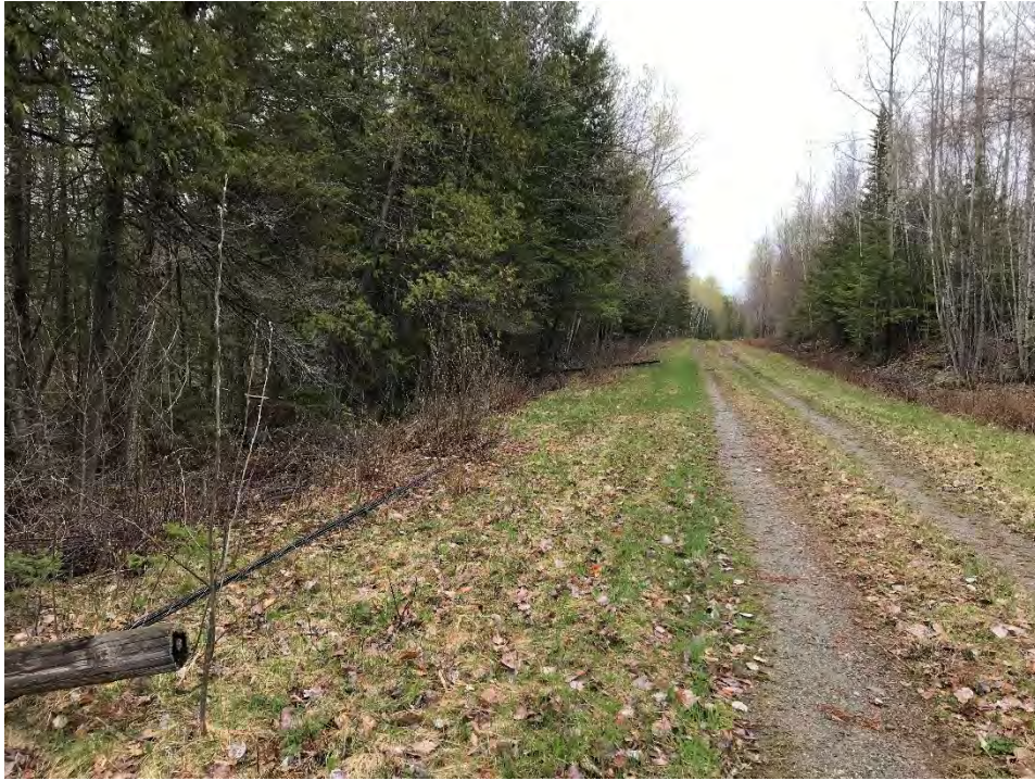
Dolby Leachate Pipeline R.O.W. Utility Line
