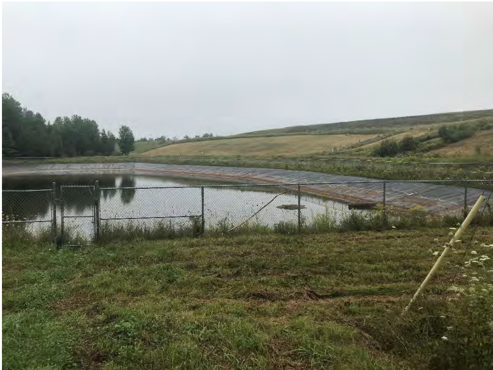
Dolby Leachate Pond
