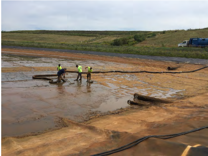
Leachate pond cleaning
