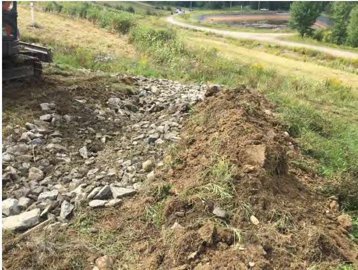
Item 5: Ditch erosion repair
