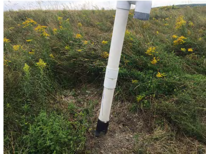
Item 3: Gas vent repair
