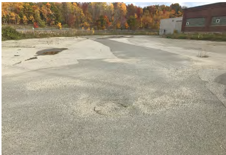
Leachate Manhole at Former GNP Mill Site
