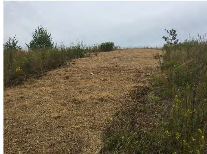
Item 7: Cover soil repair
