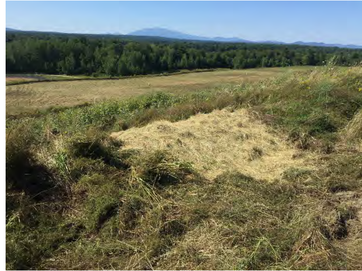
Item 2: Repair of berm that had breached
