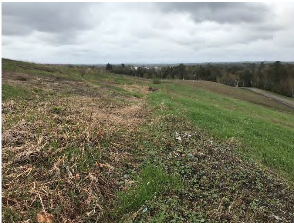
Dolby III North Side Containment Berm (Item 6)
