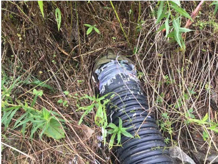
Item 4: Underdrain discharge pipe repair
