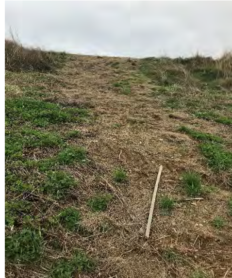
Dolby III 2019 Slope Repair Area
