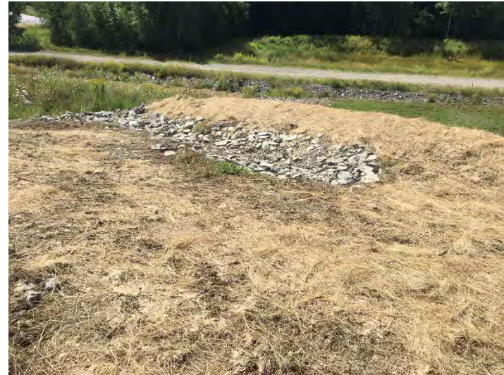
Item 5: Ditch erosion repair
