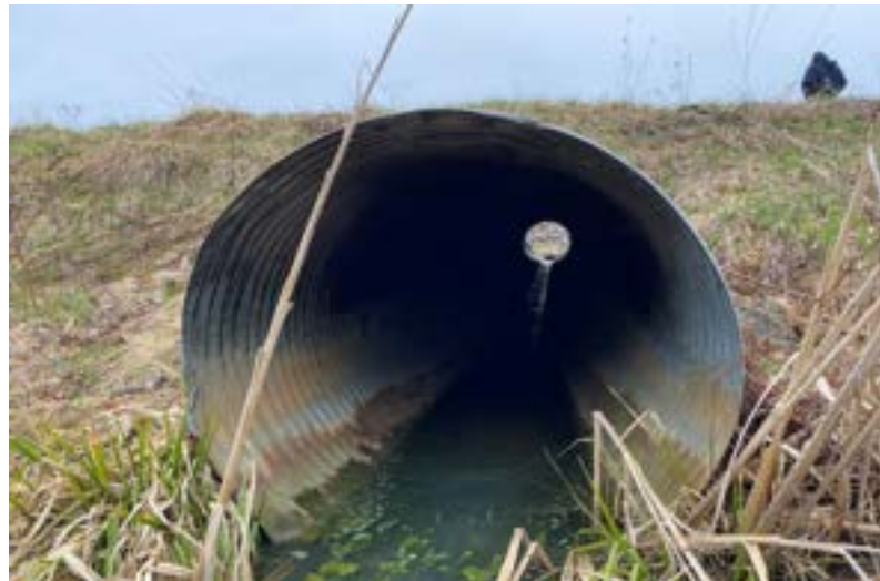
Dolby III Perimeter Access Road Culvert to Northwest Sediment Pond
