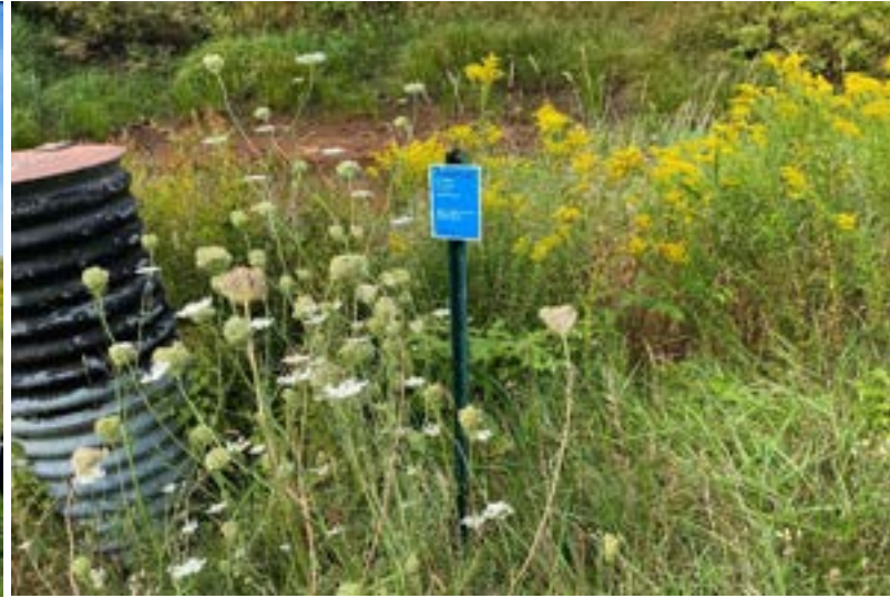
Dolby II Leachate Pond
