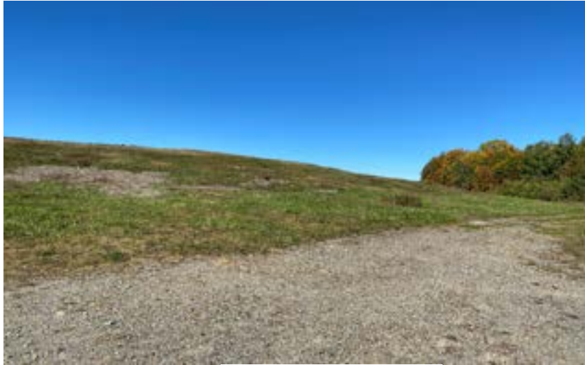
Dolby II Cover Repairs
