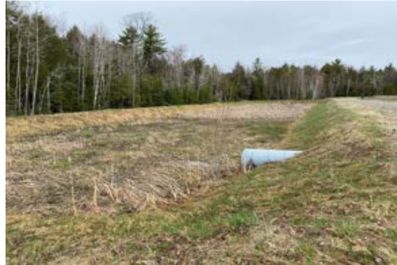
Northwest Sediment Pond
