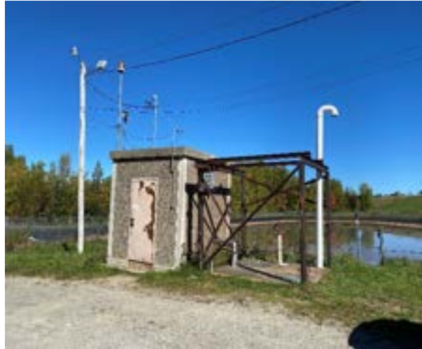
Leachate Pond Pump Station Building
