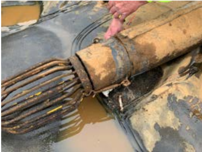
Caulking and steel band removed
