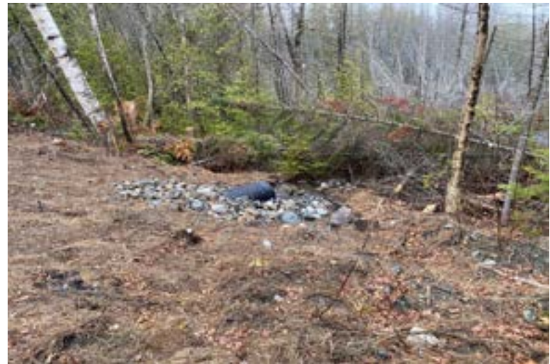
New Culvert Near Leachate Transport Manhole MH-8
