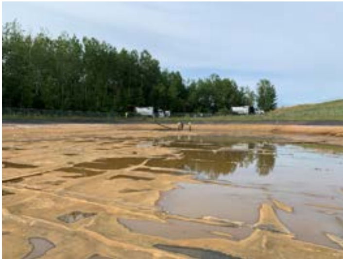
Removing sediment from North end of leachate pond
