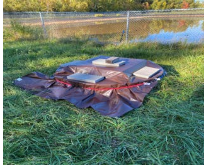
Leachate Pond Leak Detection Manhole Exterior
