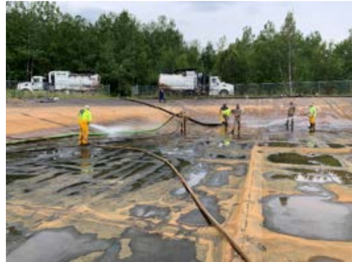
Finishing Pond cleaning at Southwest corner of leachate pond
