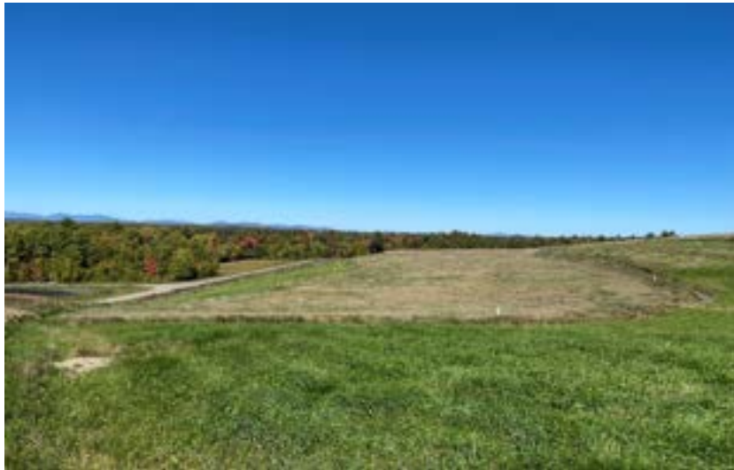
Dolby III Cover Upgrade Area West Side
