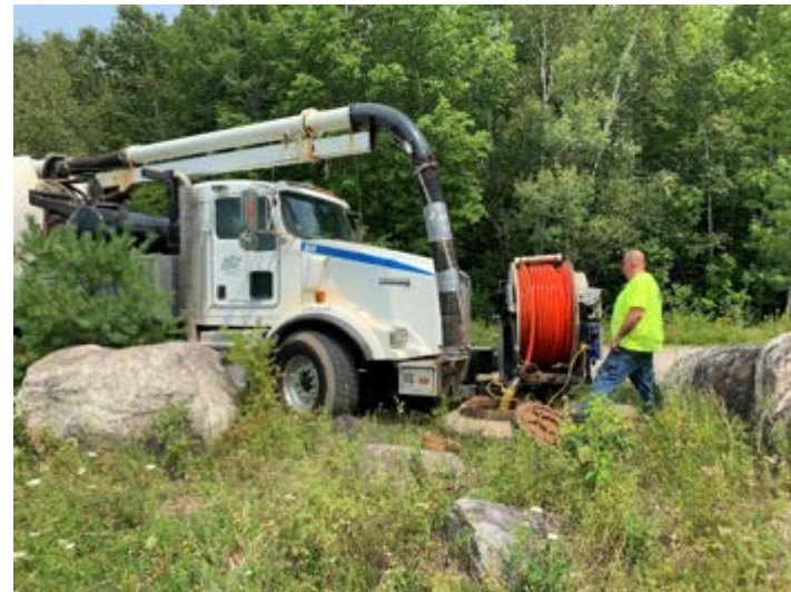
Cleaning at manhole 13
