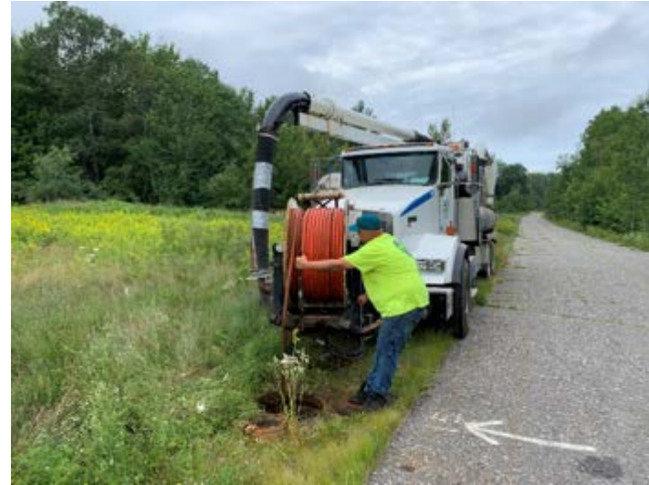
Cleaning at manhole 15
