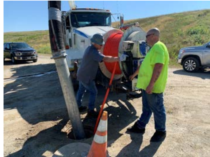
Cleaning at manhole 2
