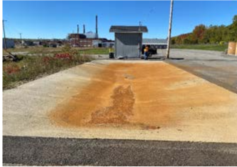
Leachate Transport Pipeline Emergency Leachate Disposal Pad
