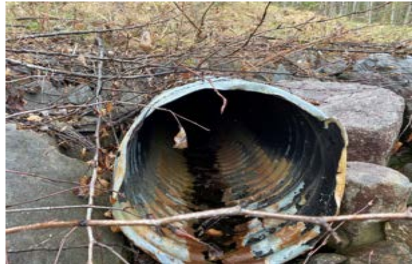
Leachate Pond Perimeter Access Road Culvert at Southwest Corner of Pond
