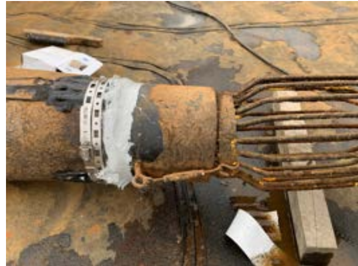
New steel bands and caulking
