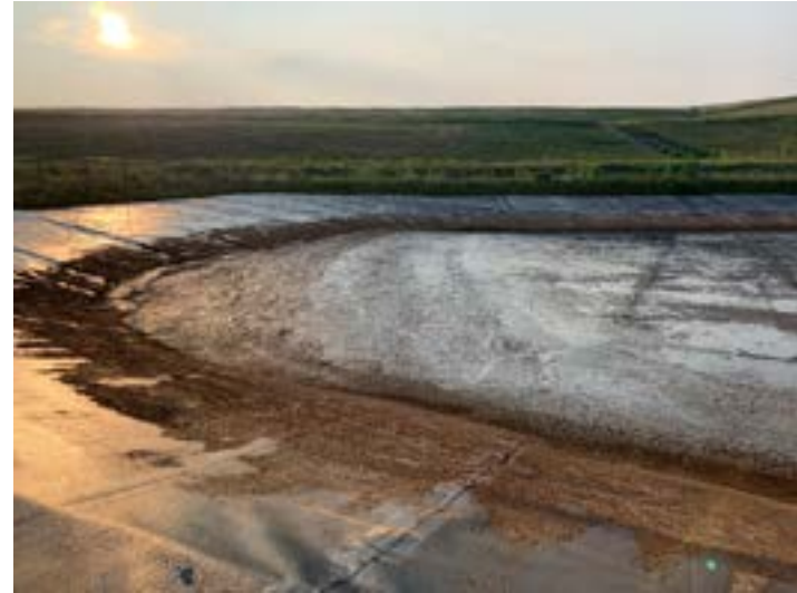
Sediment accumulation at North end of leachate pond
