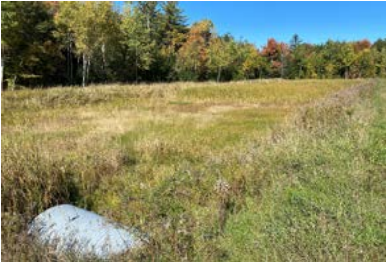
Sediment Pond #3 (Northwest)
