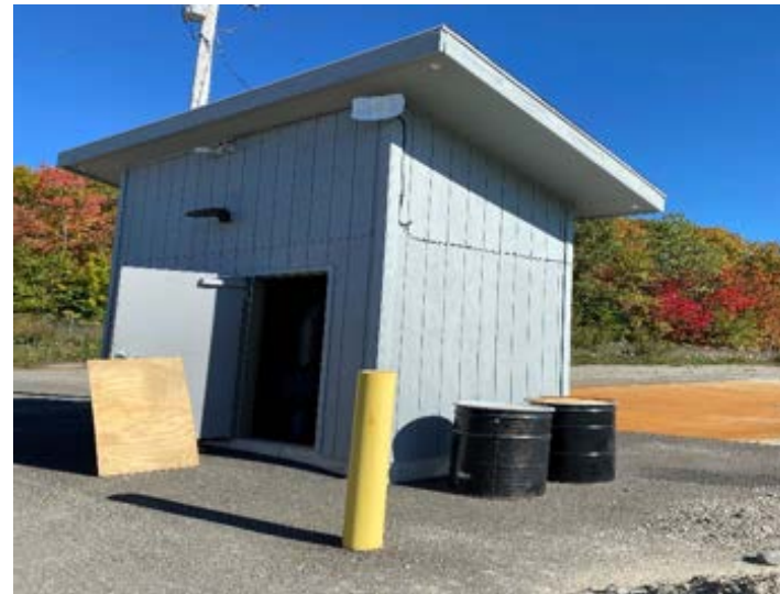
Leachate Transport Pipeline Flow Meter Building Exterior
