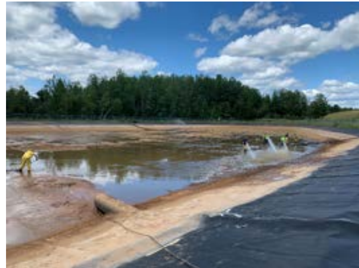
Working from North end towards inlet area
