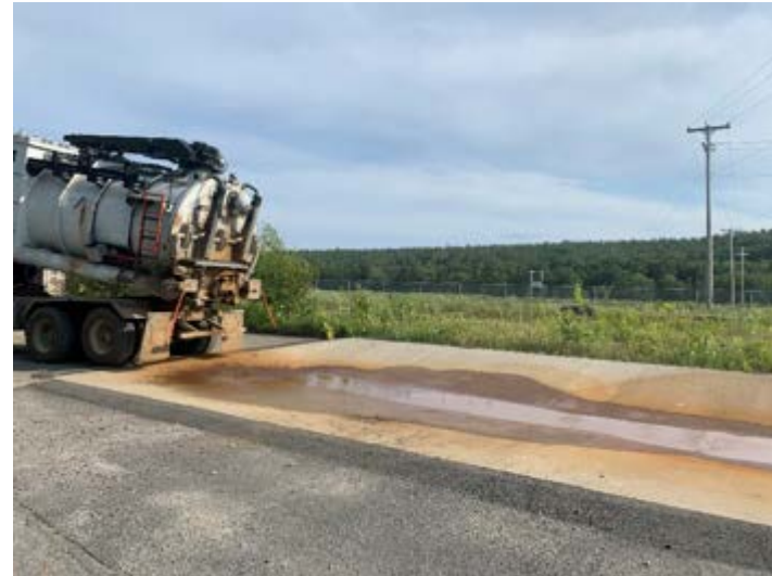
Emptying at emergency disposal pad
