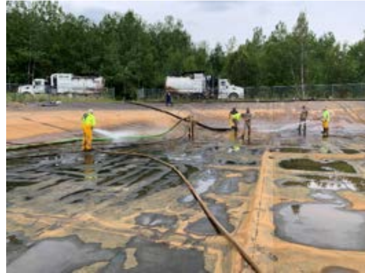
Finishing pond cleaning at Southwest corner
