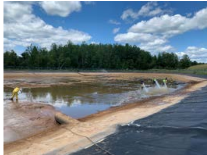
Working from North end towards inlet area
