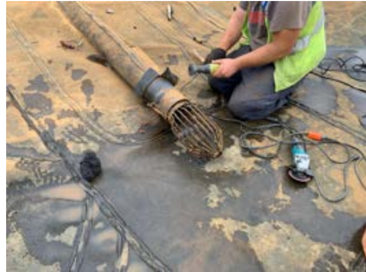
Liner cut and peeled back to install new seal
