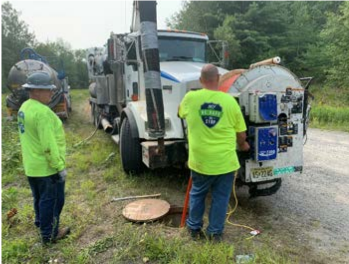
Cleaning at manhole 14
