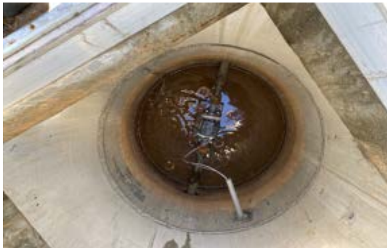
Leachate Pond Leak Detection Flow Meter
