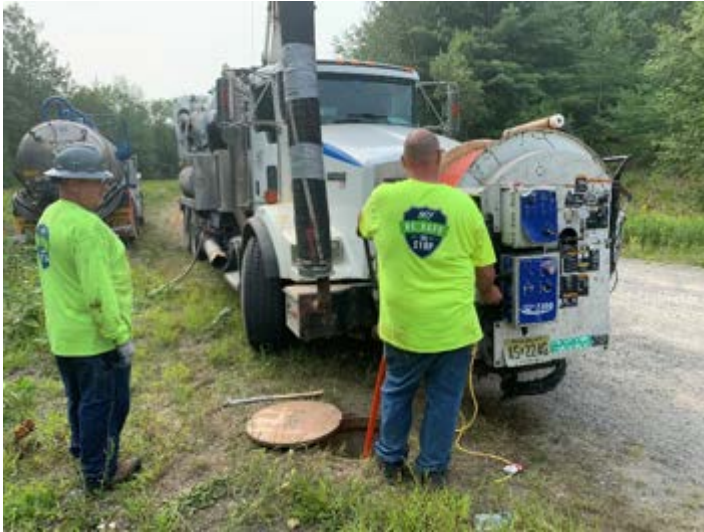
Cleaning at manhole 14
