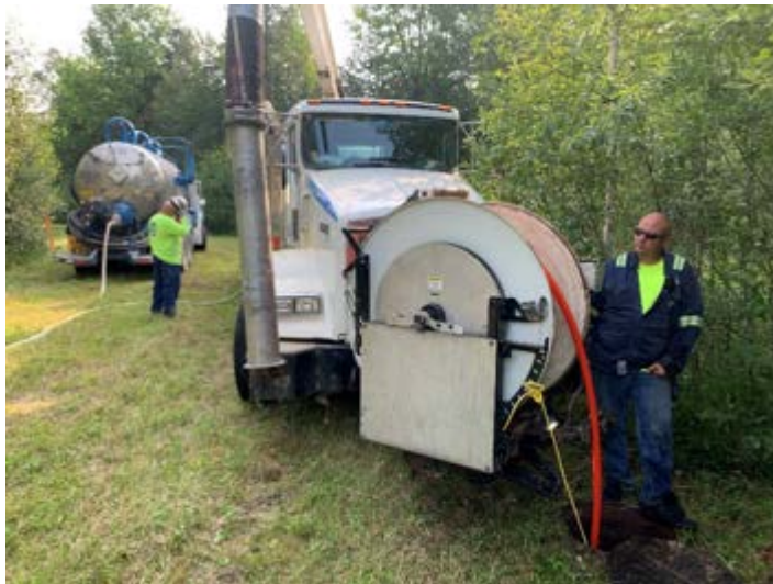
Cleaning at manhole 6
