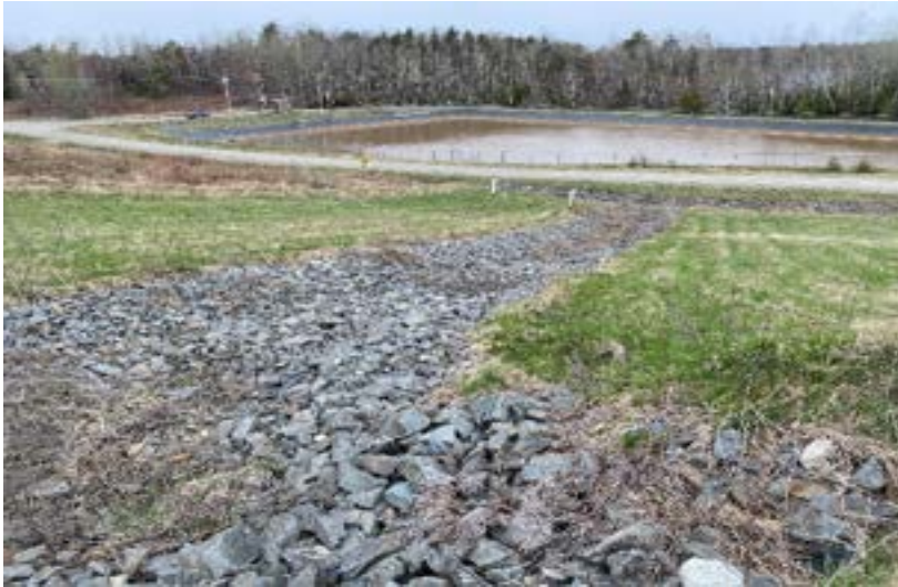
Dolby III West Slope and Leachate Pond
