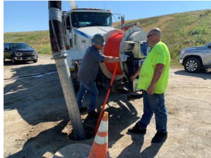
Cleaning at manhole 2
