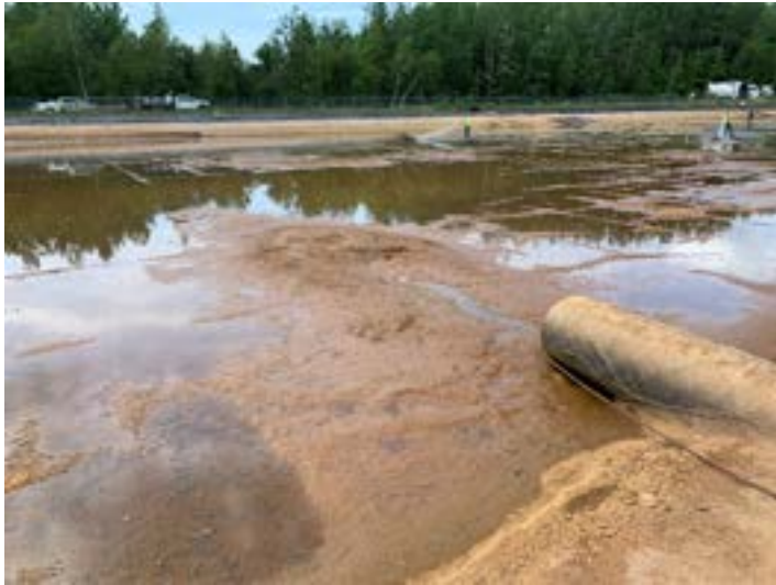
Sediment accumulation at leachate pond inlet pipe
