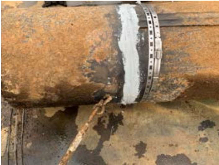
New caulking and steel band on outlet
