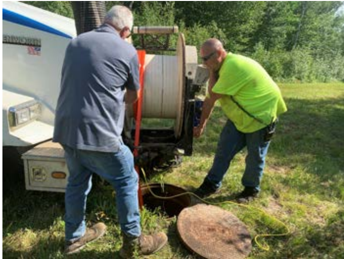
Cleaning at manhole 5
