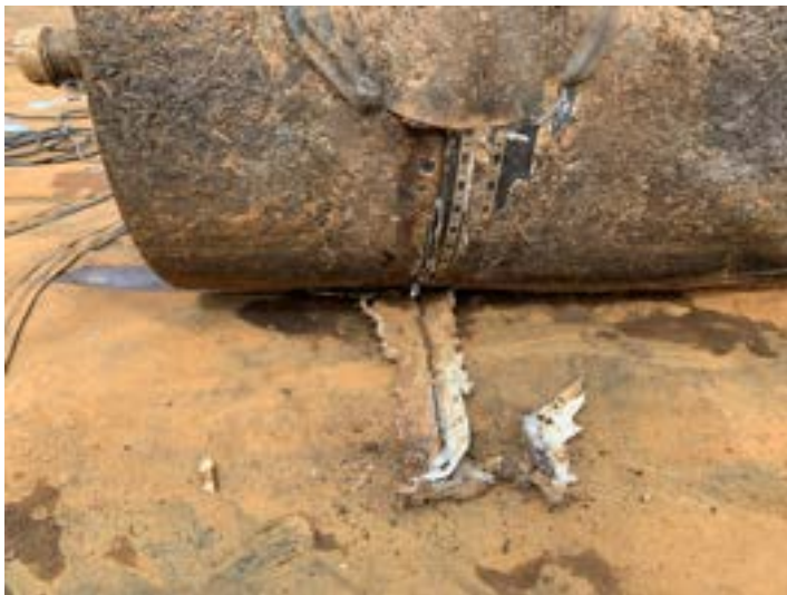
Removing existing caulking
