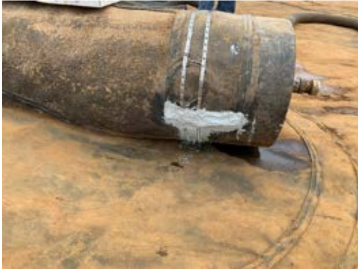
New steel bands and caulking
