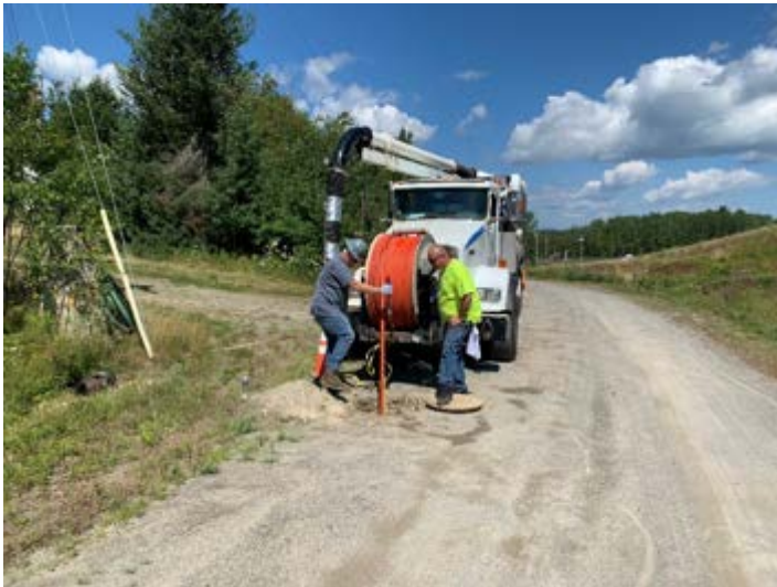
Cleaning at manhole 3
