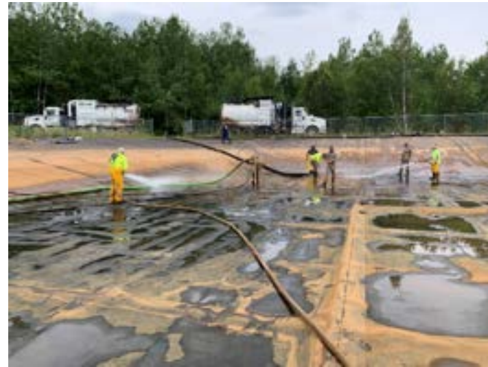
Finishing pond cleaning at Southwest corner
