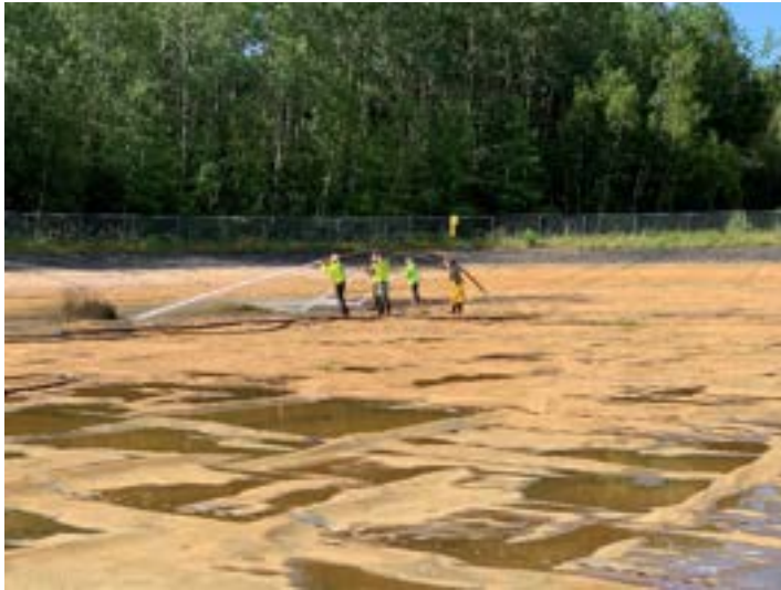
Working from North end down west side
