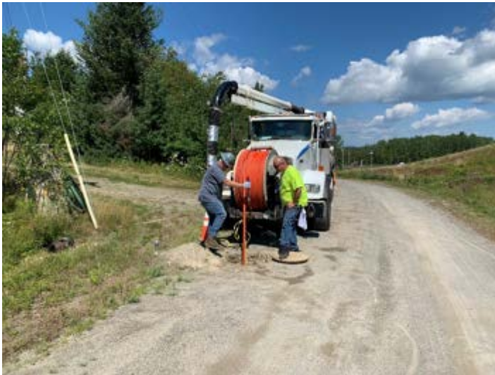
Cleaning at manhole 3
