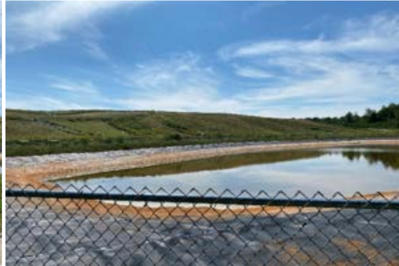
Leachate Pond North End
