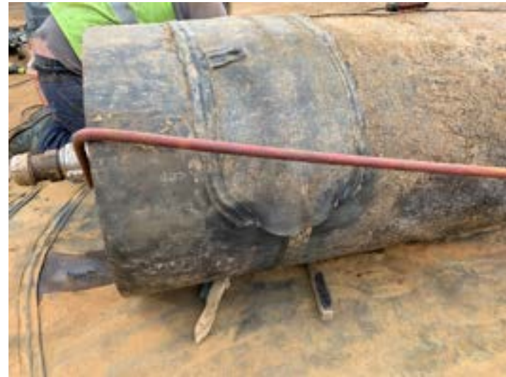
Cleaned inlet pipe and pipe boot
