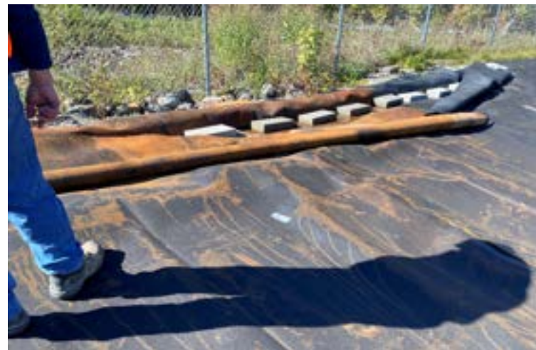
Leachate Pond Emergency Outlet
