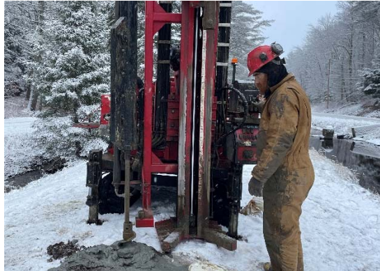
Drilling of Test Boring B-1
