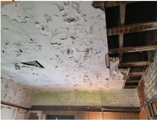
General view of Plaster Ceiling
