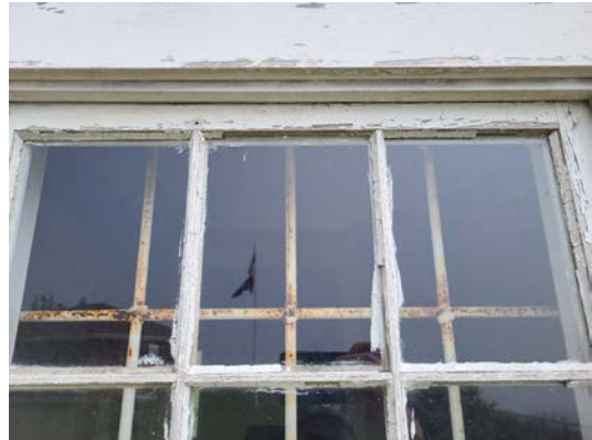
View of window glazing on South Window
