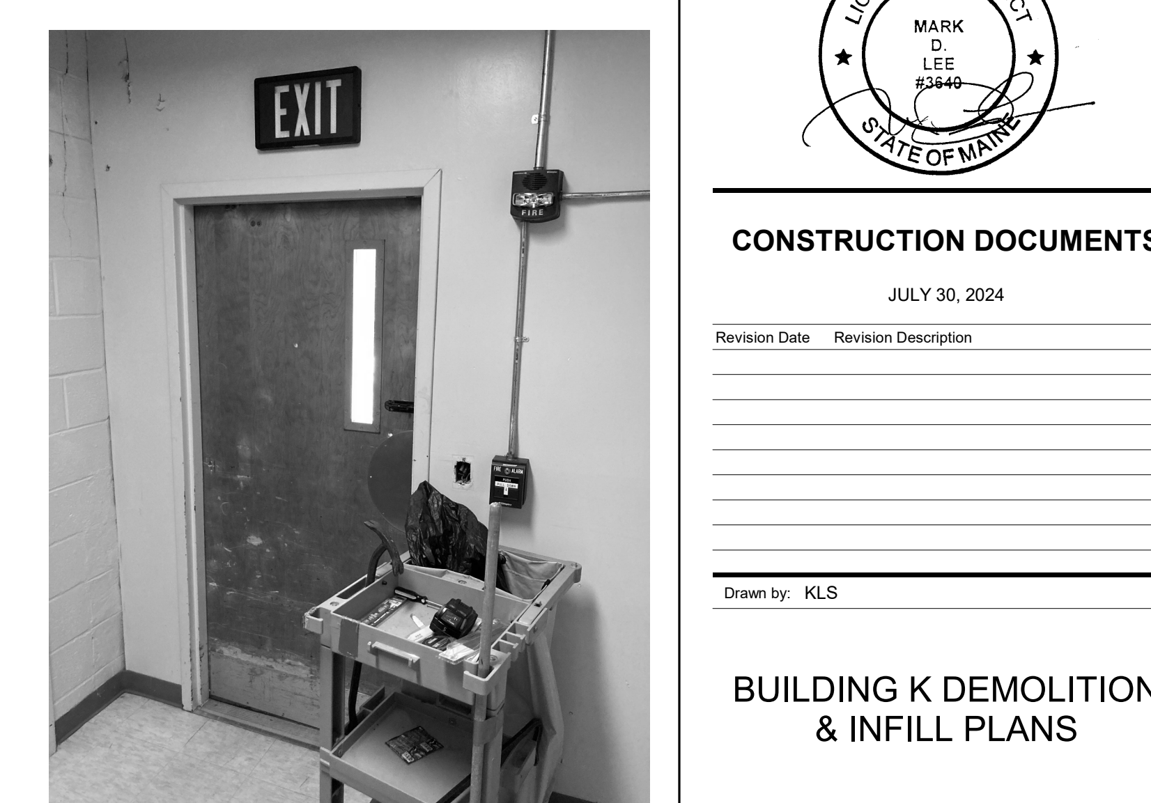
SECOND FLOOR STAIRWELL INTERIOR - CONNECTOR DOOR
