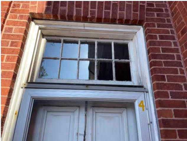
Image 86: View of typical wood transom window above entry door
