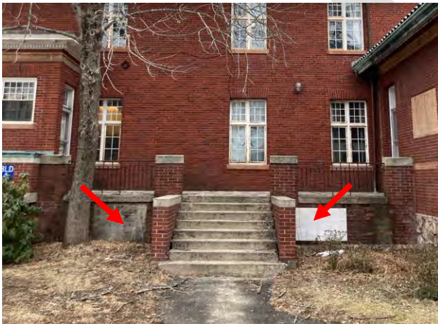
Image 48: Overall view of West entrance, including boarded up basement windows.
