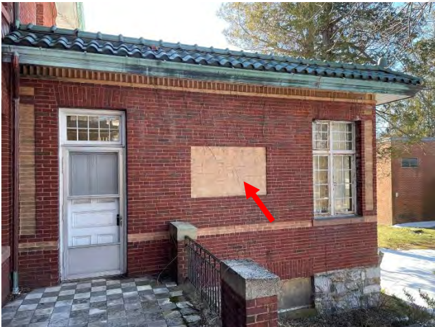
Image 24: Typical view of decorative yellow brick inlay.
