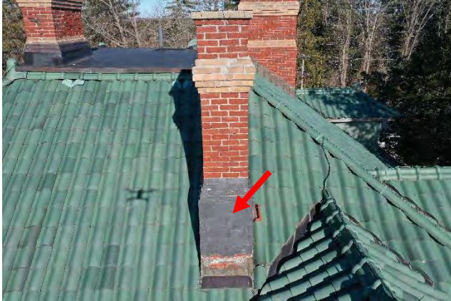
Image 20: View of chimney #4 with bituminous mastic repairs.
