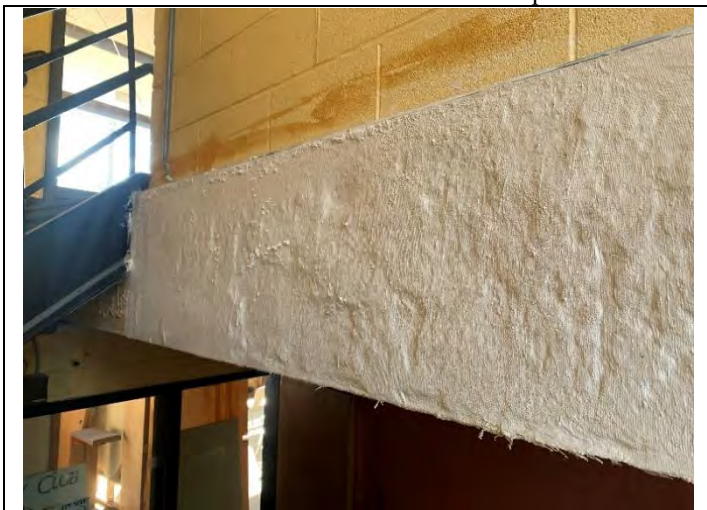
9. Building B, showing HG29 ACM, decorative surfacing
