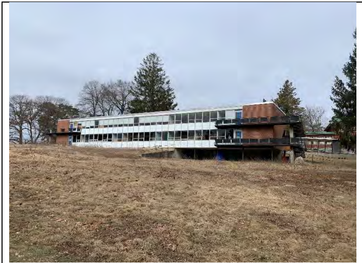
3. Building B Exterior
