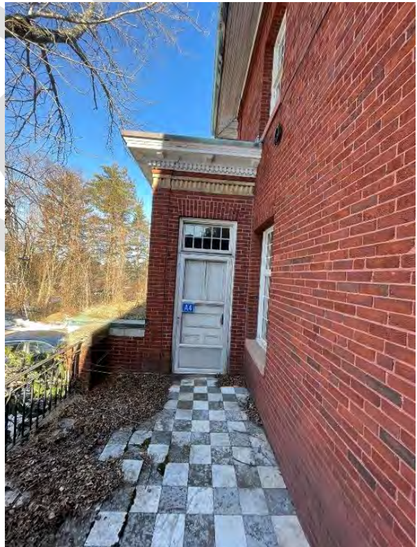
Image 75: View of entryway at West porch.
