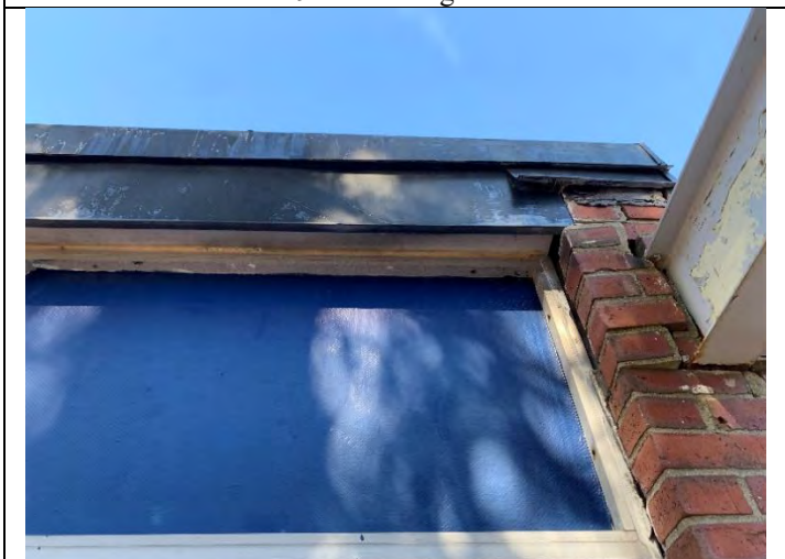
17. ACM Transite Transoms over Fire Doors, Building G, SW Exterior
