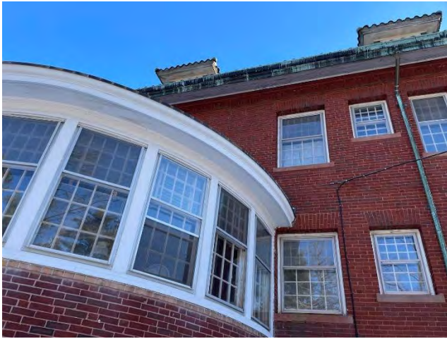
Image 84: View of typical wood framed double hung windows with storm panels.
