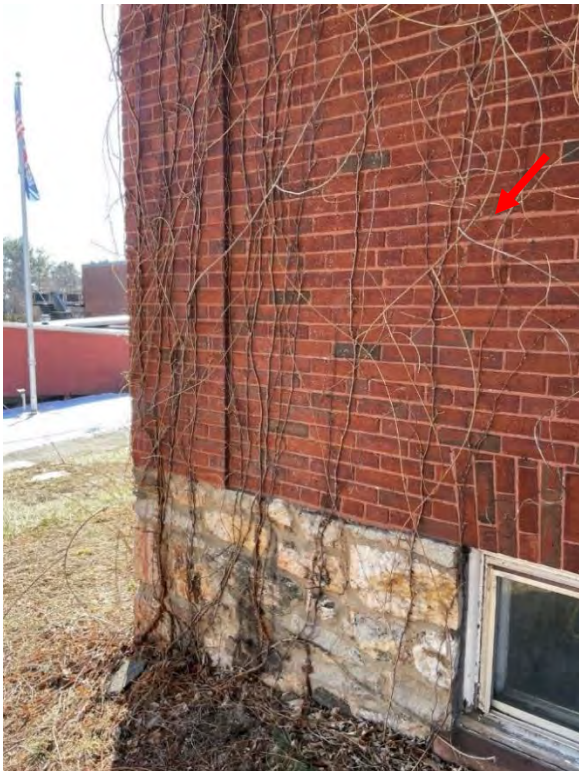
Image 30: View of vines growing against the southeast corner of the foundation.
