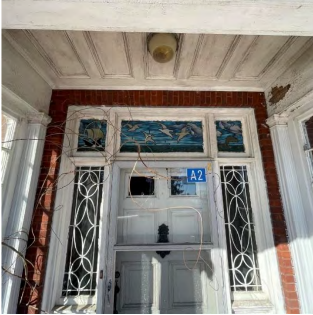
Image 76: View of exterior door at South porch
