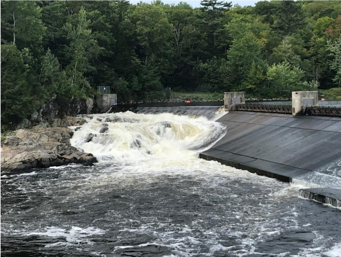
Figure 4.6.1.3.2-2: Bascule Gate No. 5 in Fully Lowered Position
