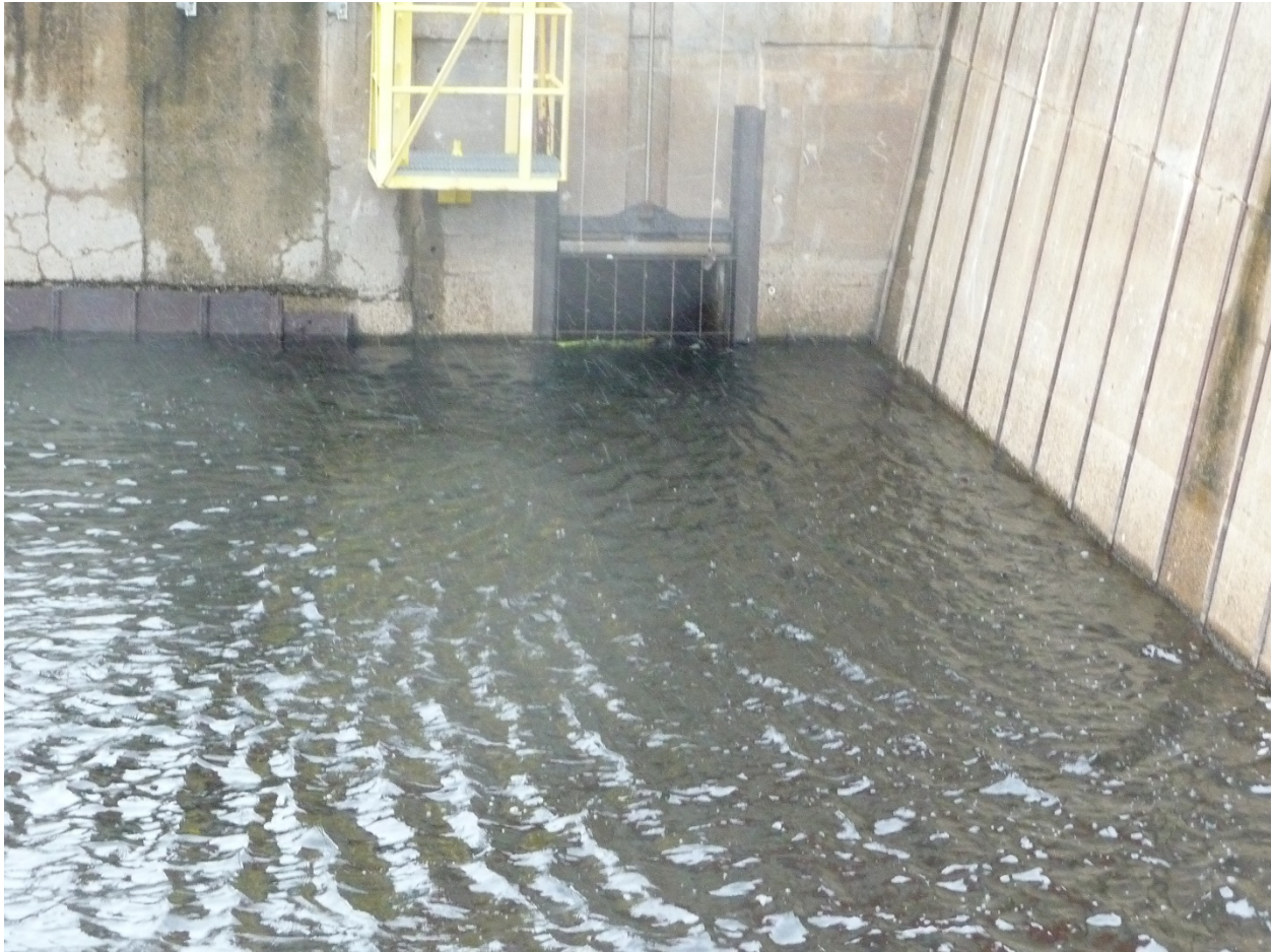
Figure 2.1.3.2-1: Downstream Fish Passage Facility Entry Weir
