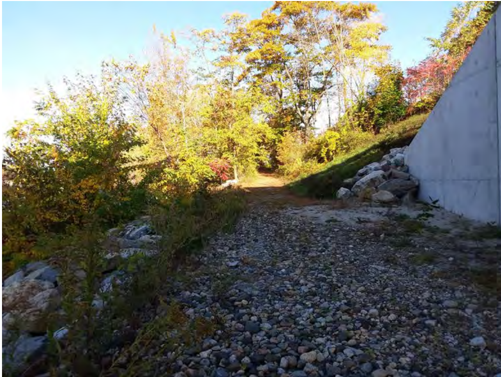
Photo 37: Lisbon Falls Fishing Park, Access Path, Bridge Abutment
