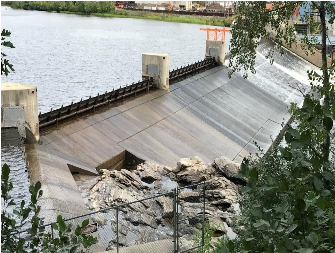
Figure 4.6.1.3.2-4: Exposed Bedrock Area below Bascule Gate No. 5 as Viewed from River Right
