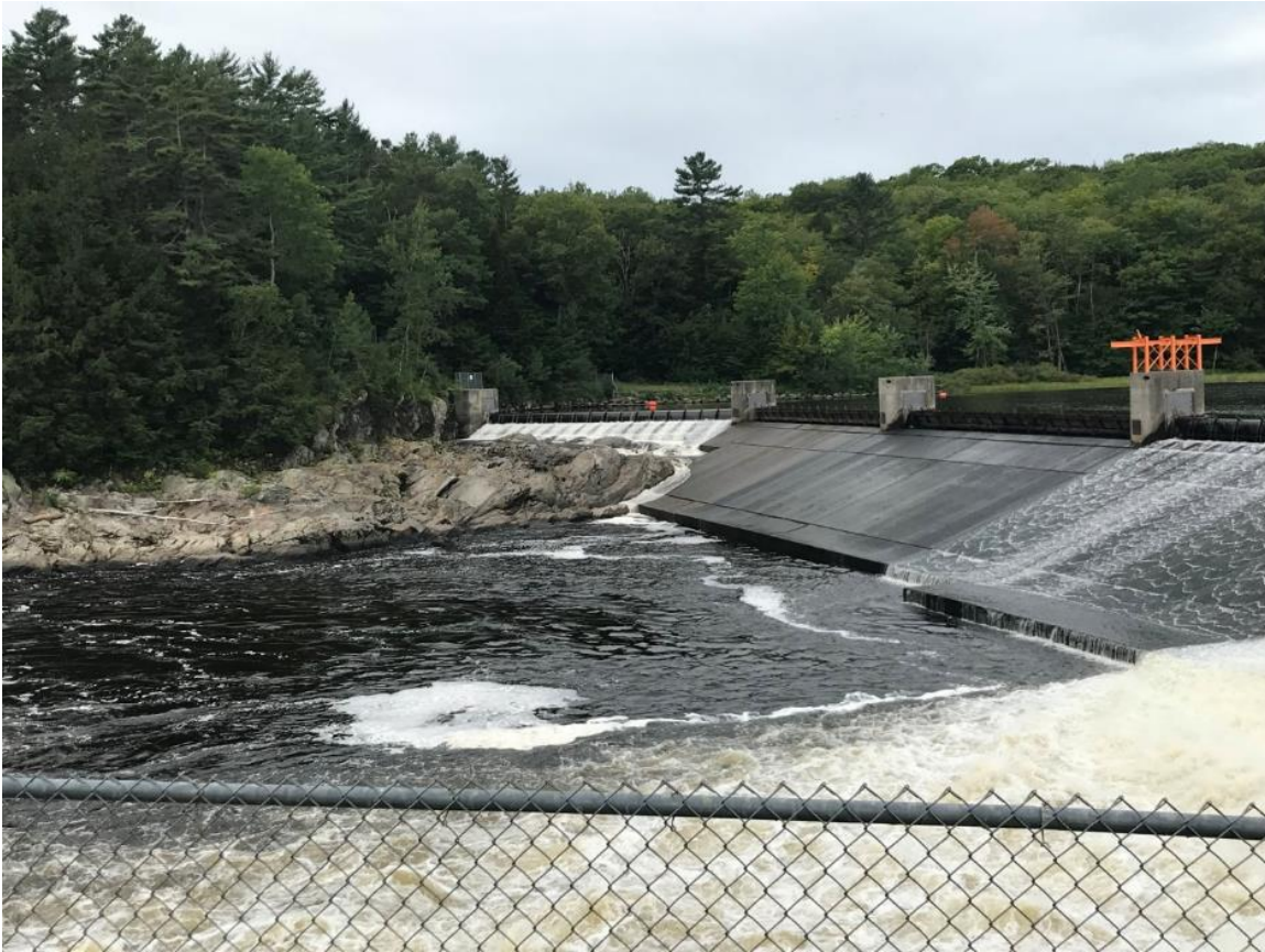
Figure 4.6.1.3.2-1: Initiation of Bascule Gate Operation
