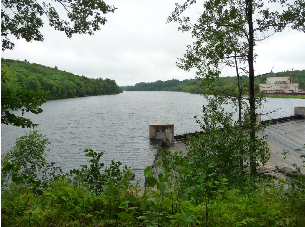
Figure 4.10.1.1-2. View Looking Upstream from Pejepscot Dam
