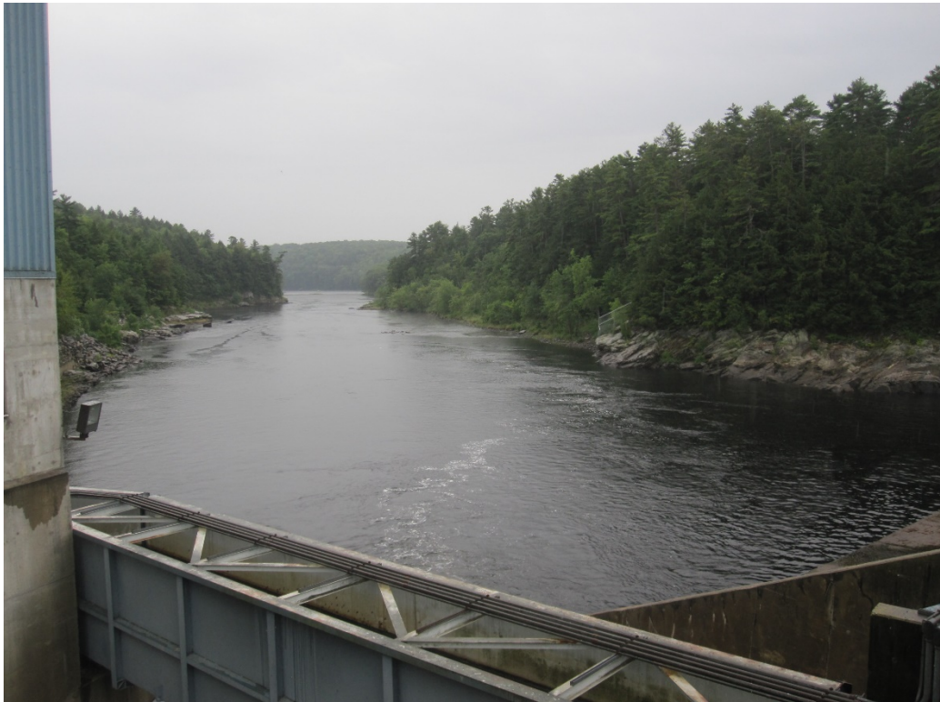
Figure 4.10.1.1-1. View Looking Downstream from Pejepscot Dam
