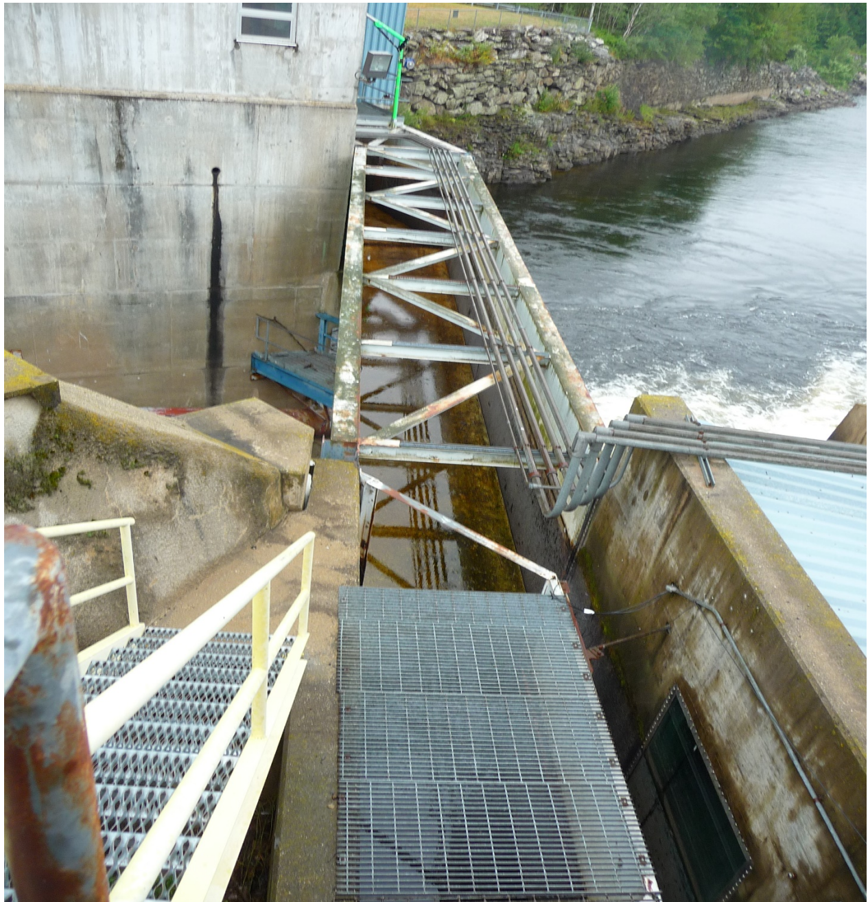
Figure 2.1.3.1-1: Upstream Fish Passage Facility
