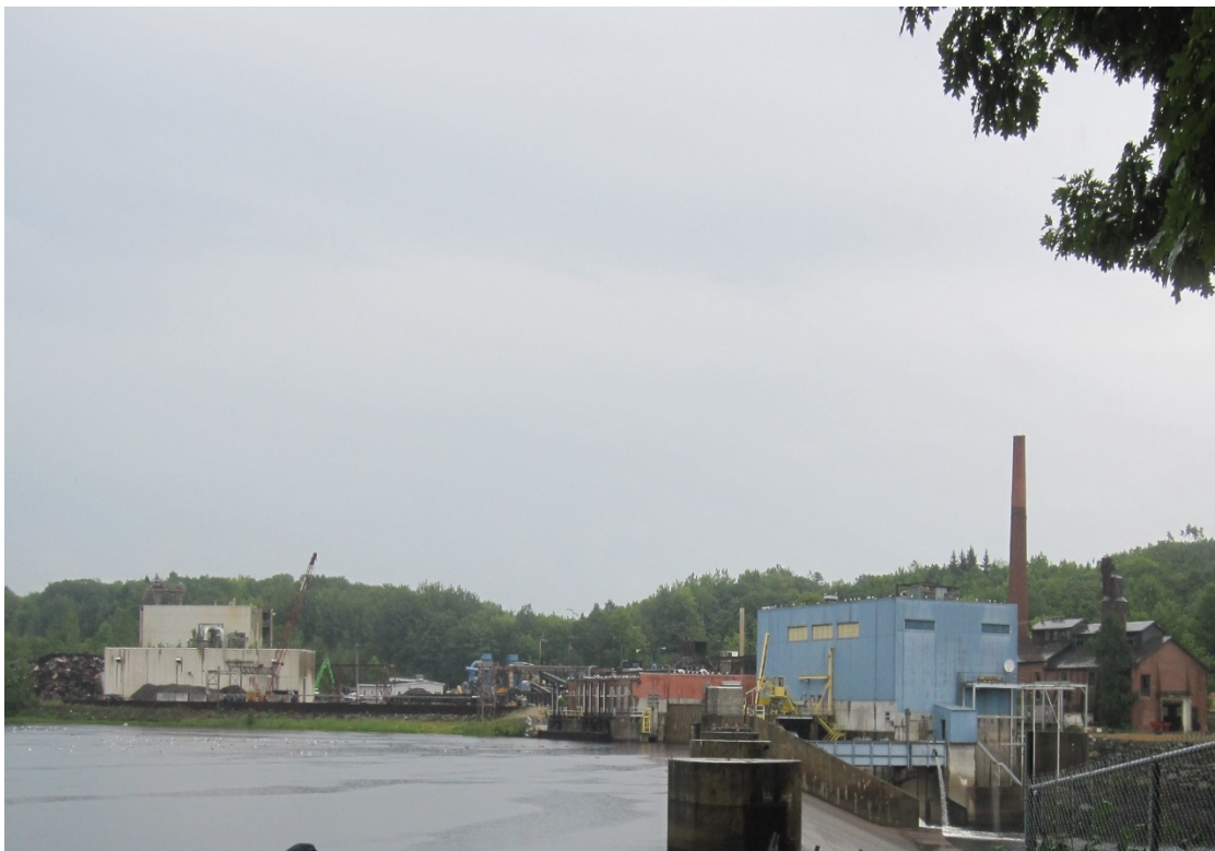
Figure 4.10.1.1-3. View of Powerhouses and Grimm Industries
