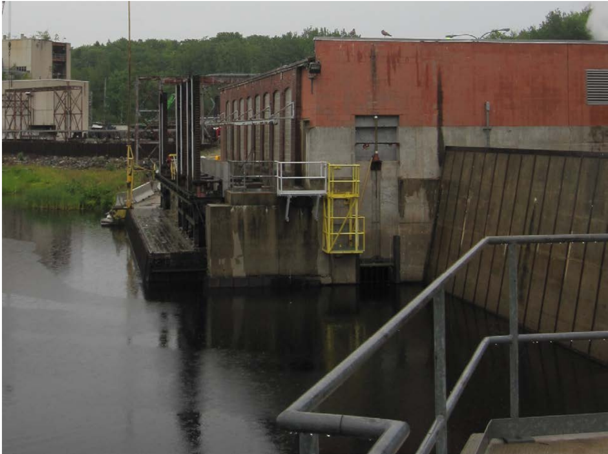
Figure 2.1.2-1: Original Powerhouse and Intake
