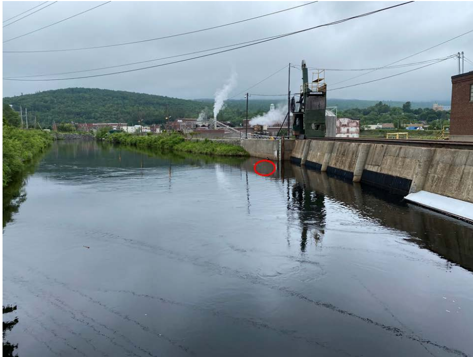
Figure 5. Power canal deployment location for the temperature/DO logger to be considered representative of conditions downstream of the confluence of the bypassed reach and lower powerhouse discharge.
