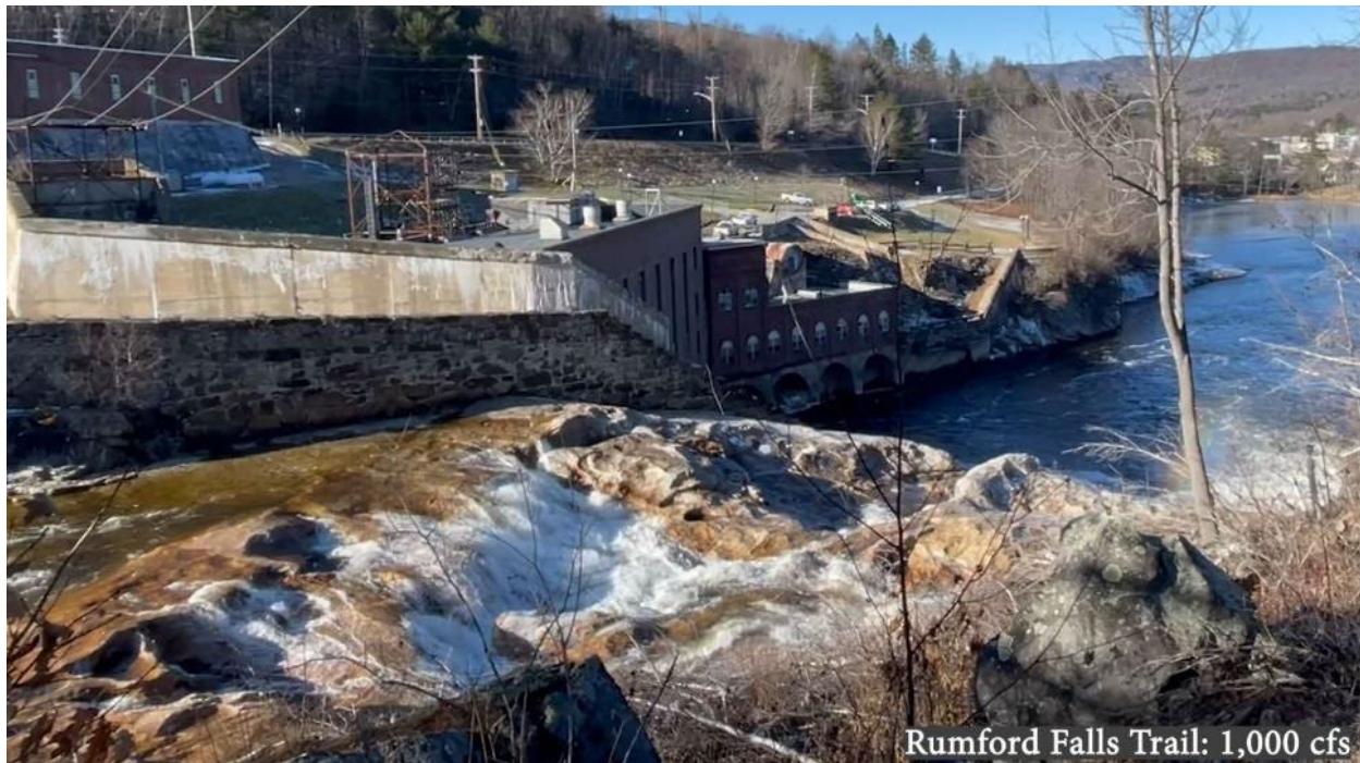
Figure 6. Upper bypassed reach with approximately 1,000 cfs of flow (source: Updated Study Report filed 8/5/22).
