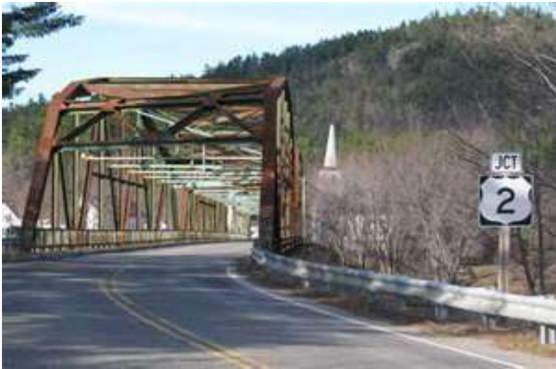
Martin Memorial Bridge
