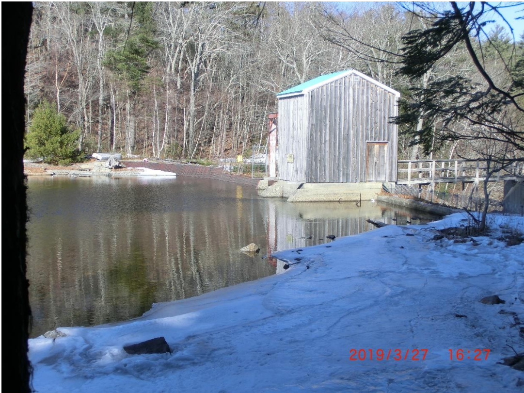
Photo 2-2 Green Lake Dam from the Southeast
