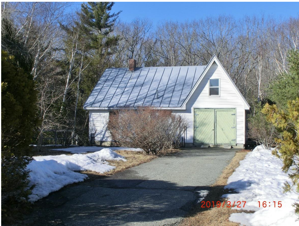
Photo 2-7 Powerhouse from Driveway
