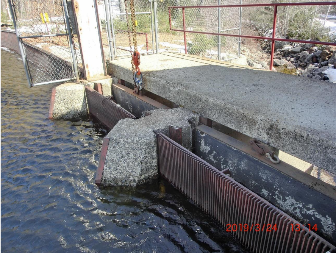
Photo 2-4 Green Lake Dam Gates and Fish Screens
