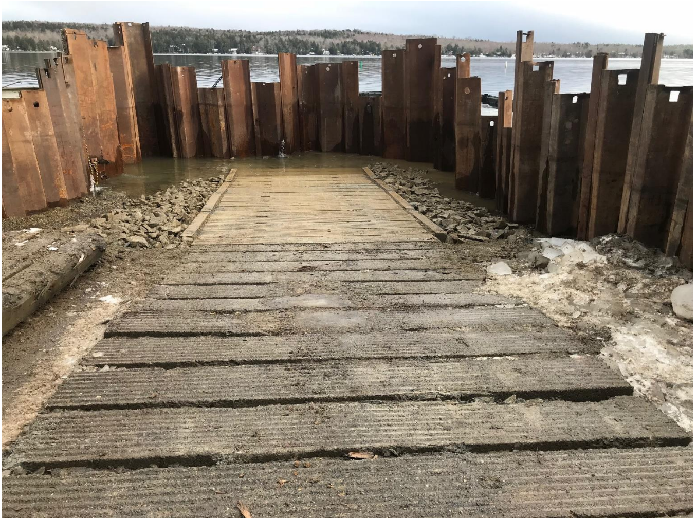
Photo 6-1 The boat ramp with extension – November 2018
