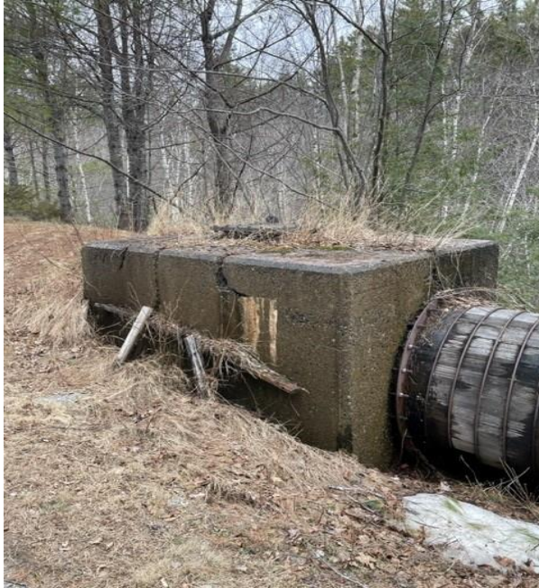
Figure 1. Penstock concrete transition block, Green Lake Hydro Power Company (P-7189), April 11, 2023.
